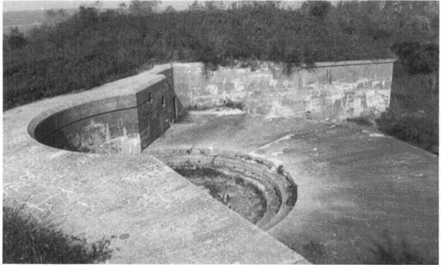
*Gun Battery, Fort Wetherill, c. 1902, Fort Wetherill Road. The inner part of this fort, now state-owned and part of a park system, shows a circular gun platform at the right, and the openings inside the concrete works.*
