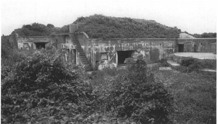
*Fort Wetherill, Submarine Mine and Cable Facility, 1908, 1940, Fort Wetherill Road. The eastern end of the Fort Wetherill site, at the cove, was used to store underwater cables that were strung here across a narrow part of the East Passage to the Newport shore. The three end-gable buildings are the earliest, built between 1908 and 1911. Above them is the site of old Fort Dumpling. The long, one-story building at the right is a submarine mine warehouse built in 1940.*
