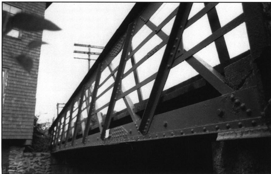
The bridge's trusses could also be considered lattice girders. The use of large lattice girders as major structural members enjoyed only a brief popularity before other types of trusses and beams became standard in bridge building.
