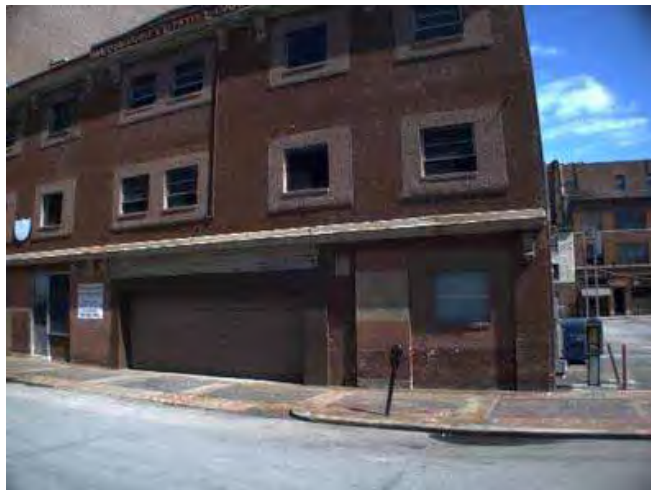
View northerly of the garage showing 1970s alterations, 2011.
