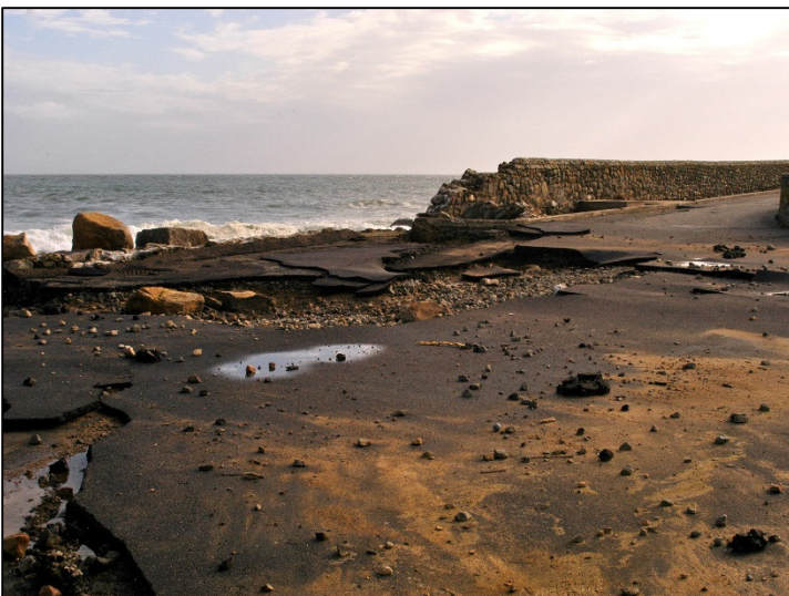
Above: Seawall at Watch Hill Lighthouse, Westerly
