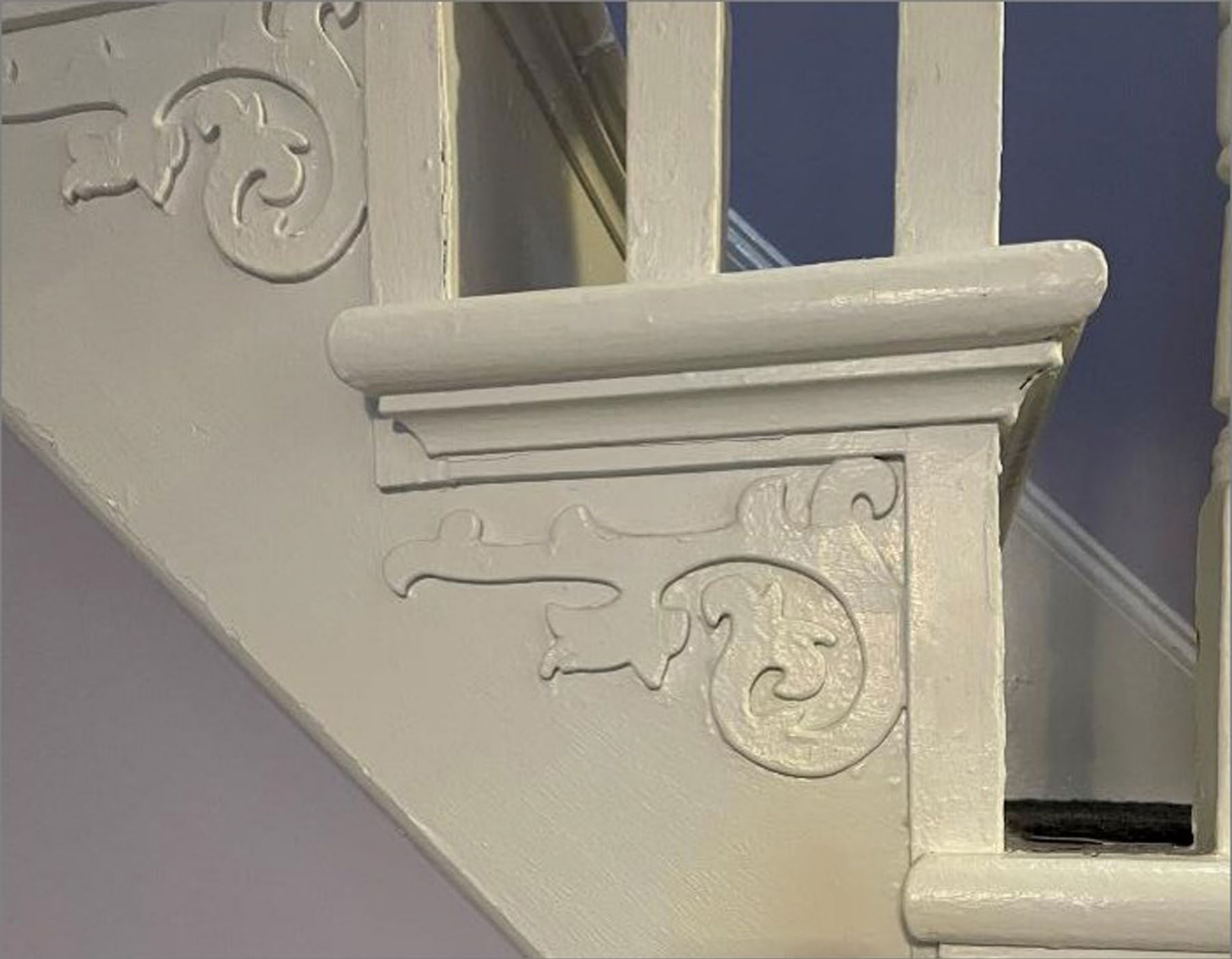
Photo 14: Detail of stringer ornamentation at first floor.
