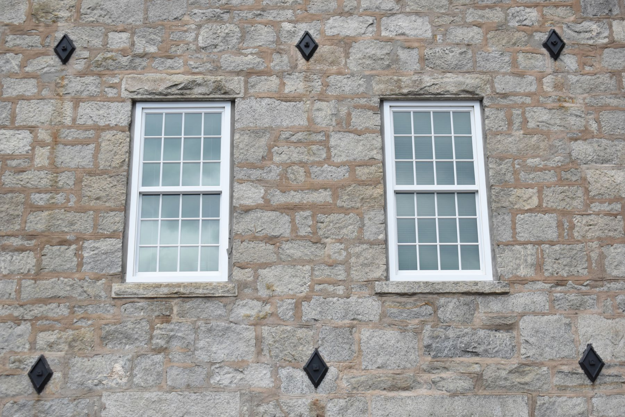
Photo #10: Detail of Arctic Mill exterior stonework and anchor plates, looking north
