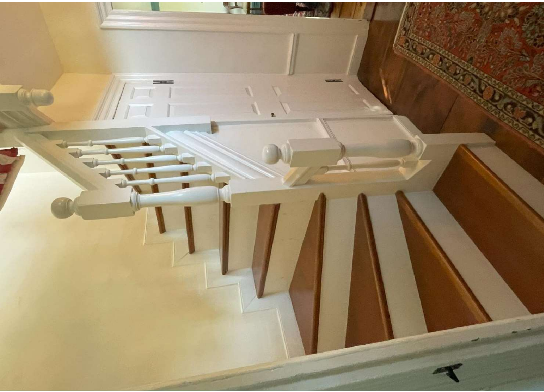
Photo 16: Interior, main block, first floor, entrance vestibule and front stair hall, looking northeast. Shows the front stairway with original Georgian-style railings, newel posts and drop pendant. The closet under the stairs provides access to the smoke chamber in chimney.
