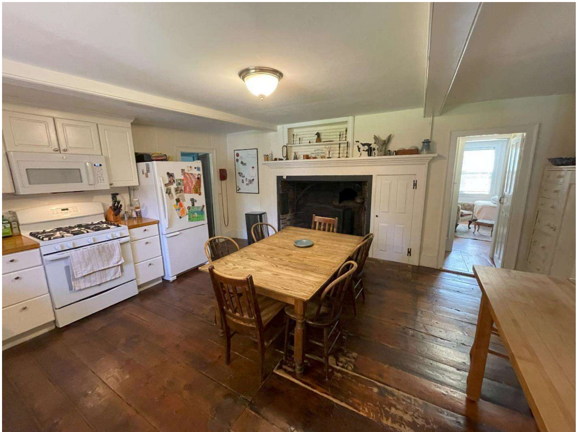
Photo 23: Interior, main block, first floor, kitchen, looking southeast. Both exposed chimney girts with beaded-edge casings are visible.
