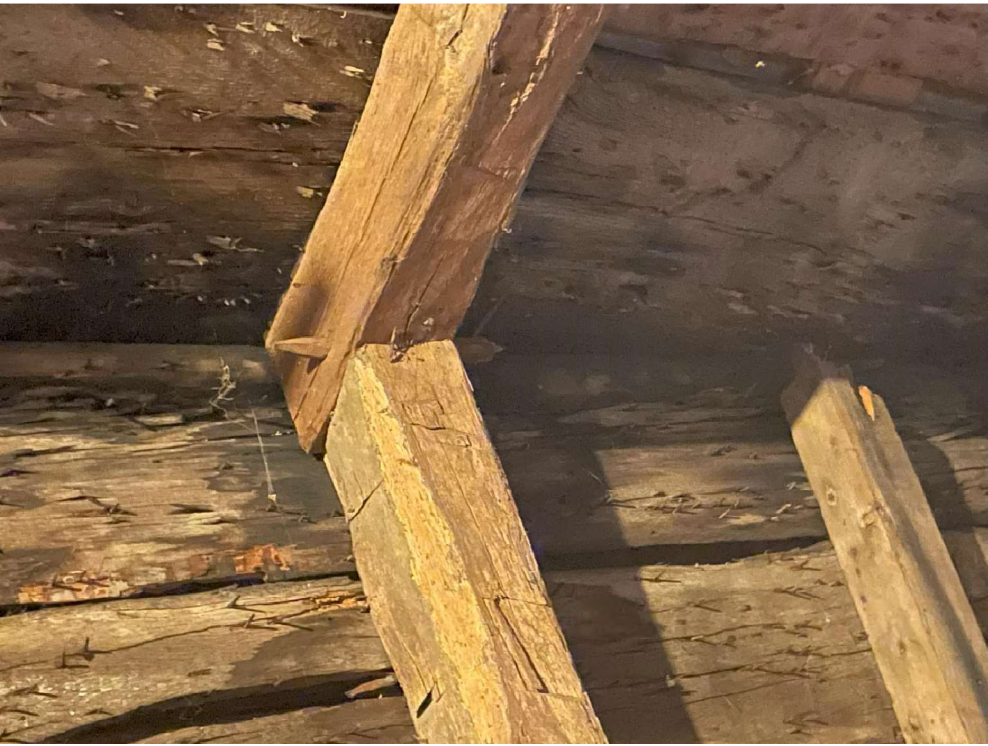
Photo 47: Interior, main block, attic, detail of pegged rafters.
