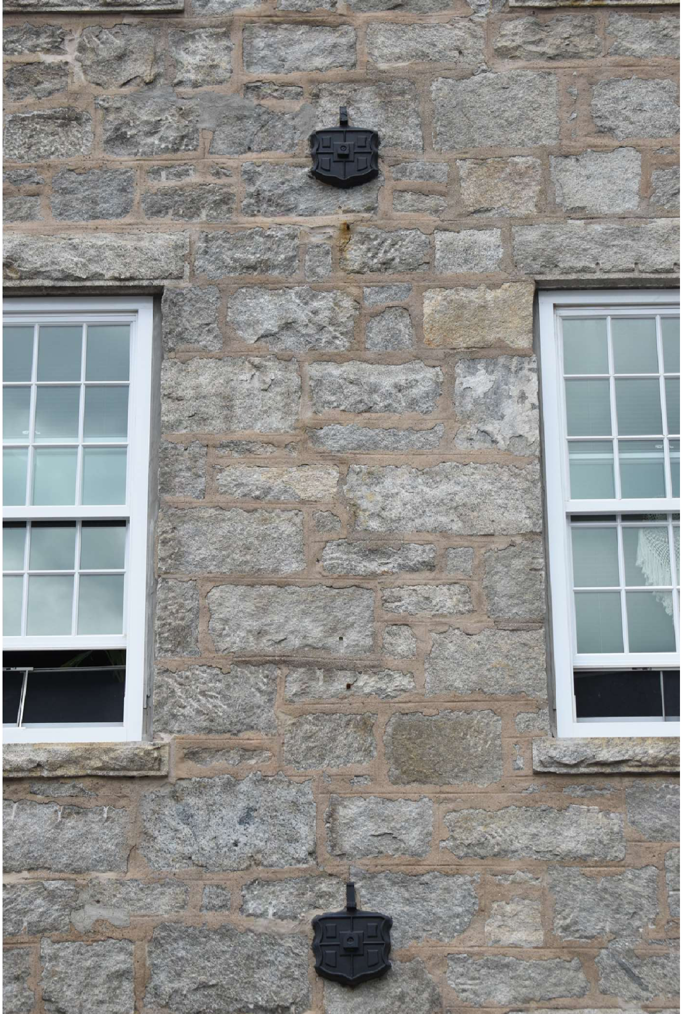
Photo #11: Detail of Arctic Mill exterior stonework and anchor plates, looking west
