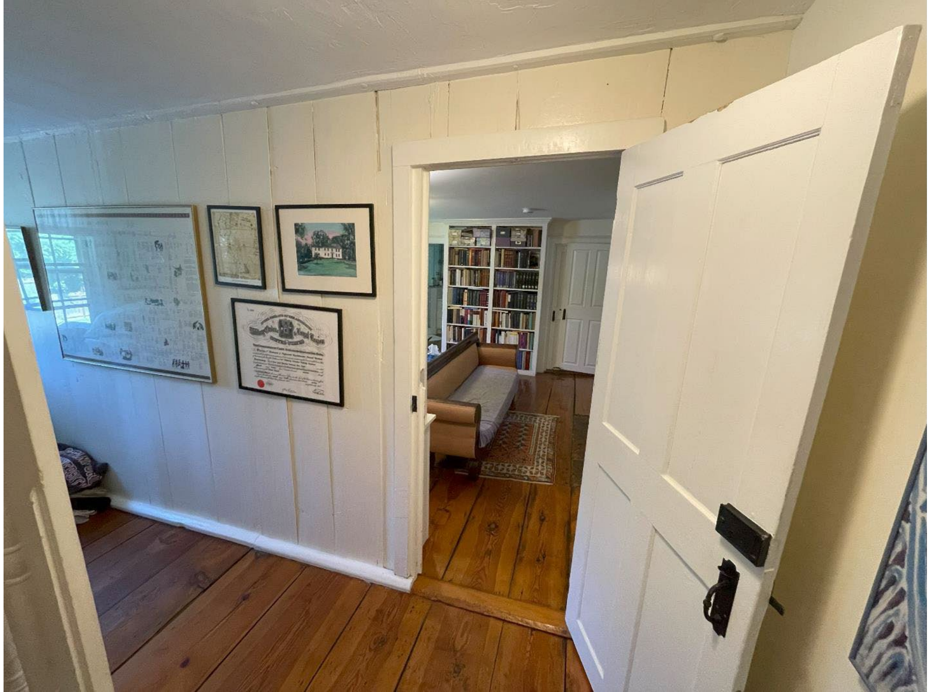
Photo 42: Main block, second floor, back stair hall, looking northeast at partition wall installed ca. 1802 when the house was converted to 2-family use.
