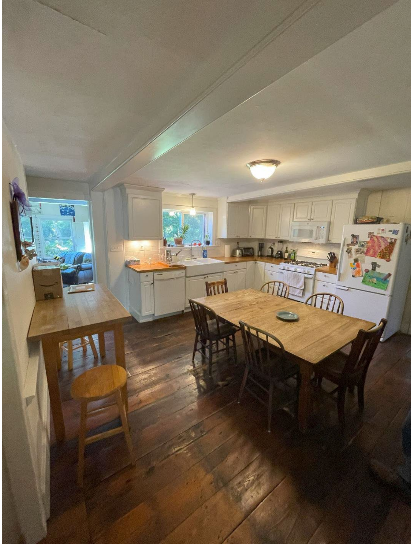
Photo 22: Main block, first floor, kitchen, looking northeast. The ceiling beam with beaded-edge casing in the foreground is the west chimney girt; part of the east chimney girt is also visible.
