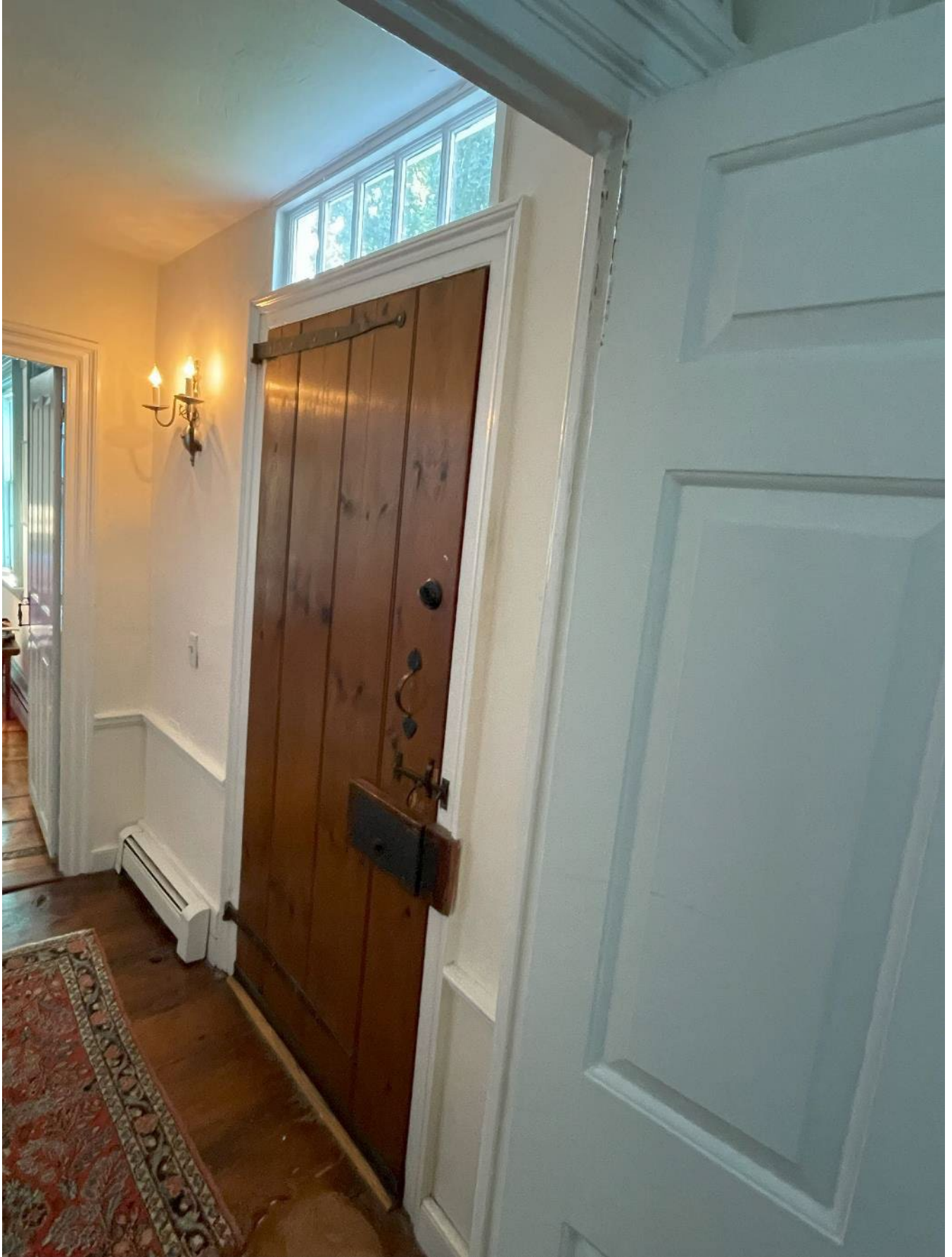
Photo 15: Main block, first floor, entrance vestibule and front stair hall, looking southeast. Shows the interior face of the front door with ca. 1951 “colonial” vertical board panels and reproduction wrought iron strap hinges, and an 18 th century rim lock.
