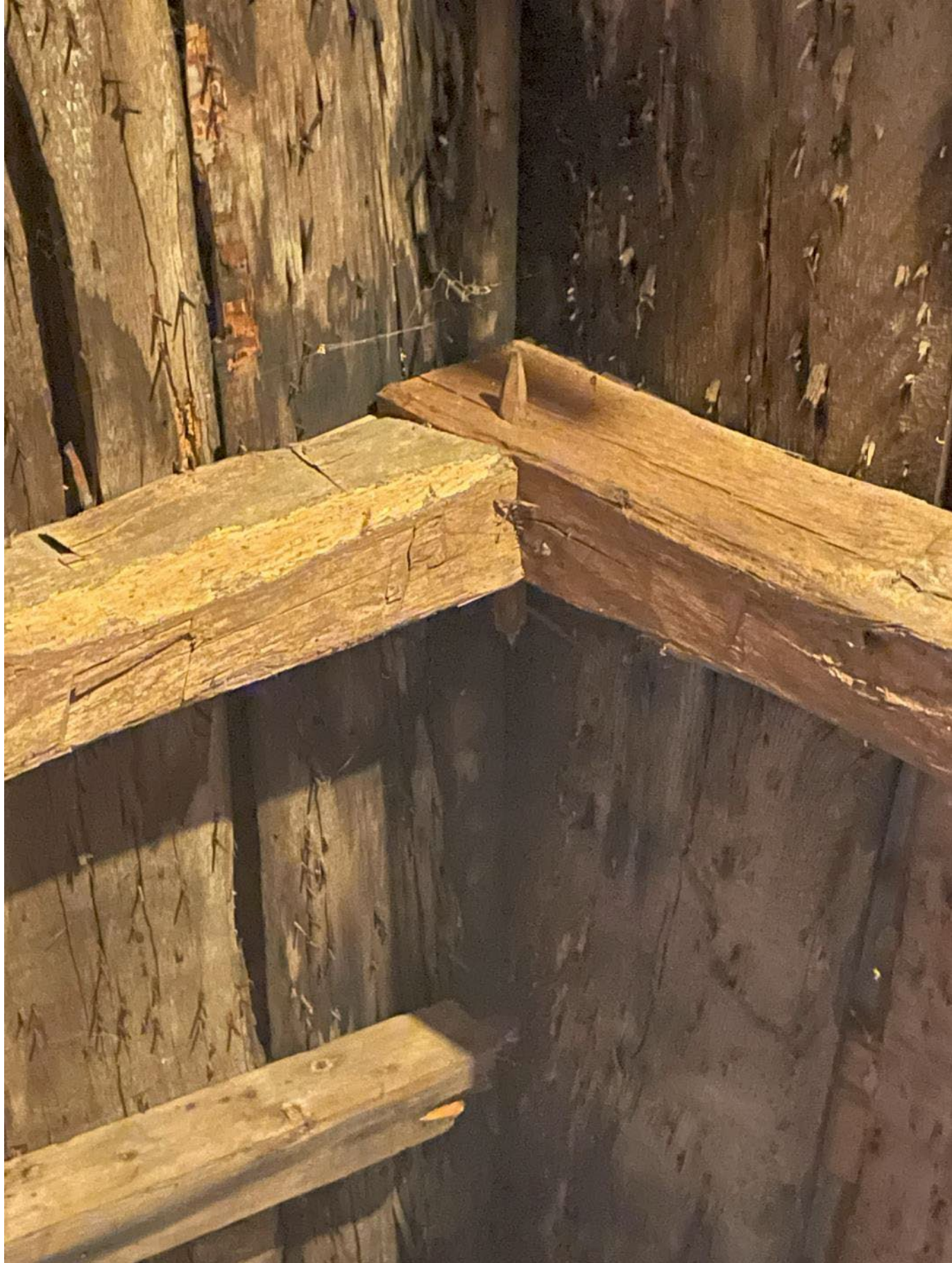
Photo 47: Main block, attic, detail of pegged rafters.
