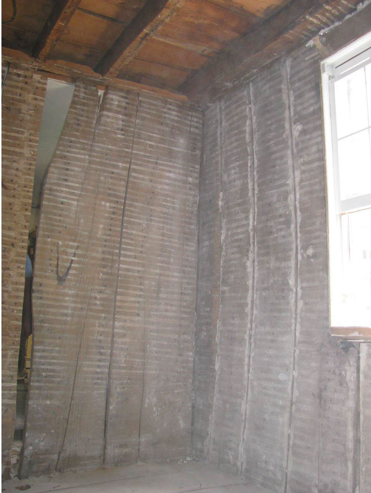
Photo 27: Main block, first floor, northwest corner room before 2010 removal of partition wall, looking southwest. The oak vertical planks of the partition wall that ran east-west (shown at left) match the oak vertical planks of the west exterior wall (shown at right), indicating that the partition wall was likely original.
