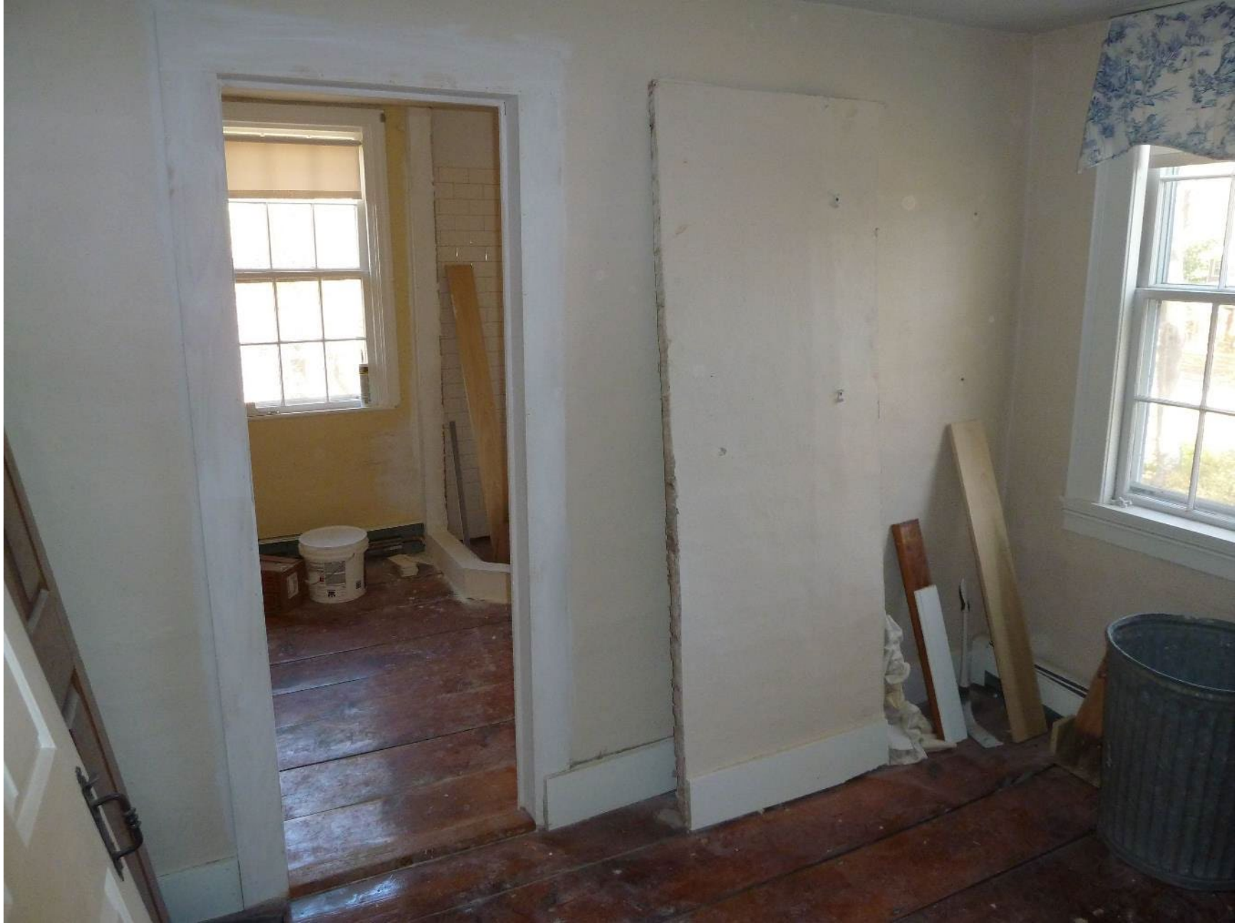
Photo 38: Main block, second floor, northeast corner rooms, looking northeast. Shows the original partition wall running east-west with a doorway cut out in 2010 to connect the present master closet (seen in foreground) with the master bathroom beyond; see Photo 39 for a detail view of the cut-out section.
