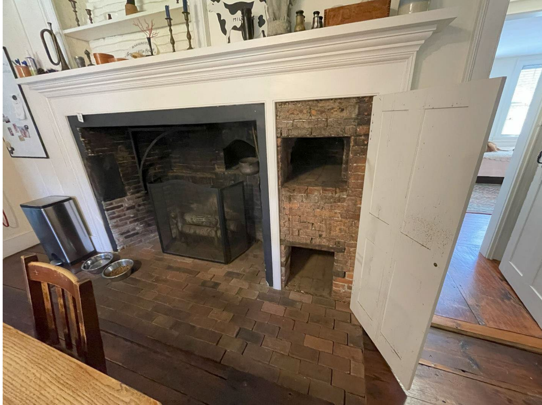
Photo 24: Main block, first floor, kitchen, looking southeast. Close-up view of the fireplace with two beehive ovens, firewood storage, and whetstone (on the left wall of the firebox).
