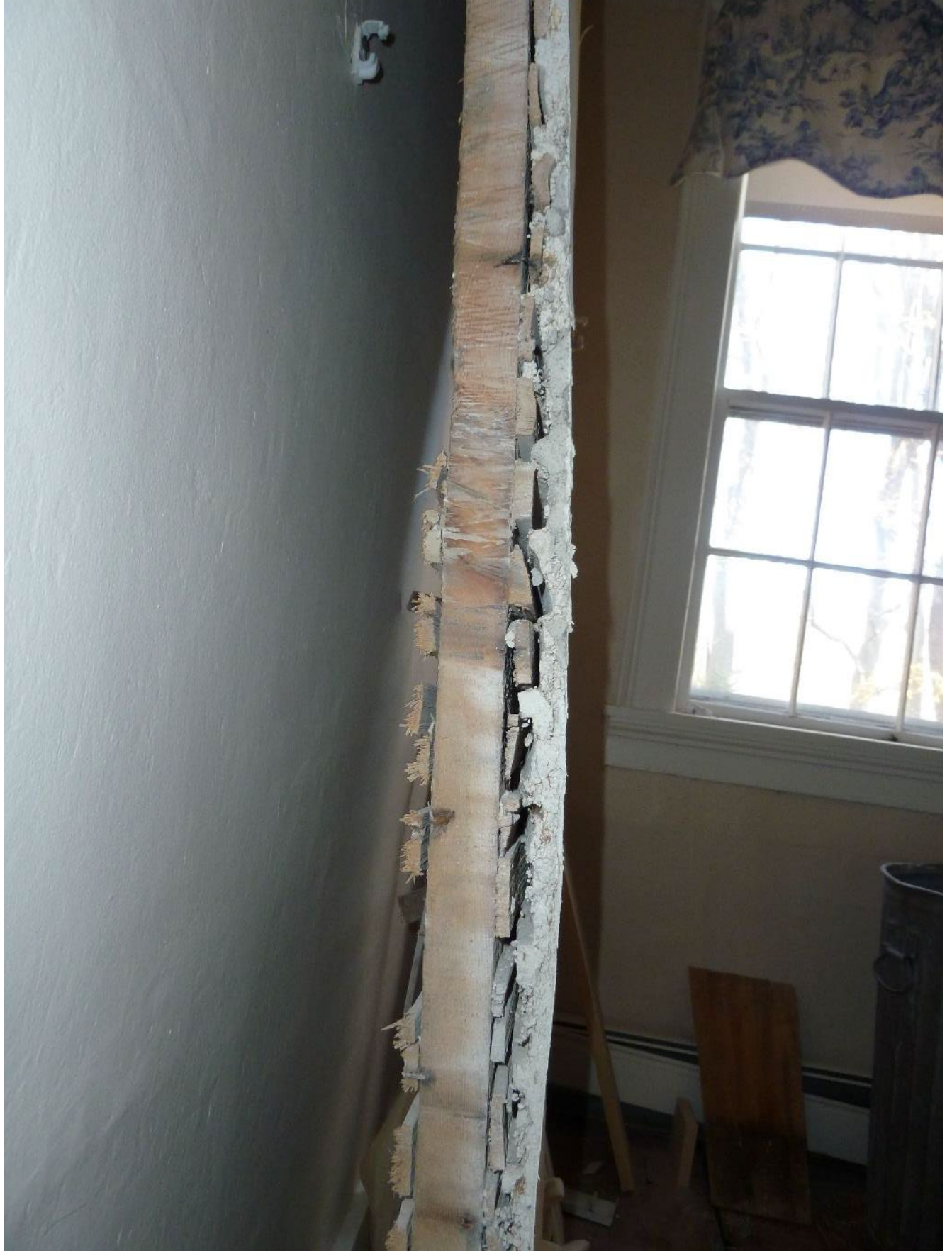
Photo 39: Main block, second floor, northeast corner rooms, detail of partition wall running east west that was cut out in 2010 to create a doorway; see Photo 38. Shows the original vertical plank wall structure of the partition wall, with applied lath and plaster.
