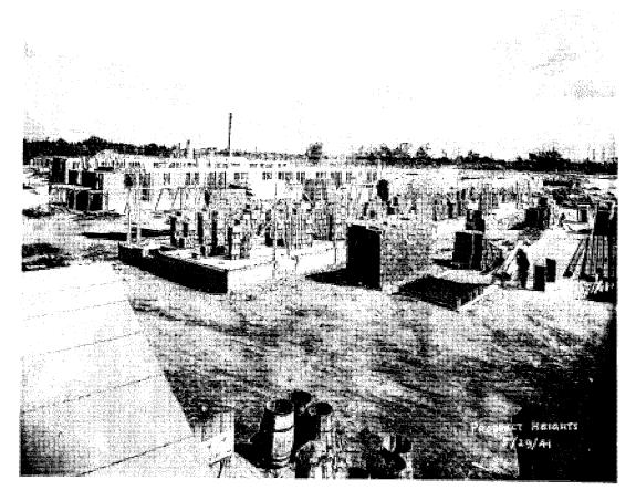
Figure 12 Row house concrete foundations ready for brickwork (May 1941)
