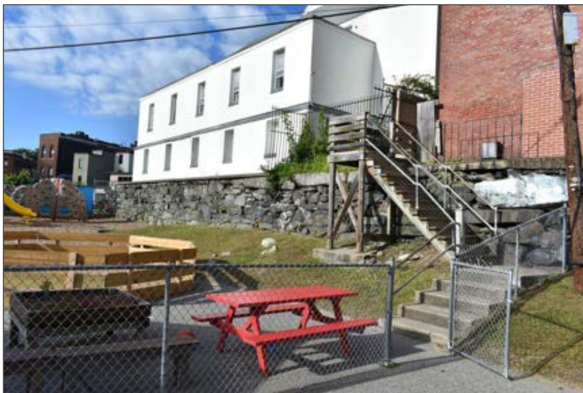
19. Detail of the historic stone retaining wall looking east.
