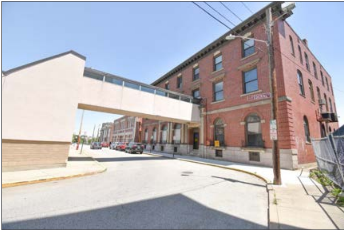
9. Streetscape of Federal Street looking east near dogleg turn with the YMCA in foreground.
