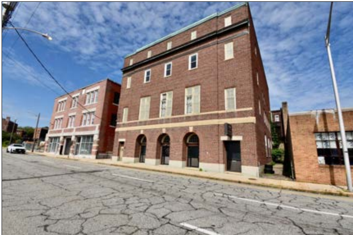
2. View looking southwest towards Masonic Temple (foreground) and Joseph Grenon's Garage (left).
