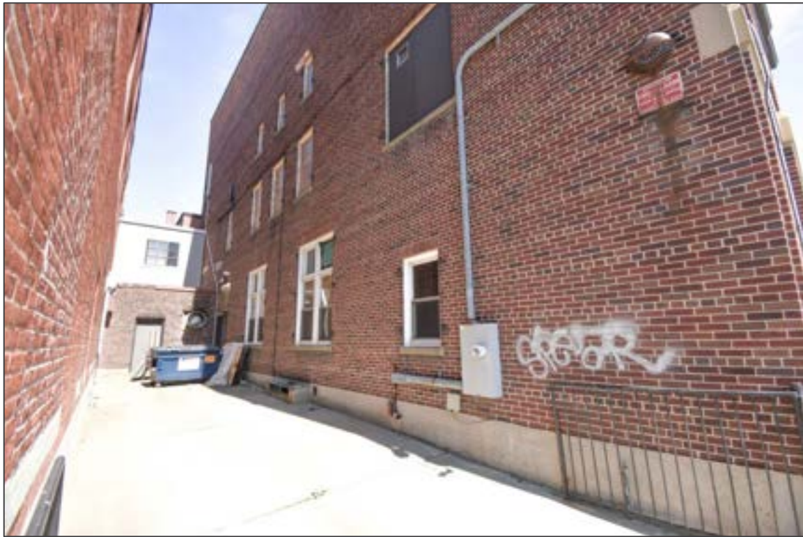
3. View looking north towards Joseph Grenon's Garage (far left), Masonic Temple ell and CYO passageway (near left), and Masonic Temple (right).
