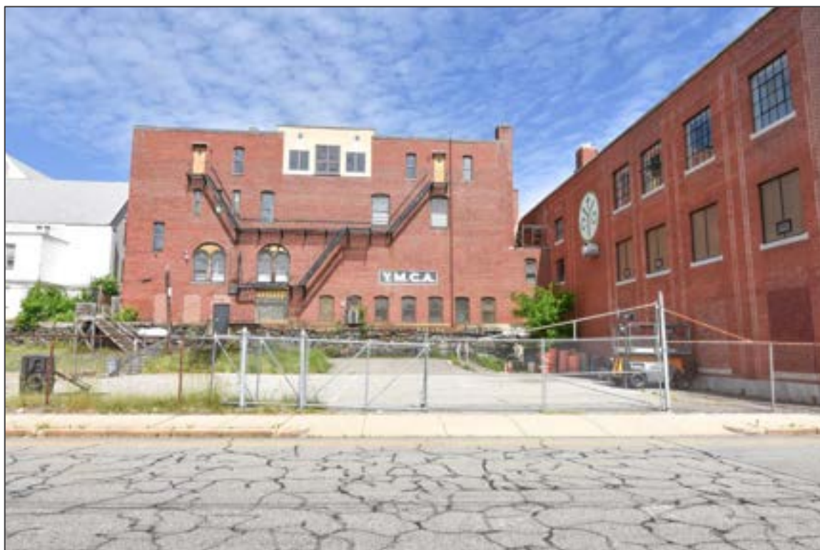
11. View looking northwest towards the YMCA, First Methodist Episcopal Church (left), and Joseph Grenon's Garage (right).
