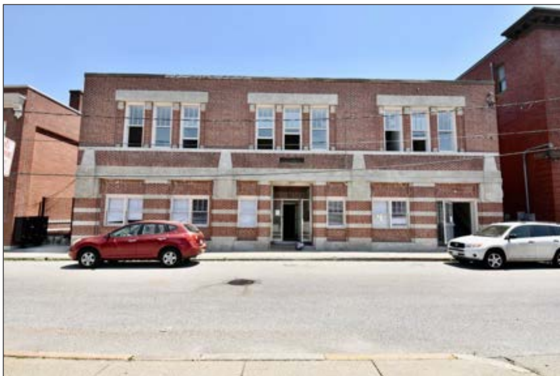
13. View looking southeast towards Joseph Grenon's Garage.
