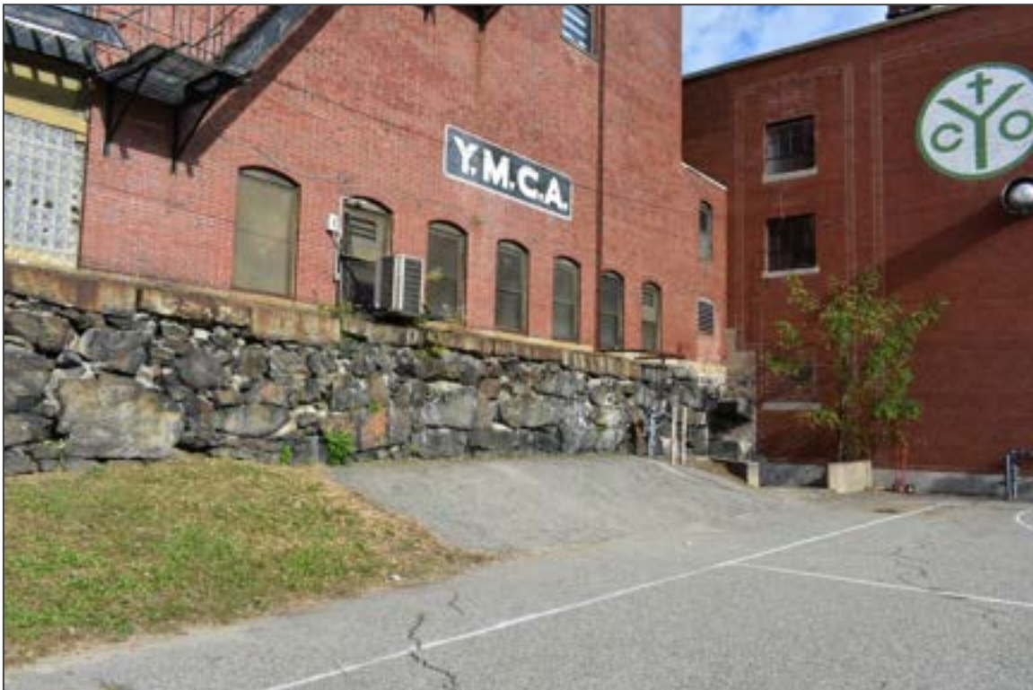
18. Detail of the historic stone retaining wall looking north.
