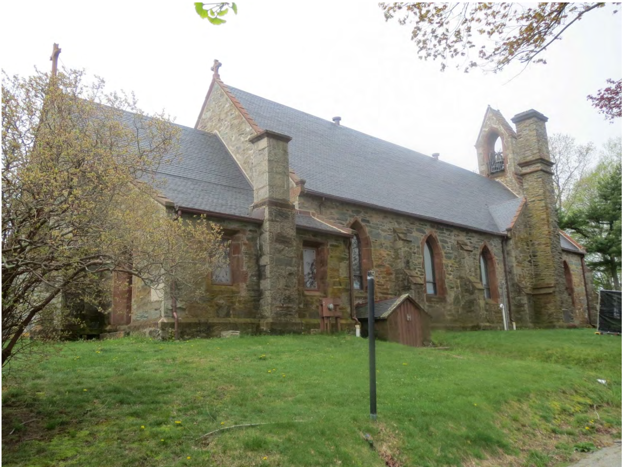
Photo #3: St. Mary's Church, east and north elevations, looking southwest.
