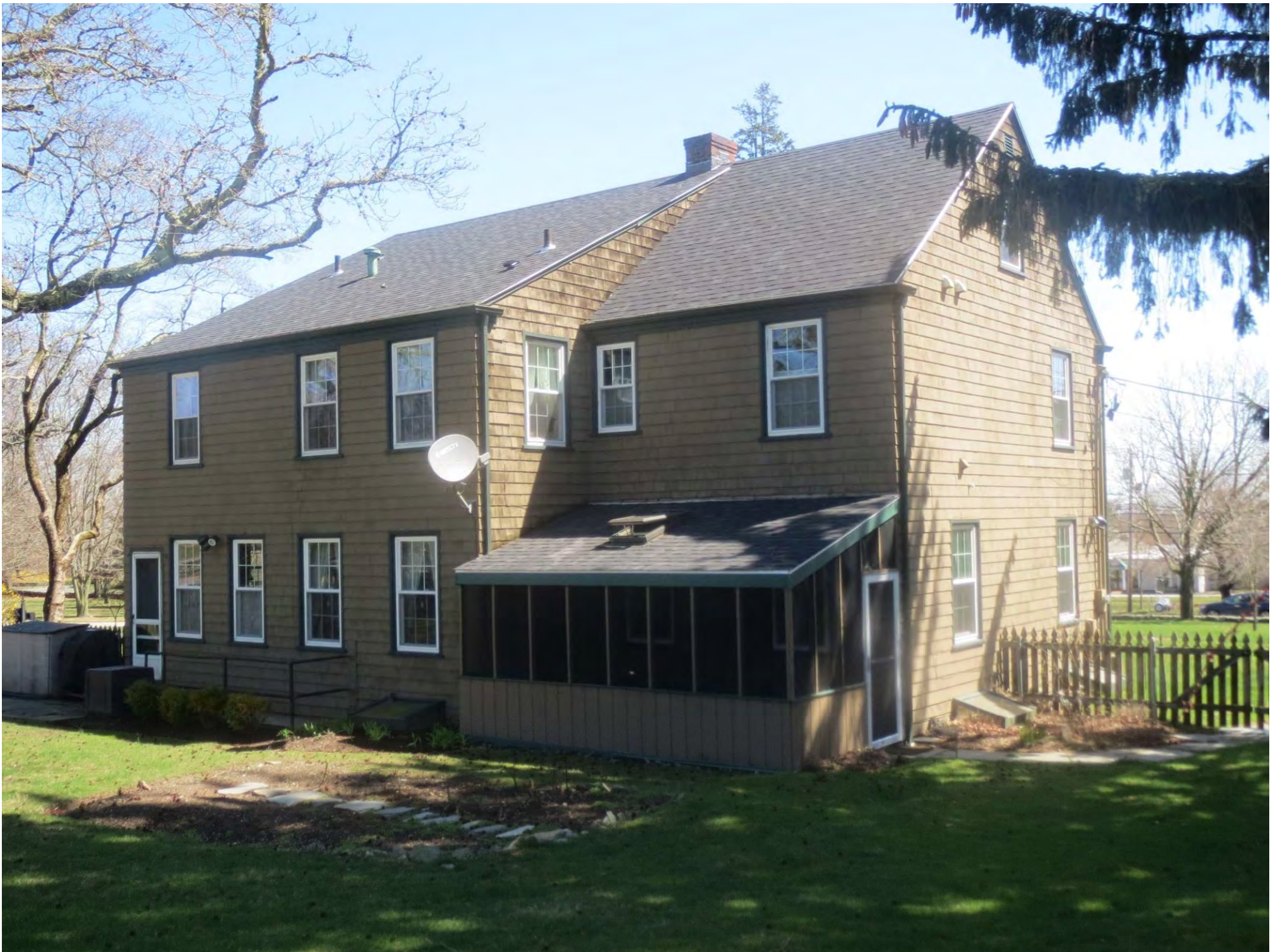
Photo #17: St. Mary's Rectory, west (rear) and south elevations, looking northeast.
