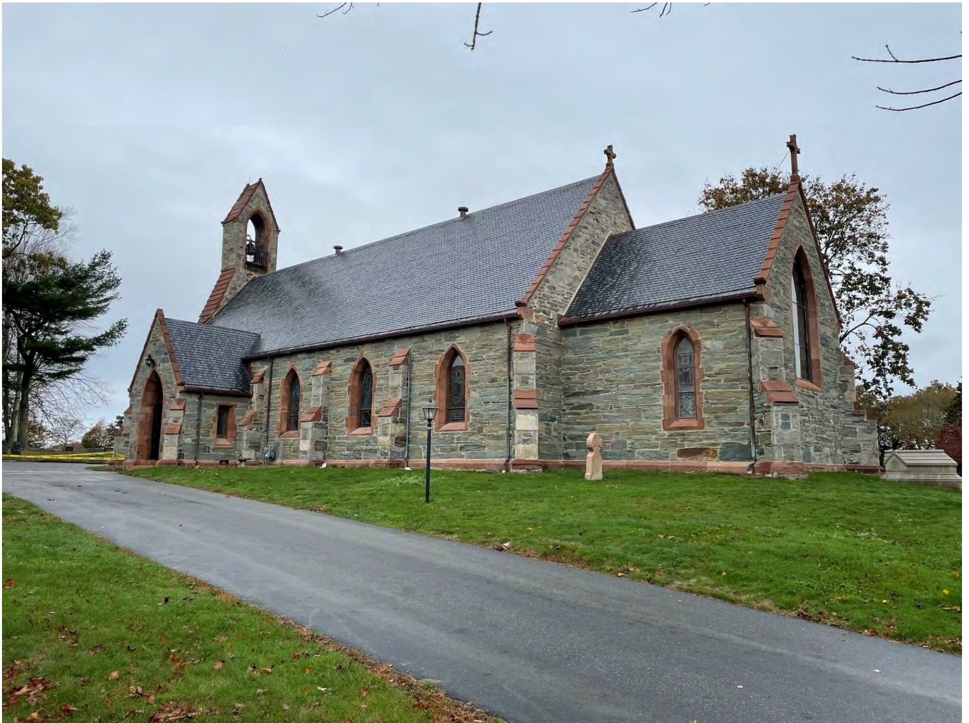
Photo #2: St. Mary's Church, south and east elevations, looking northwest. Note the two funerary monuments: one for St. Mary's founder and benefactor Sarah Gibbs, stands at far right in photo; (see also Photo 26); the other for St. Mary's first and longest-serving Rector, Rev. Hobart Williams and his wife Augusta, stands in mid-foreground.
