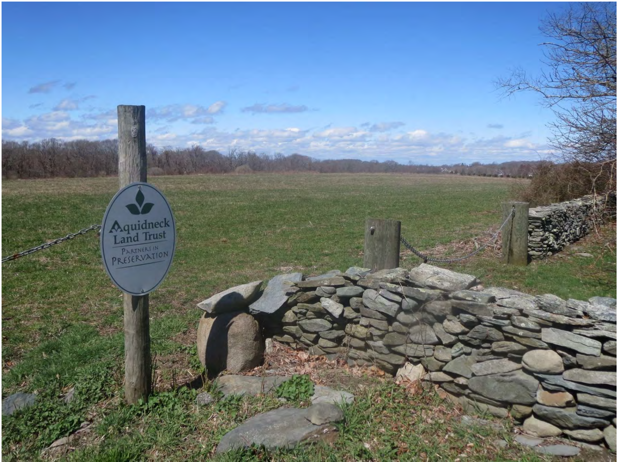
Photo #30: St. Mary's property, looking northwest beyond the historic stone wall that marks the western boundary of that part of the property where all buildings and the cemetery are located.
