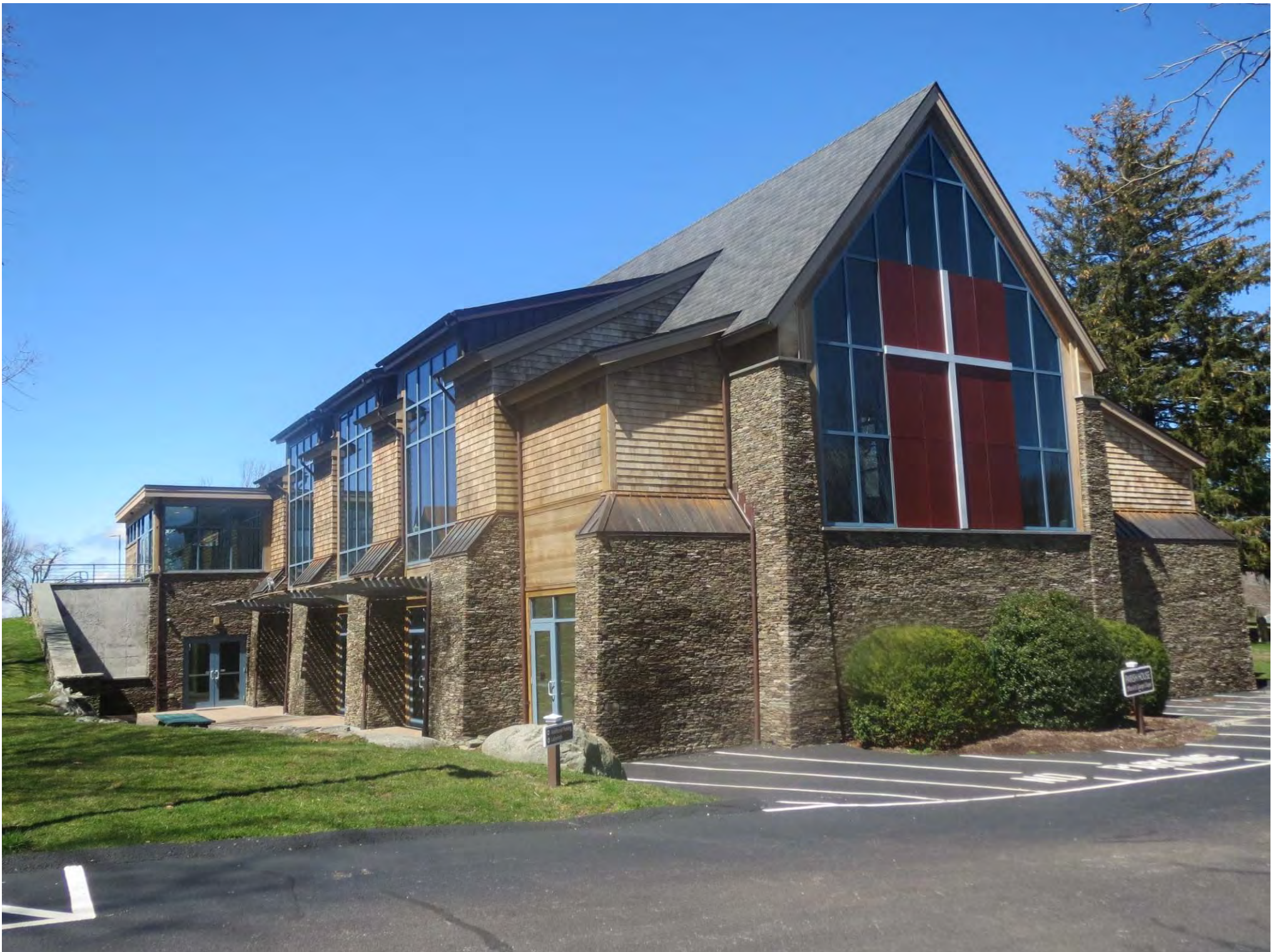
Photo #22: Parish House, east and south elevations, looking northwest.
