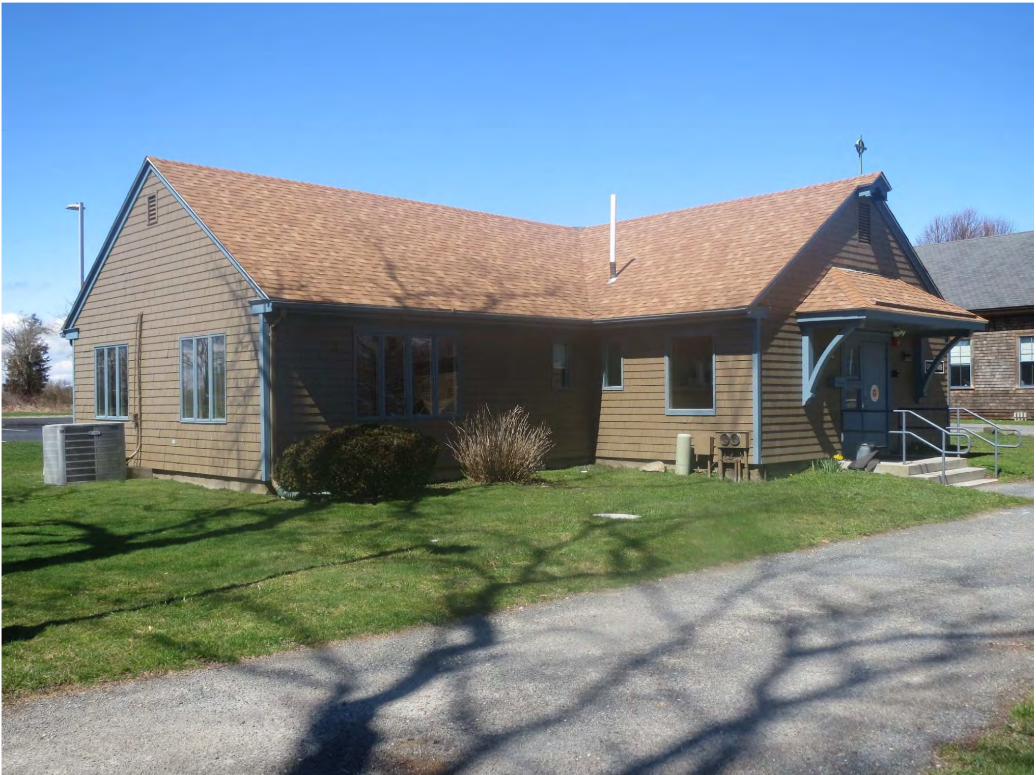
Photo #21: Gibbs House, east façade and south elevation, looking northwest.
