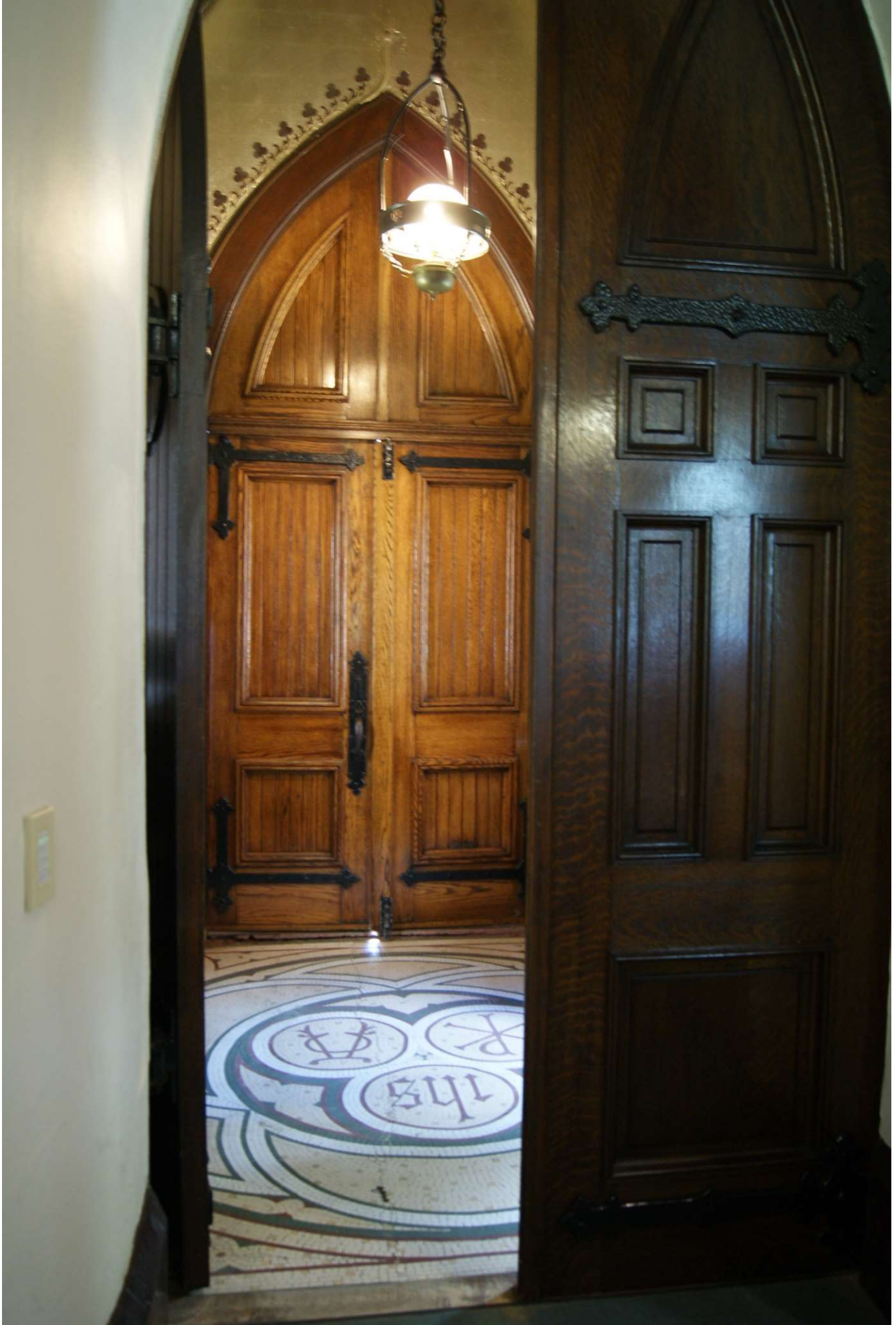
Photo #14: St. Mary's Church, interior, vestibule, looking south from the nave; exterior doors and mosaic tile flooring installed 1908.
