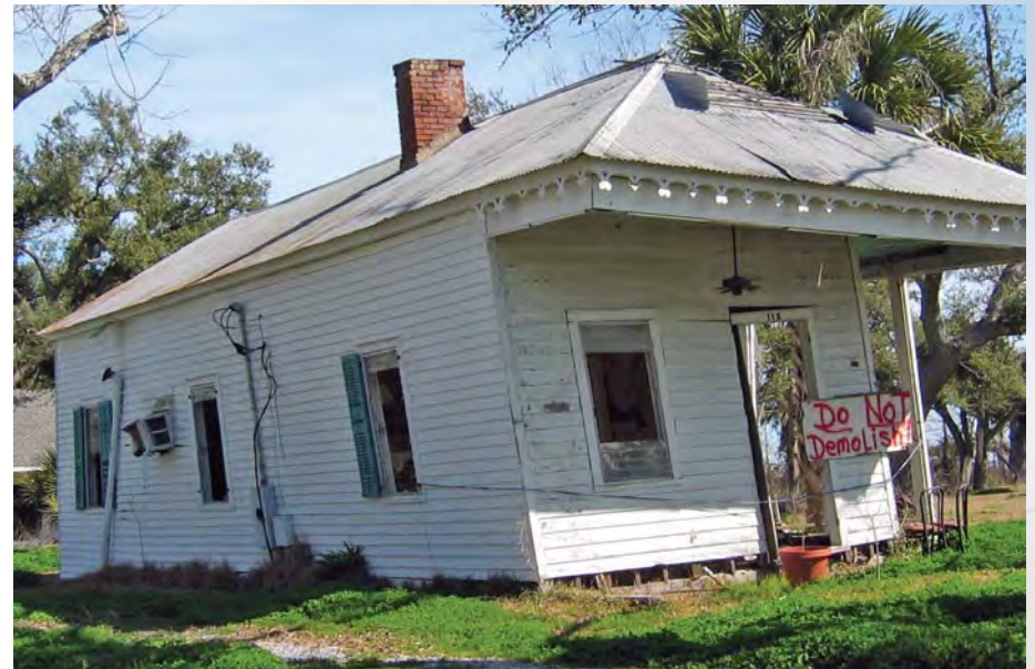
The MDA Grant Program can help historic property owners reduce their risk from future floods.
