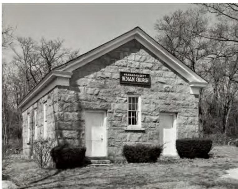
Figure 8: Narragansett Indian Church (1859), listed in the National Register in 1973 as a contributing resource to the Historic Village of the Narragansetts in Charlestown Historic District, Charlestown, RI. [Image credit: John M. Miller, via Society of Architectural Historians “Archipedia.”]
