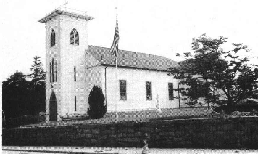
St. Mary's Roman Catholic Church (1844-45); Church Street, Crompton
