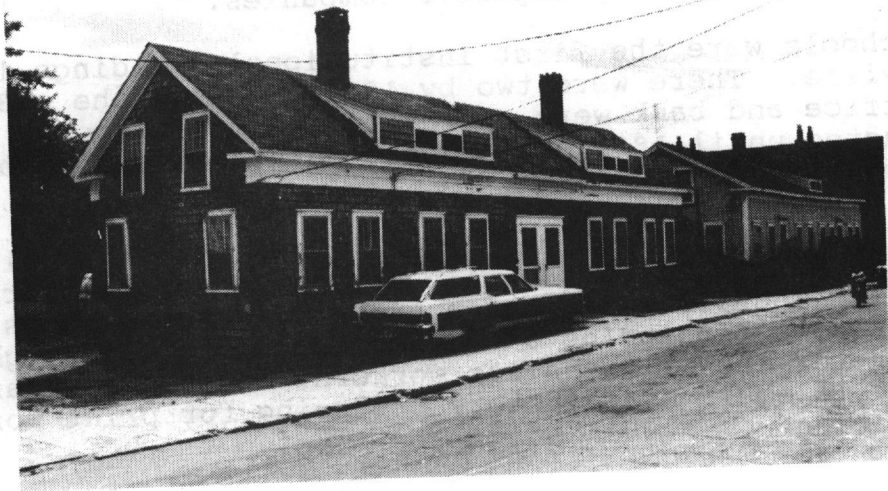
Mill Houses (early 19th century); 6-8 and 10-12 Remington Street, Crompton
