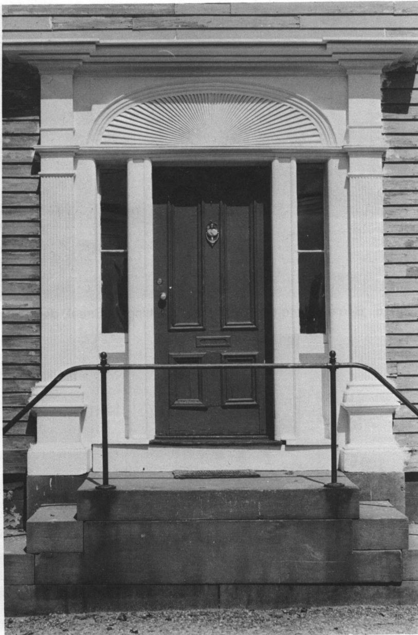
Fig. 8: Rudolphus B. Johnson House (c. 1790, c. 1823), 43 Miller Street
