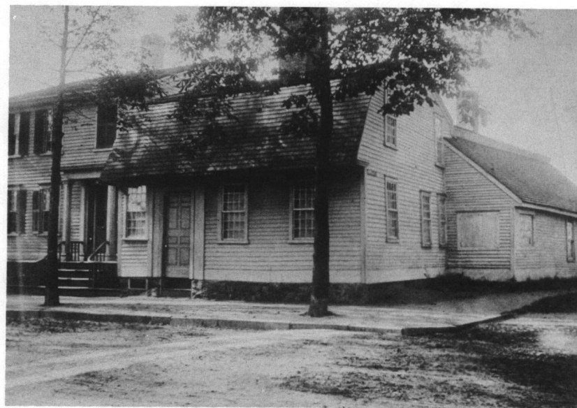
Fig. 6: Burr's Tavern (c. 1680), Main/Washington Street, demolished
