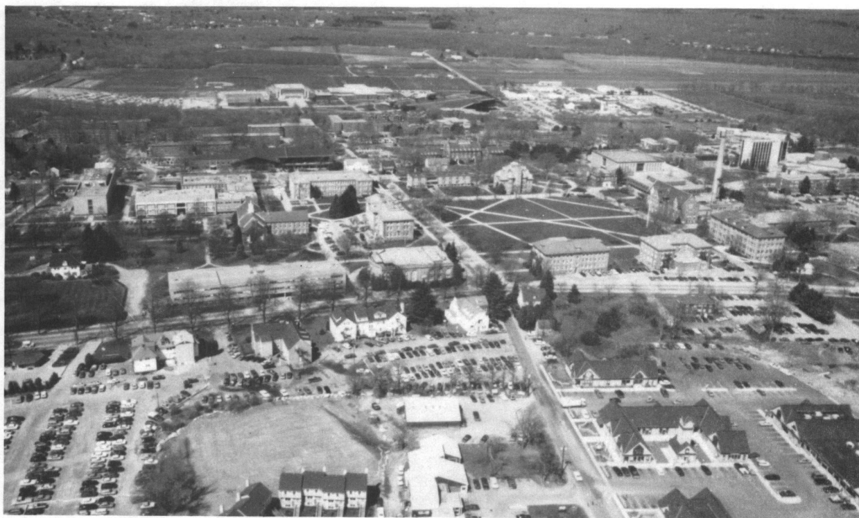
University of Rhode Island (1888 et seq.), off Kingstown Road (RI Route 138) at Upper and Lower College Roads, Kingston village, South Kingstown. View to west showing the original quadrangle and fields on the right. Photograph courtesy of the R. I. Department of Economic Development.
