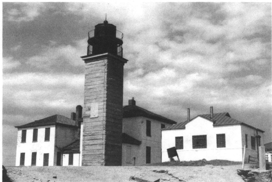
Beavertail Light Station (1856, 1898), Beavertail Road, Jamestown. View northwest with (left to right) assistant keeper's house, lighthouse, keeper's house, and old signal house.
