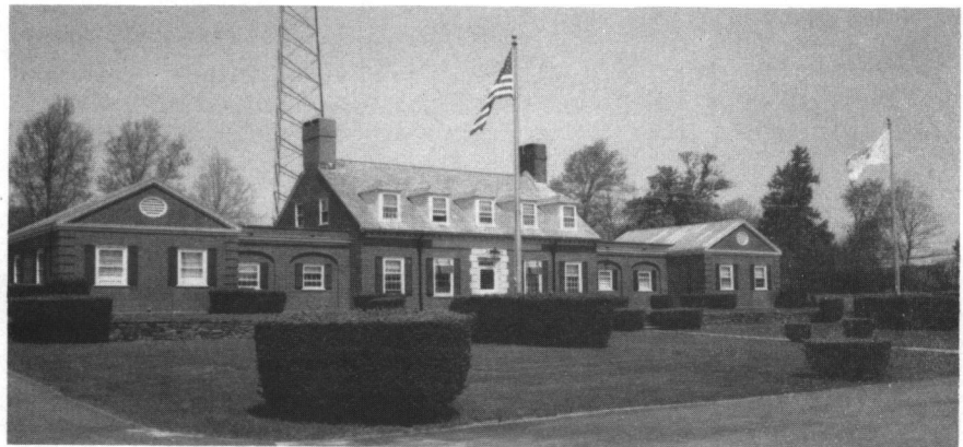
State Police Barracks (1935), East Main Road, Portsmouth.
