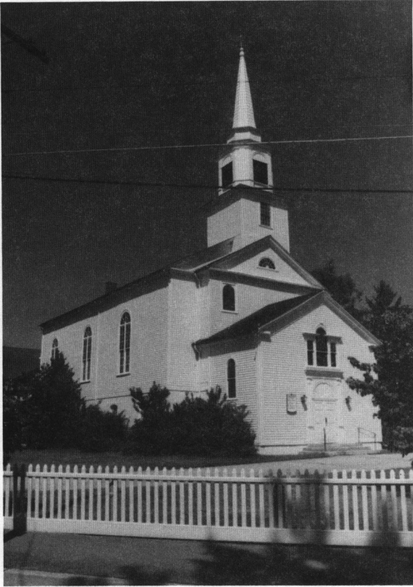
Greenville Baptist Church, 1820, 582 Putnam Pike. This typical New England meetinghouse following the models of Wren and Gibbs was built by Clark Sayles. The present high brick basement and deep front pavilion were added in 1866.
