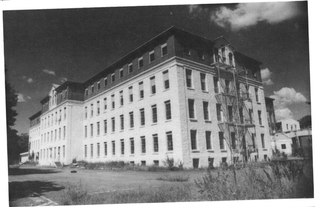
Georgiaville Mill/The Homestead Mill, 1853 et seq., Higgins Avenue. This large, Greek Revival-Italianate, stuccoed factory, was built by Zachariah Allen in 1853 as a successor to several earlier mills here. Textile manufacturing was carried on until the 1930s. In the late 1980s it was sold and converted into a condominium/townhouse complex and renamed the Homestead Mill.
