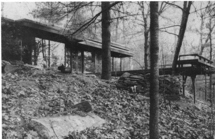
Baker House, 1962, hidden from view, at 40 Walter Carey Road. Designed by Rhode Island architect Lloyd A. Baker, this frame house, built with redwood, has a flat roof with a wide overhang and a clerestory.
