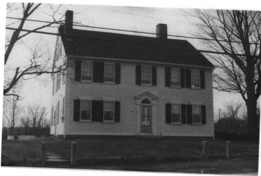
Angell's Hotel, c. 1810, 620 Douglas Pike. This structure was probably used as a hotel when the Douglas turnpike was constructed in 1809. It has a pedimented entry with a leaded fanlight.
