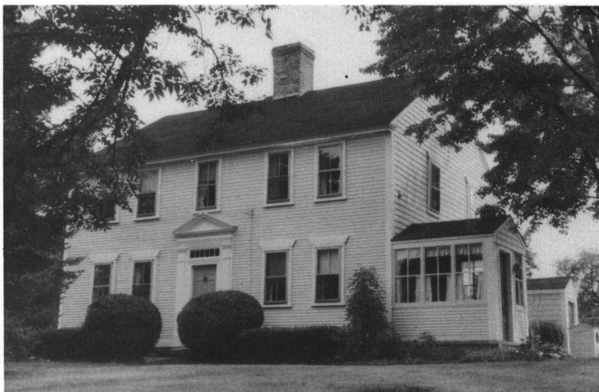
Farmhouse, late 18th century, 211 Harris Road. A large Rhode Island farmhouse. This one has a pedimented entry with transom lights.
