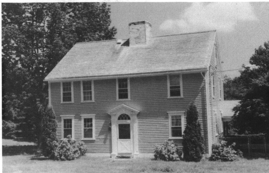
Joseph Farnum-Brown House, c. 1770, 243 Old County Road. This typical Rhode Island farmhouse has a fine pedimented entry with a semi-elliptical fanlight of a type common in early Smithfield houses.
