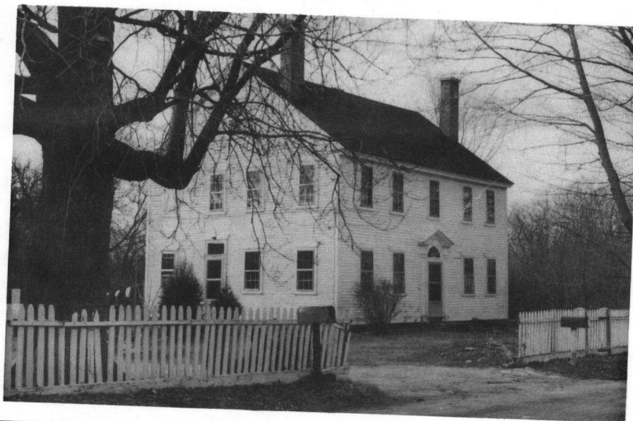
Angell-Ballou House, early 19th century, 43 Ridge Road. A fine early farmhouse with paired brick chimneys and an ornately leaded semi-circular fanlight in a pedimented entry.
