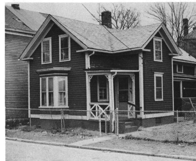
Fig. 23: Michael Noon House (1850s); 23 Calder Street.
