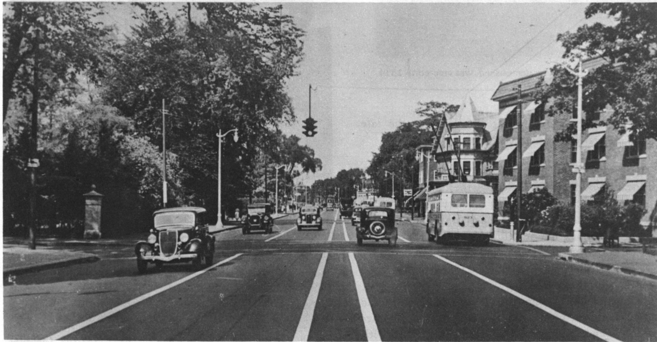
Fig. 60: Elmwood Avenue north of Daboll Street following its reconstruction in 1936; photograph, c. 1937.
