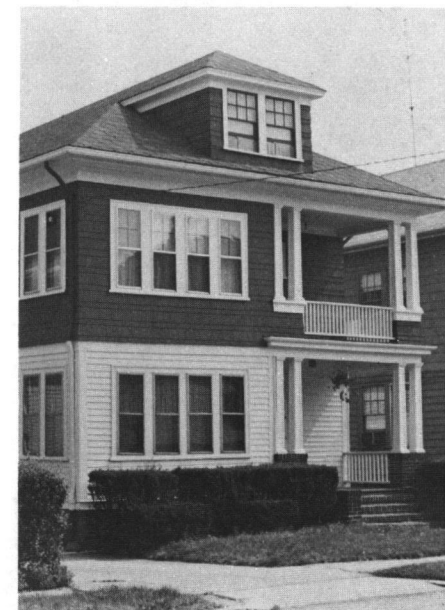
Fig. 54: Nathan Landy House (c. 1927); 90-92 Sackett Street.
