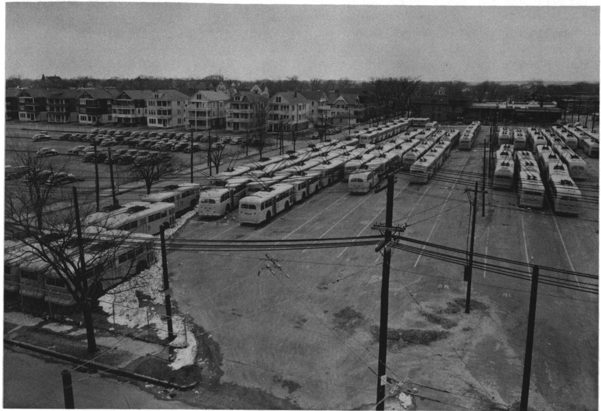
Fig. 75: The trackless-trolley storage yard at the Elmwood Garage in 1949, surrounded by early twentieth-century triple-deckers.
