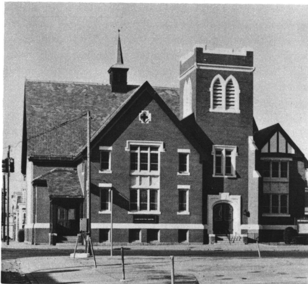
Fig. 19: Elmwood Christian Church, now First Presbyterian Church (1914-1915); 353 Elmwood Avenue.
