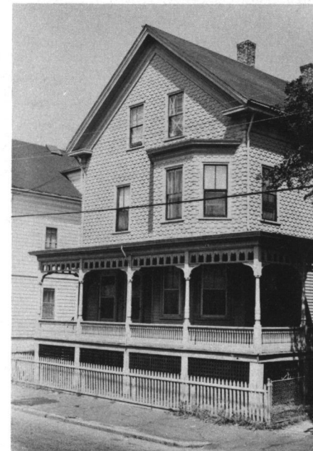
Fig. 53: Two-family House (c. 1890); 171-173 Hanover Street.
