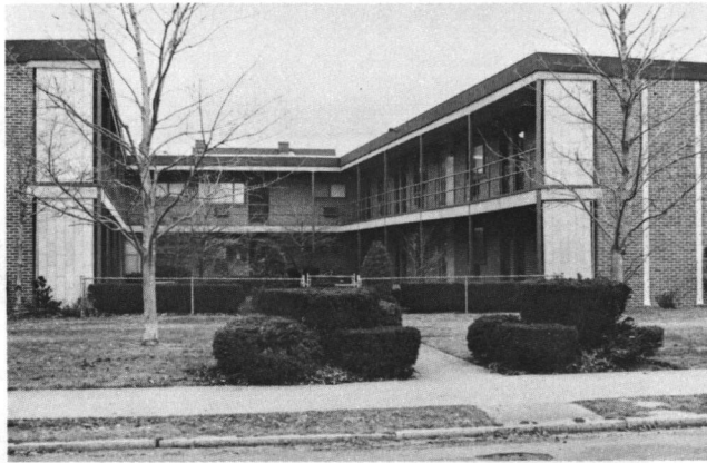
Fig. 72: Apartment House (c. 1962); 211 Adelaide Avenue.
