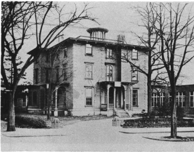
Fig. 30: Butts-Davis Mansion (c. 1860); formerly at 194 Elmwood Avenue; demolished, c. 1912.
