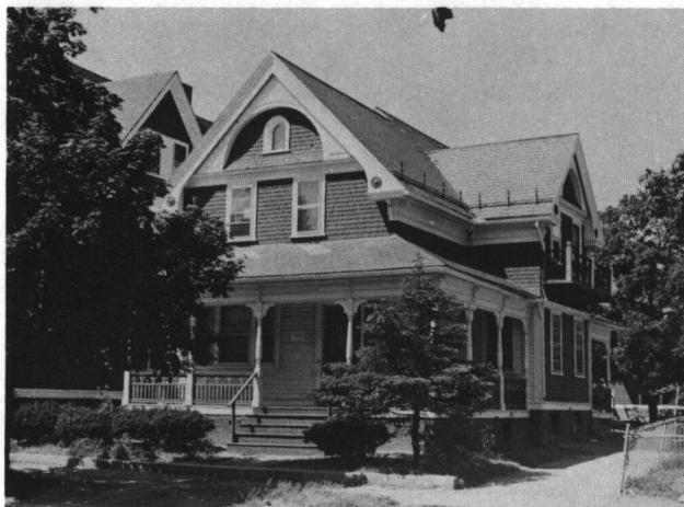
Fig. 26: Octave Bouchard House (1894); 162 Linwood Avenue.
