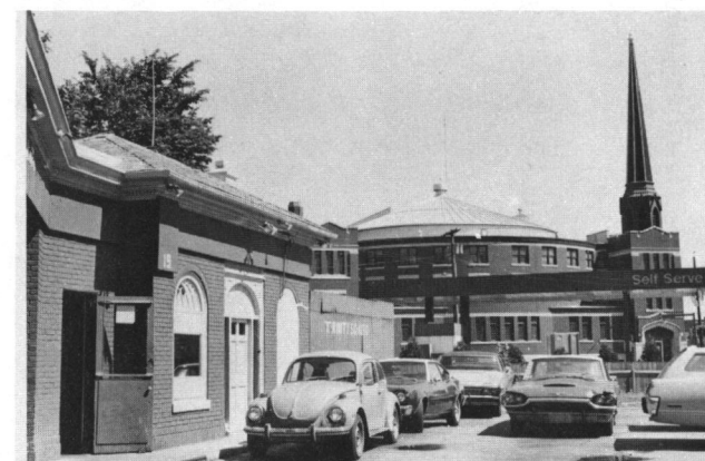
Fig. 63: Beacon Oil Company Service Station, now a used-car dealership (1930); 19 Elmwood Avenue.
