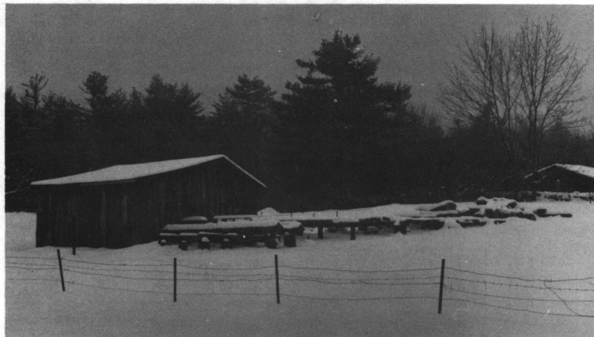
Sawmill, John Durrans Farm: Grange Road Historic District. (#3-B)
