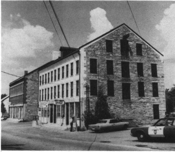
Commercial Blocks (1850 ; 1970): 7-9 and 11-13 Main Street, Slaters- ville Historic District. (#4-L)
