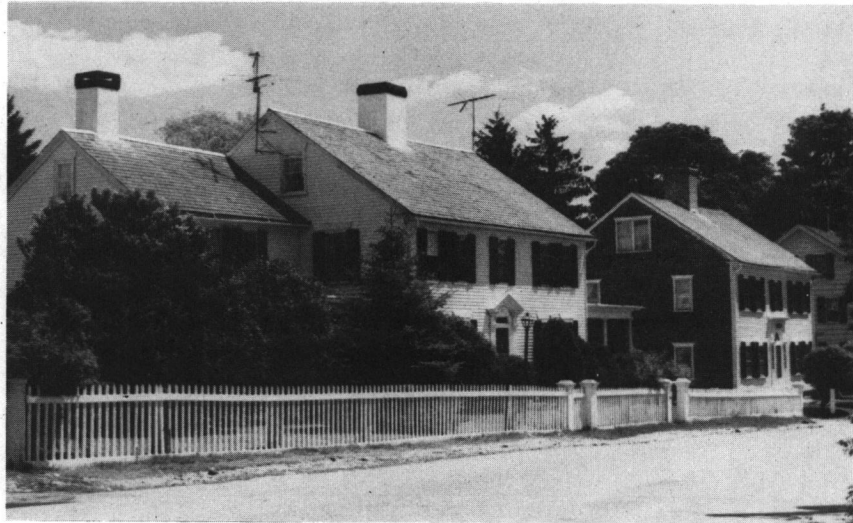
John Slater House (c. 1810): 16 School Street, Slatersville Historic District. (#4-V)
