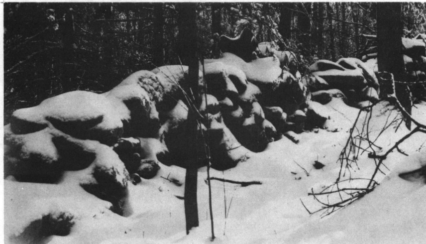
Sheep Fence: Woonsocket Reservoir Number 3 Natural and Historic Area. (#12)
