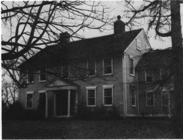
Walter Allen House (1802): 138 Great Road, Union Village Historic District. (#6-I)
