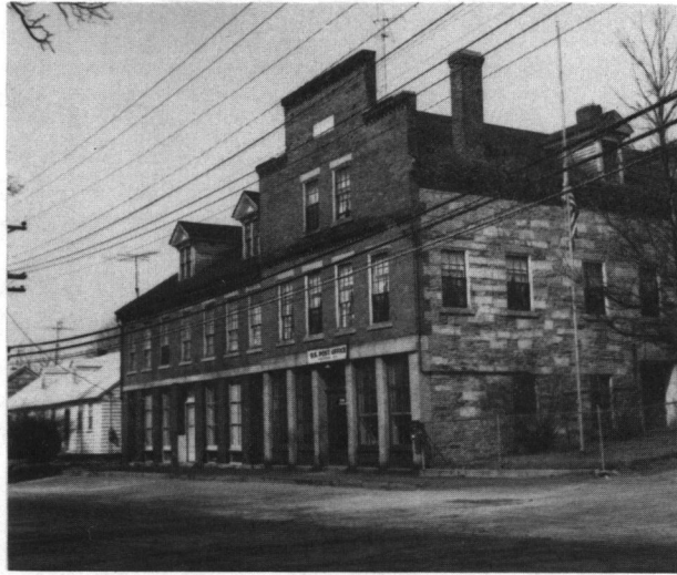
Commercial Block (1858): Main Street, Forestdale Historic District. (#2-D)
