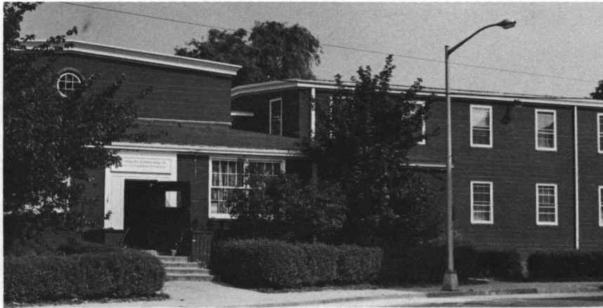
Figure 40: USO Building (Martin Luther King, Jr. Community Center), 1944; 20-28 West Broadway.
