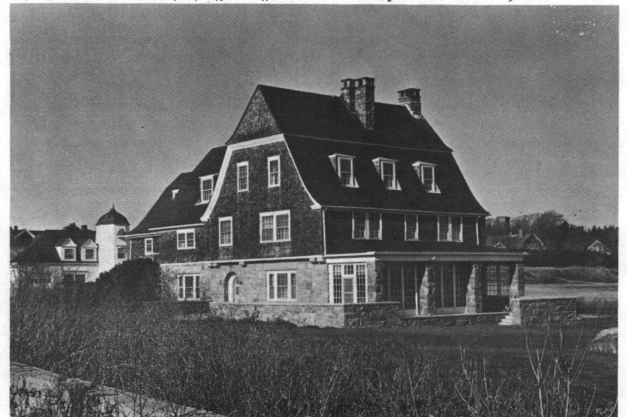
Fig. 17: Stone Lea, the George V. Cresson House (1883-1884, altered 1940s); 55 Newton Avenue; 1977 photograph.
