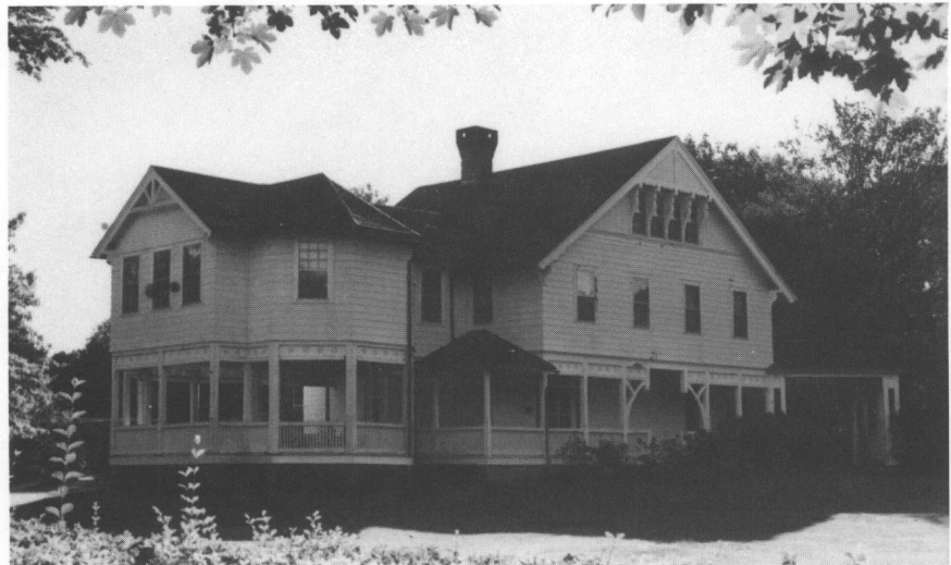
La Sata (1887), 94 Central Street. This dwelling, noted for its "Swiss Chalet" porch and gable ornamentation and the scrolled consoles on a row of four windows in the front gable, was built for John H. Shepard of New York.
