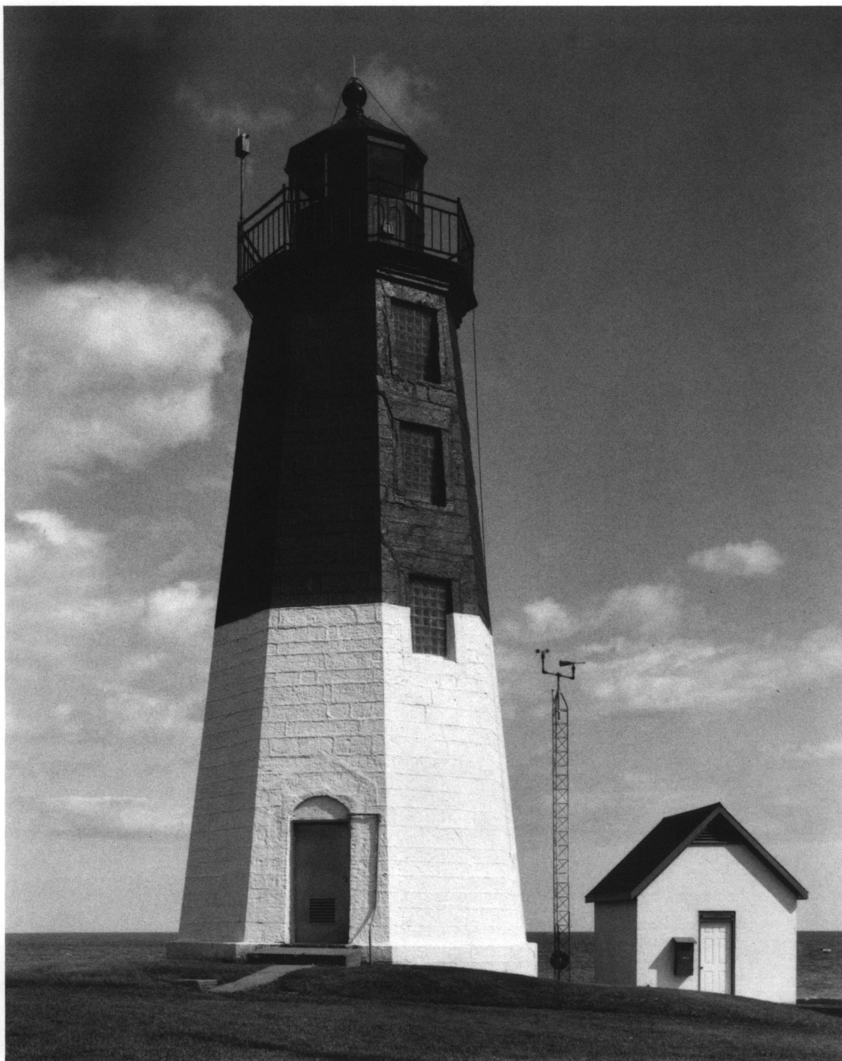
Point Judith Lighthouse (1857, 1862), 1470 Ocean Road. Photograph by Eugene Wick York. View of third tower on site; it has 24,000-candle-power and range of 16 miles. The adjacent small brick oil house (1917) was built to store fuel.
