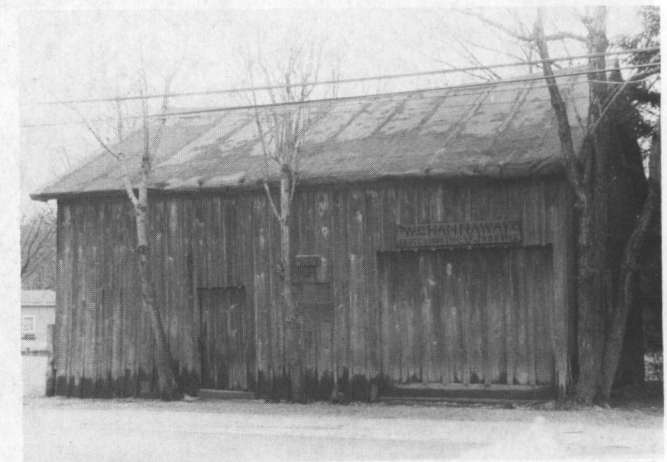
Fig. 26: Hannaway's Blacksmith Shop (late 19th-century); Great Road. The rare one-story, barn-like shed, clad with unpainted board-and-batten siding is a vital element of the Great Road Historic District.
