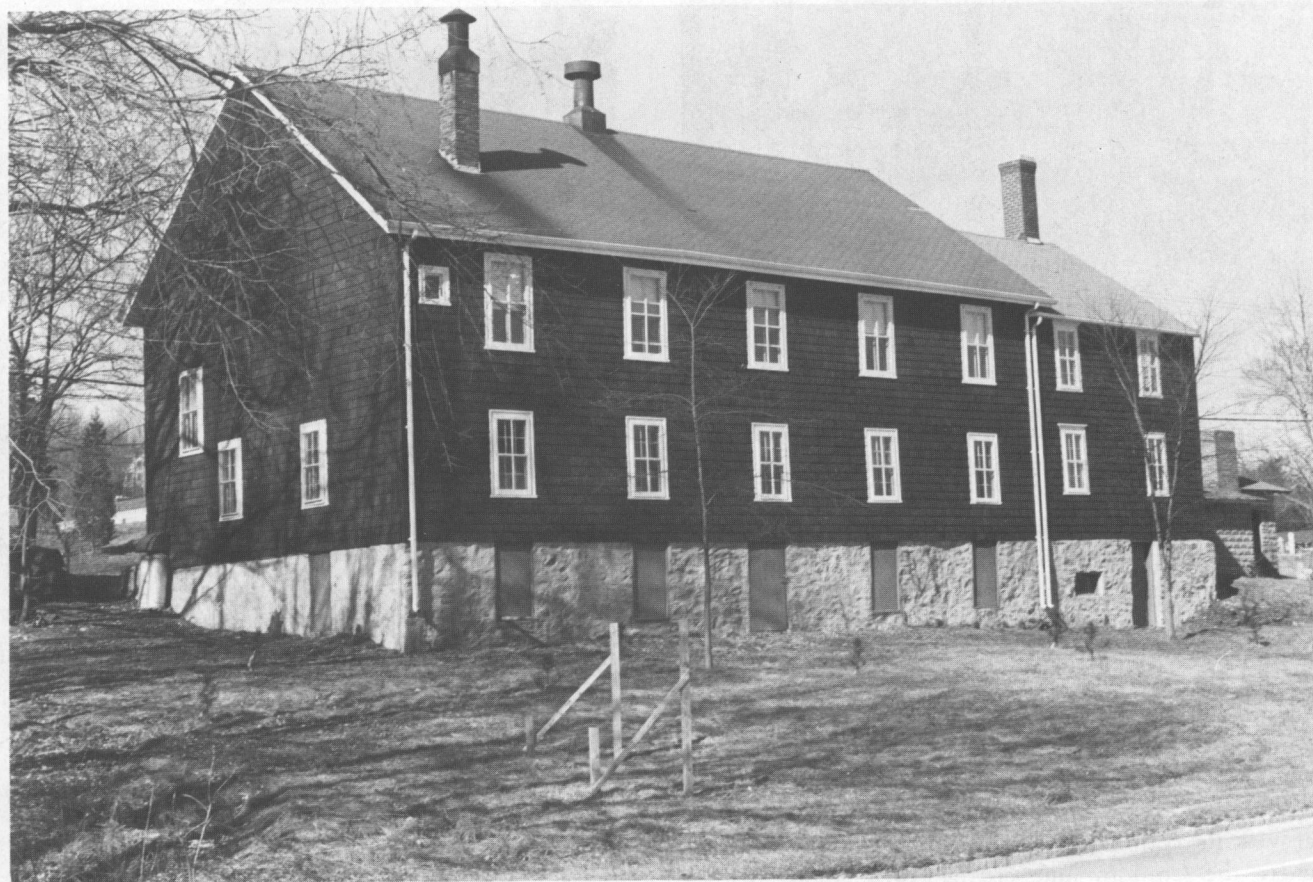
Fig. 18: North Gate (1807 and later); Old Louisquisset Turnpike; photograph, 1974. North Gate is a long gable-roofed building. Its six, unevenly spaced, bays reflect the several additions made since it was built as the northern toll house on the Louisquisset Turnpike.
