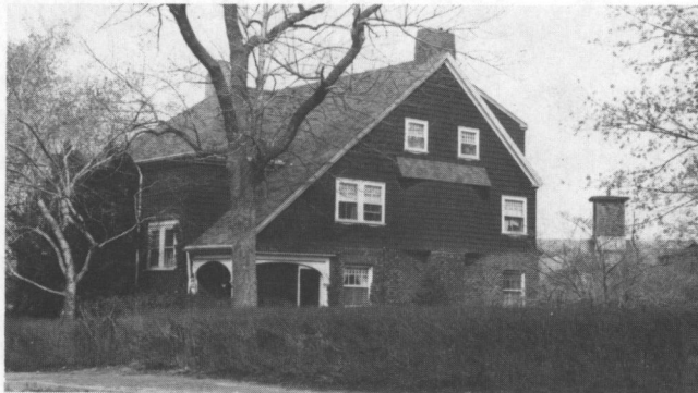
Fig. 13: 1693 Lonsdale Avenue (c. 1885): A Queen Anne house with long, sloping roof lines and contrasting wall materials.
