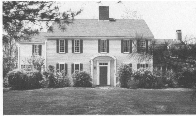
Fig. 5: 1730 Old Louisiquisset Pike (c. 1730): A classic, two-story, center chimney, five-bay, eighteenth-century house.
