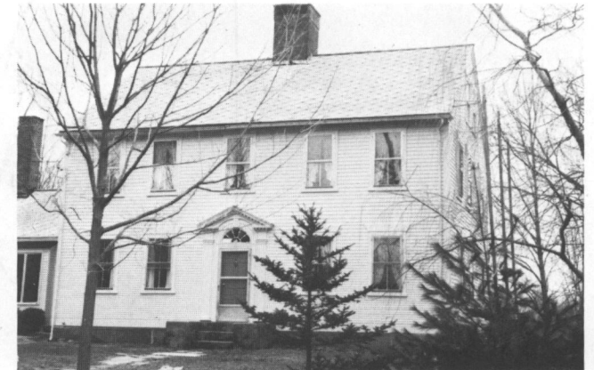
Fig. 7: Wilbur Road (c. 1790): A classic, center-chimney, gable-roof, Federal house with pedimented fanlight entrance.
