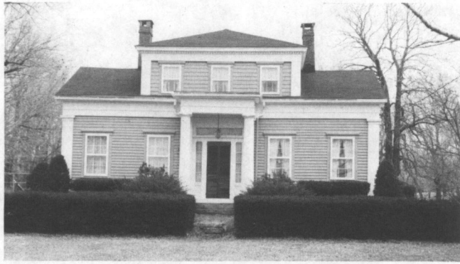
Fig. 9: Great Road (c. 1850): A one-and-one-half story, Greek Revival house with corner pilasters, raised central section and Doric porch.
