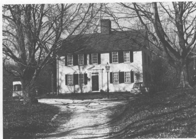
Fig. 27: Simon Aldrich House (c. 1760); Old Louisquisset Pike. Set at the center of the most complete early farm complex in Lincoln, the Aldrich House is a two-and-one-half story, five-bay structure with a large, brick, central chimney and pedimented central entrance.
