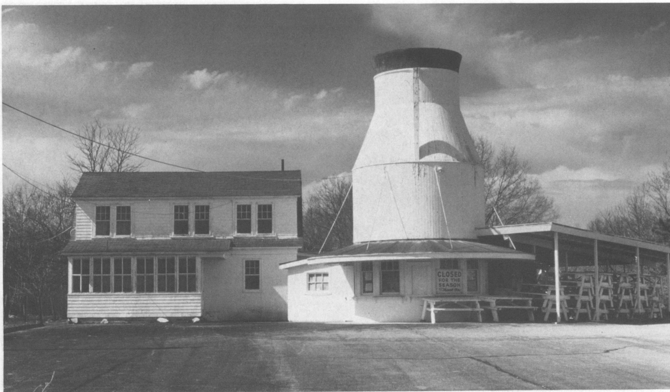
Fig. 58: The Milk Can (c. 1931); Louisquisset Pike. A wood-frame structure, constructed of vertical boards with diagonal sheathing, its exterior is covered with matched boards while the "cap" and "handle" are fabricated from sheet metal.
