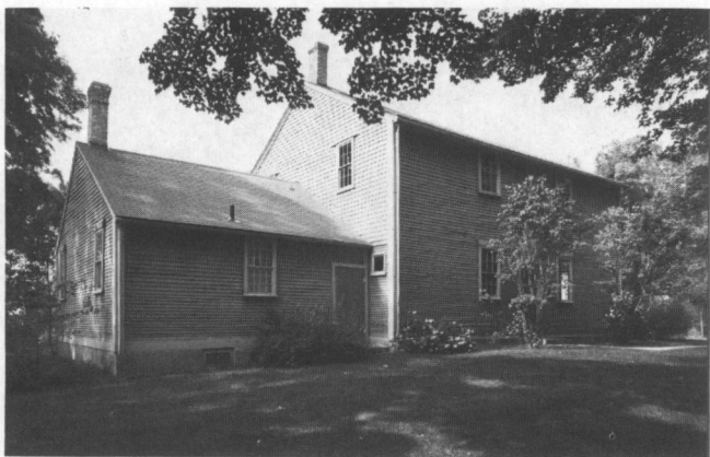
Fig. 7: Quaker Meeting House (1704, c. 1745); Chapel Street. Lincoln's oldest house of worship, the meeting house was built in two sections; the small, one-room, one story wing is the earlier section.
