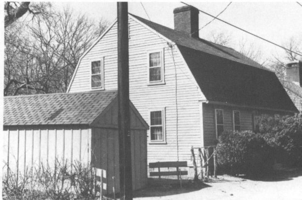
Fig. 4: 1016 Lower River Road (c. 1800): A common, eighteenth- to early-nineteenth-century, center chimney, one-and-one-half story house type.
