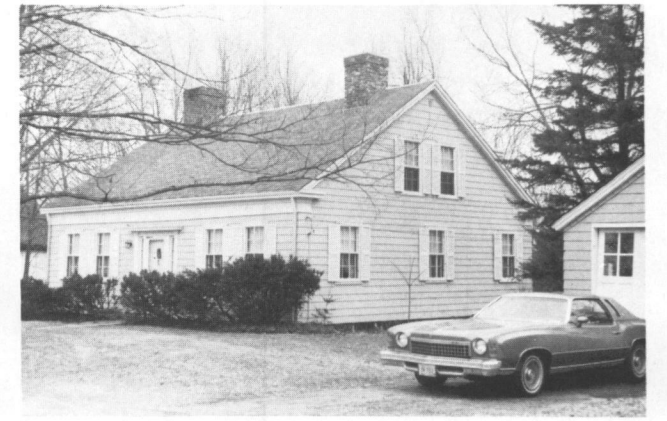
Fig. 8: Great Road (between 1840 and 1850): A one-and-one-half story, five-bay, Greek Revival house with a gable roof.
