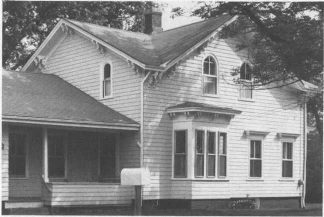
Fig. 10: 1406 Old Louisquisset Pike (c. 1850): A bracketed cottage with cross gable, bay window, and cornice brackets.
