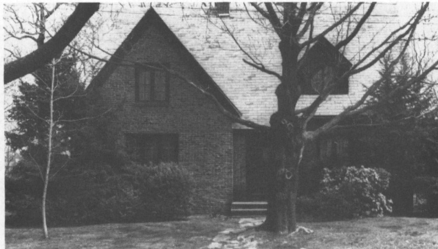
Fig. 21: 65 Read Avenue (1930): An early twentieth-century "English Cottage" of brick with a slate roof.
