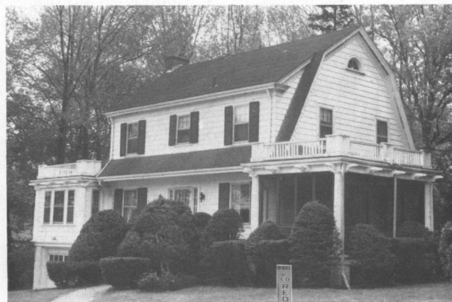
Fig. 22: 60 Progress Street (c. 1935): A typical, mid-twentieth-century, gambrel roof, suburban "colonial" house.
