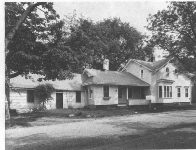
Fig. 10: Elliott-Harris-Miner House (c. 1710; c. 1850); 1406 Old Louisquisset Turnpike. Actually two separate dwellings joined by a middle wing, the gable-roofed house (on the left) seems to be Lincoln's earliest center-chimney house.
