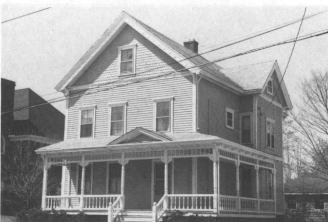
Fig. 14: 1570 Lonsdale Avenue (1897): A modest Queen Anne house with a wraparound porch, spindle work, and decorative bargeboard.
