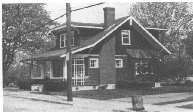
Fig. 19: 31 Walker Avenue (1920): A typical bungalow with wide overhanging eaves and a recessed porch.
