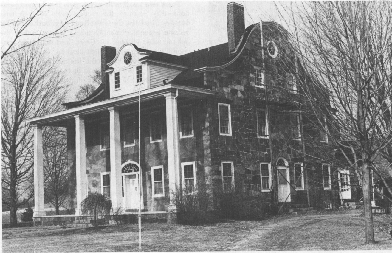
Fig. 25: Hearthside (1812); Great Road; photograph, 1978. Exterior features include rugged, picturesque, stone walls, ogee curves on the gable ends, and a two-story portico across the front.
