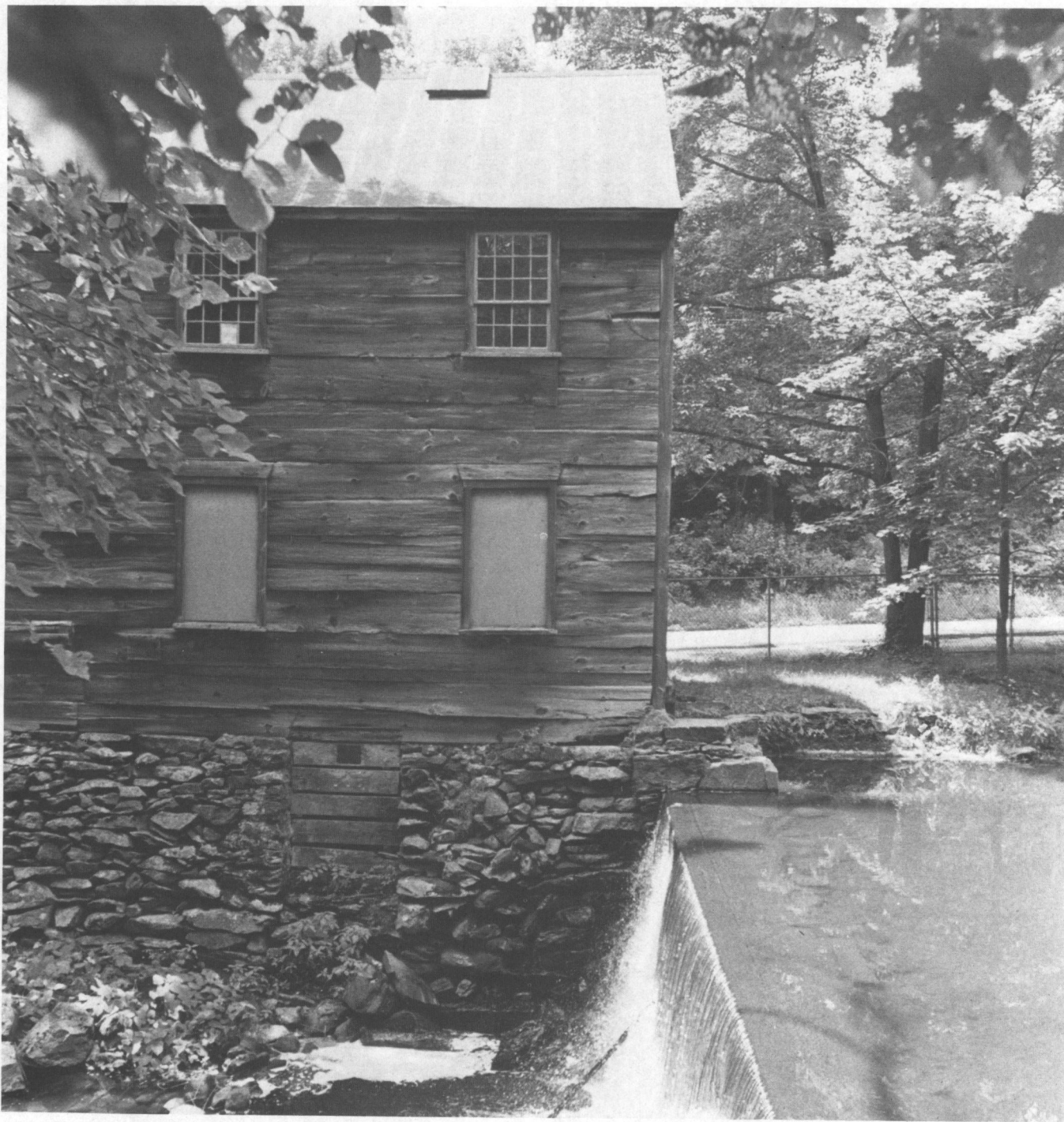
Fig. 23: Moffitt Mill and Dam (c. 1812); Great Road. The Moffitt Mill is a small two-story, gable-roofed, wood-frame building with a stone foundation and walls clad with wide board siding.
