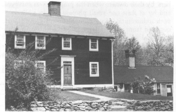
Fig. 6: Albion Road (1782): A simple, center-chimney, gable-roof, four-bay wide house of the Federal period.
