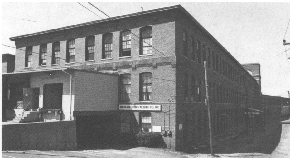
Fig. 64: Lonsdale Mill Complex (1833 through early 20th-century); Cook Street. The last great building project of the Lonsdale Company, the tower on the east side has lost its hip roof.
