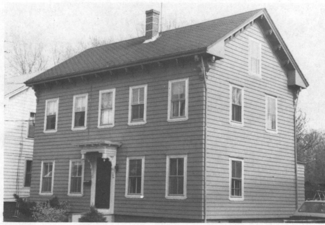
Fig. 12: 58 Union Street (c. 1880): A simple, two-story workers house with bracketed cornice and door hood.
