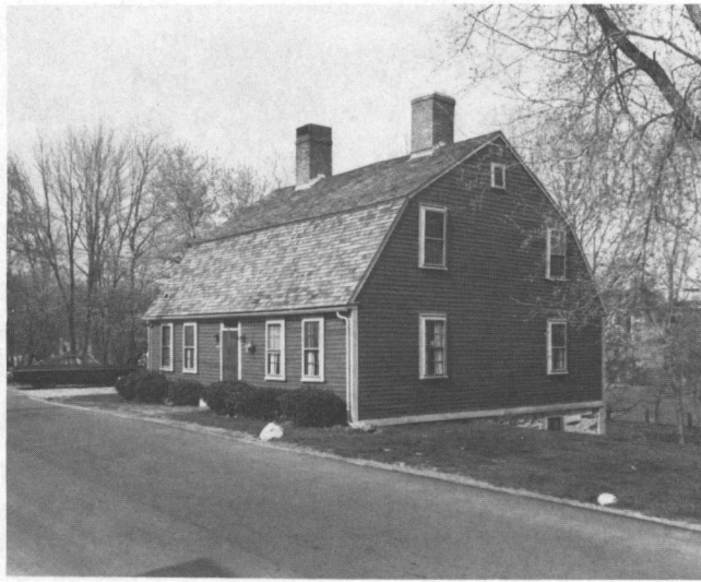
Fig. 37: Old Ashton Mill House (c. 1810); 1027 Lower River Road. One of four surviving houses built by Smithfield Cotton and Woolen Manufacturing Company.
