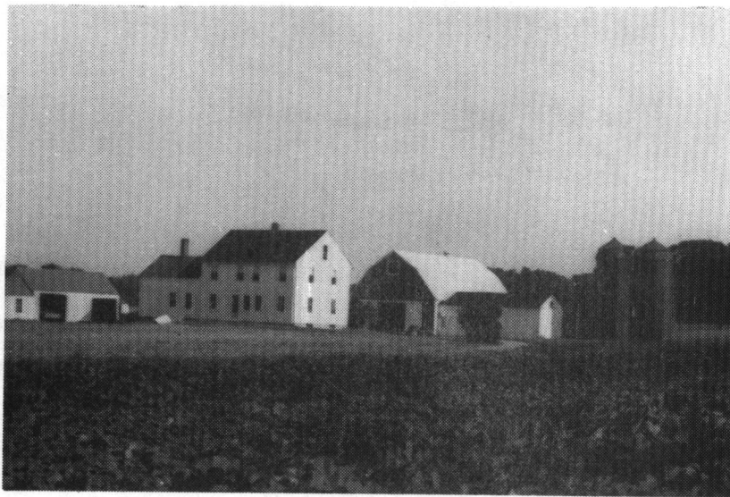
DAME FARM COMPLEX : Farm House, c. 1790, Sheds, c. 1790, Barn, 1910, Silos 1925, Brown Avenue. (Map #1.)
