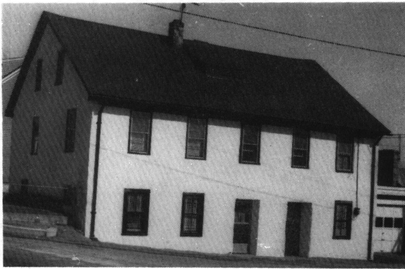
MILL HOUSE: c. 1850, Early Victorian, Simmonsville Avenue. (Map #20.)
