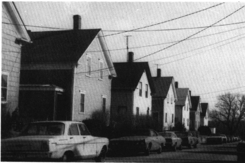
MILL HOUSES: early 20th century, Off Plainfield Pike, Thornton. (Map #67.)
