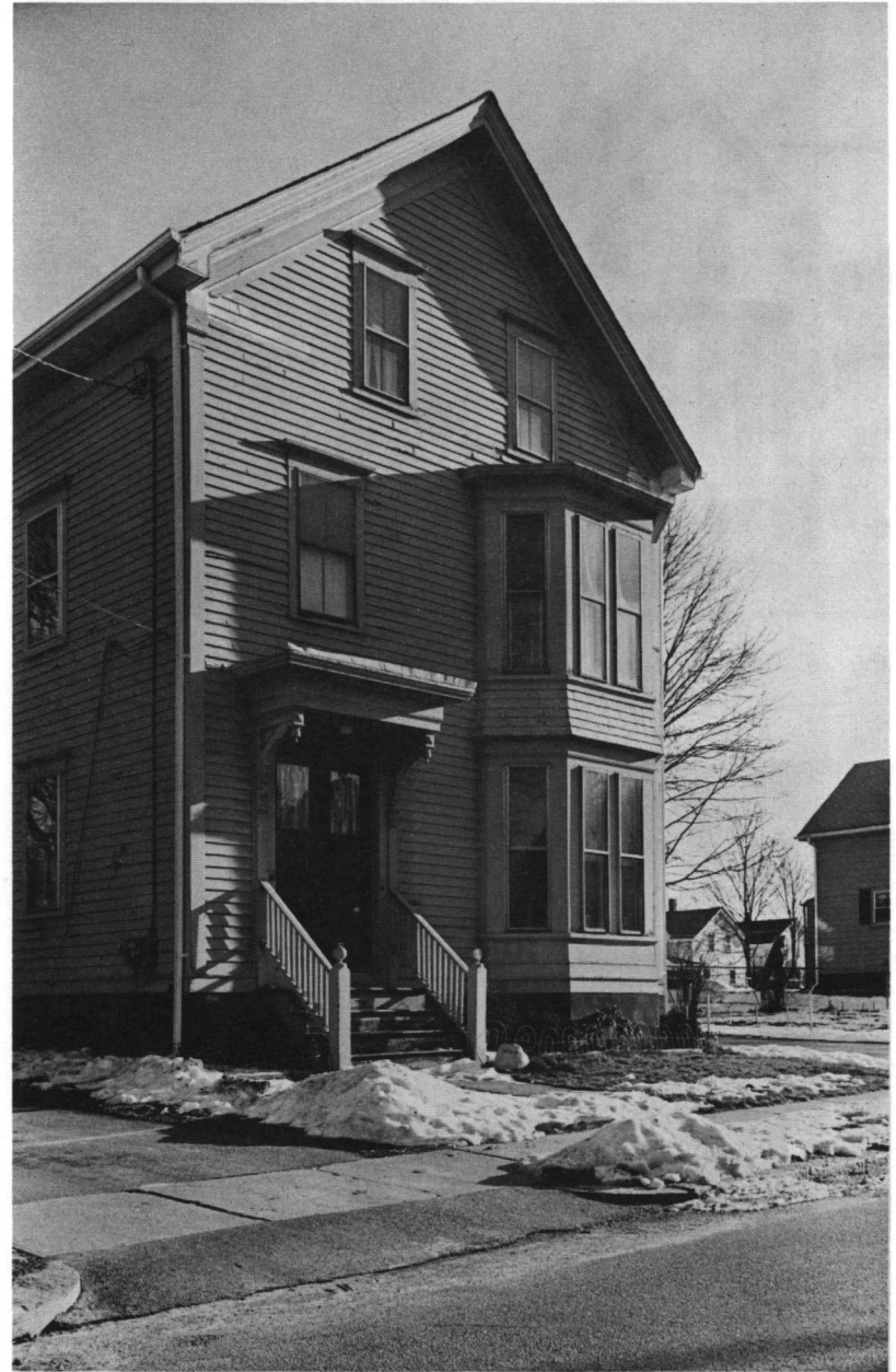
Fig. 31: Double house (ca. 1880s), 107 Vine Street.
