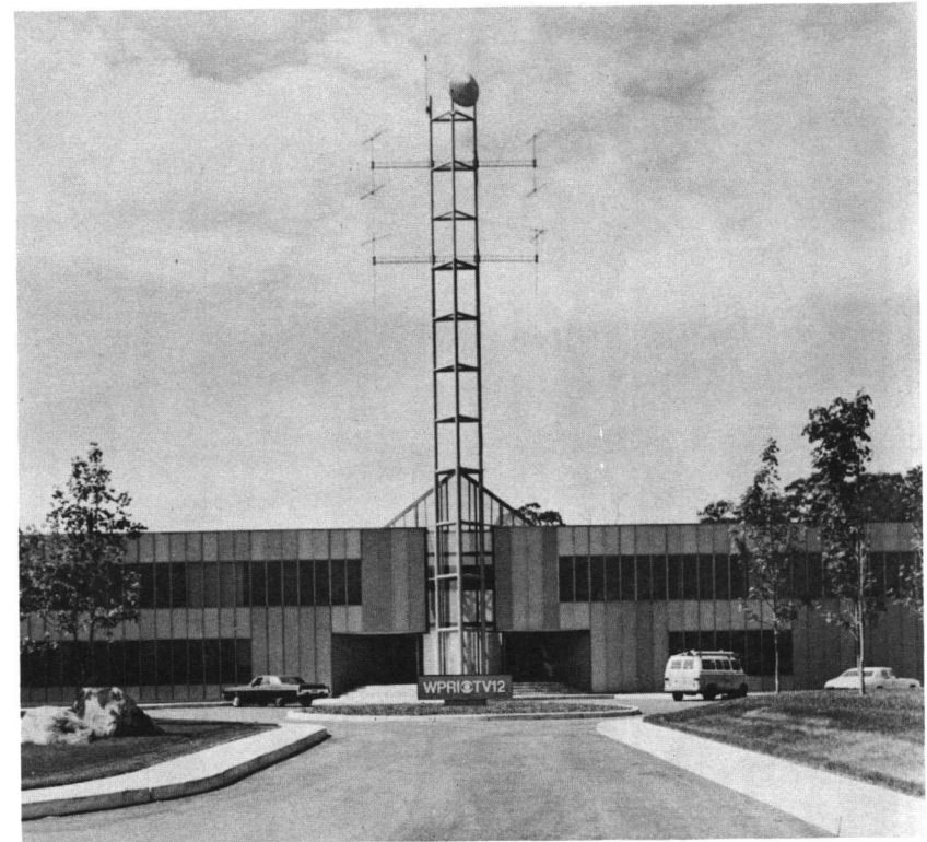
Fig. 74: WPRI Studios (1973-1974) William Kessler & Assoc., archs., 25 Catamore Boulevard.
