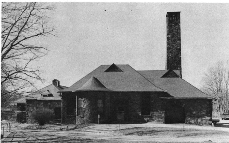
Fig. 44: Pumping Station (1893), Hunts Mills Road,
