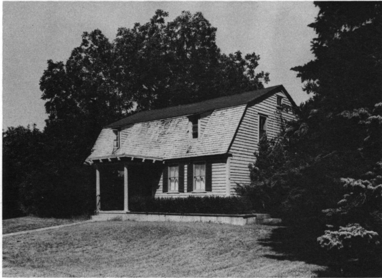
Fig. 10: House (ca. 1730s), 319 Willett Avenue.
