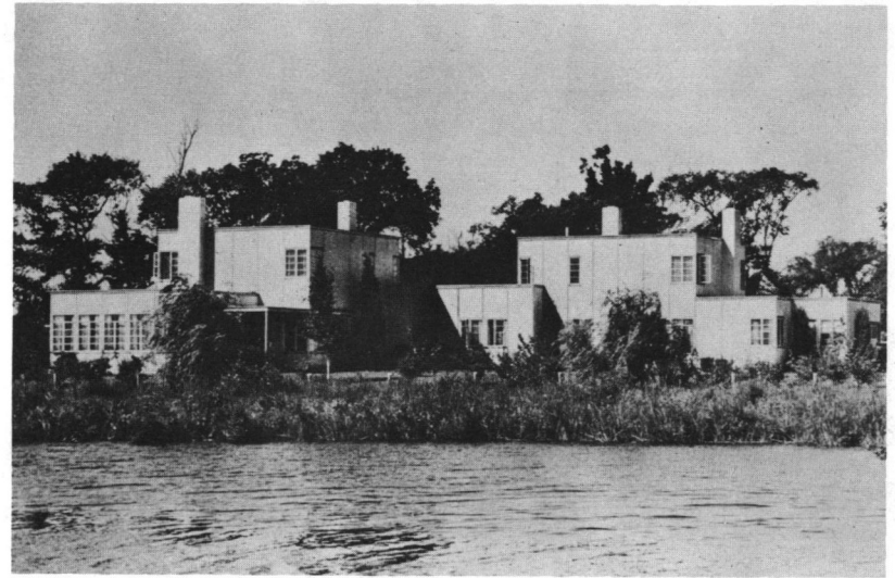
Fig. 66: Monsarrat houses (1936), General Housing Corp., des., 366 Newman Avenue.
