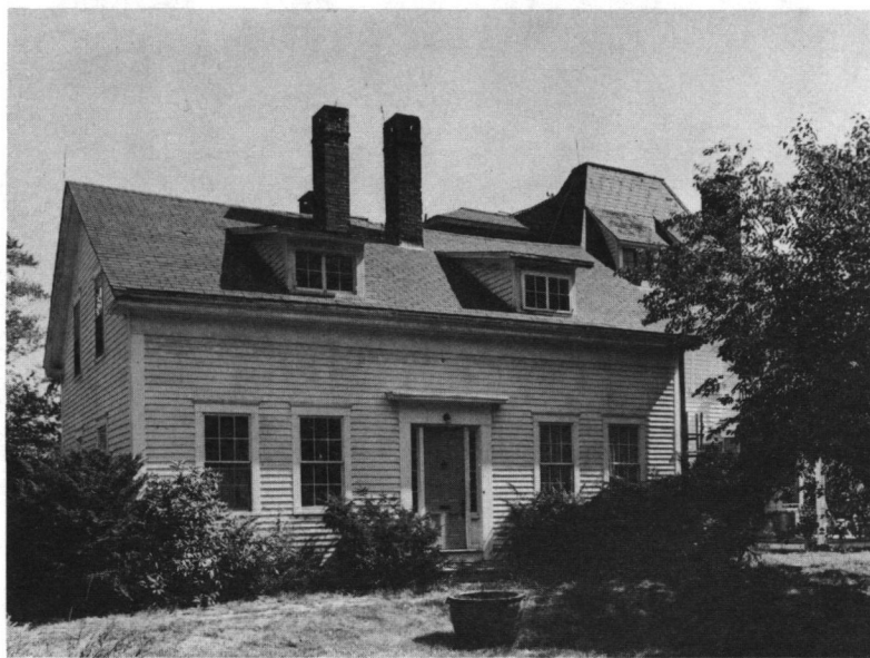
Fig. 19: Bridgham tenant house (1866), Nathan West, bldr., 150 Pleasant Street.
