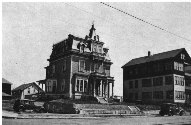
Fig. 25: Miles house (ca. 1870s) destroyed, and 3-decker, Waterman Avenue at James Street.
