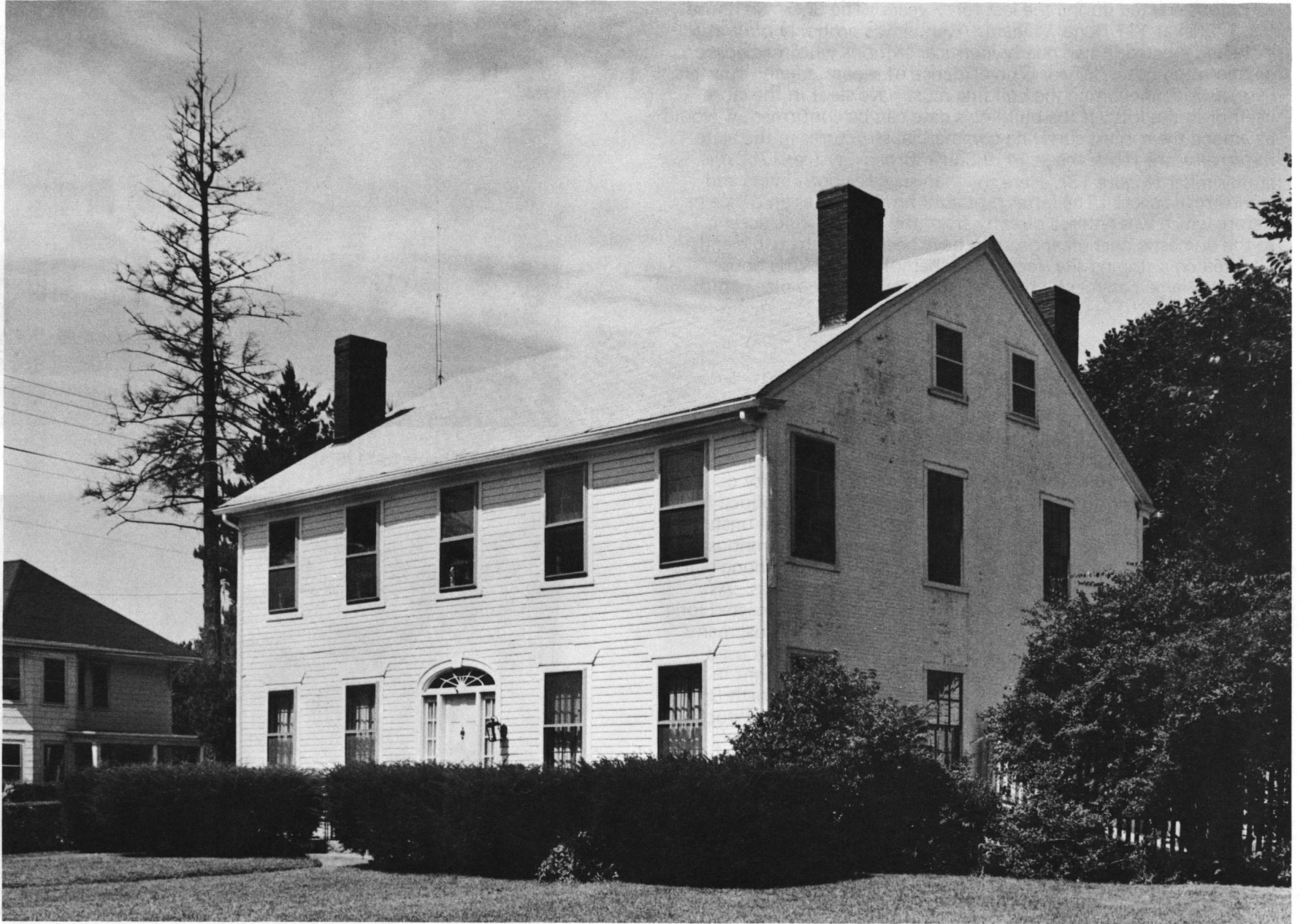
Fig. 14: Allin house (prob. after 1805), 36 Willett Avenue.
