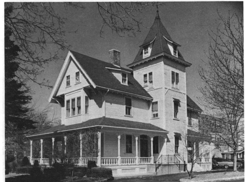
Fig. 22: Dennis house (ca. 1870s), 3120 Pawtucket Avenue.
