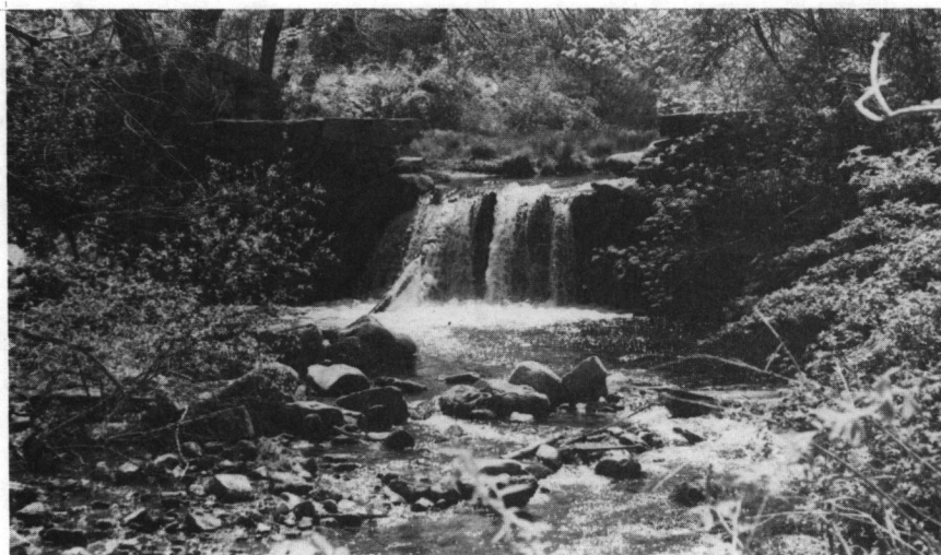
Dam along Tarkiln (18th Century et. seq.) at site of grist mill off Nichols Road, Oak Valley-Tarkiln Historic District (#12-H).
