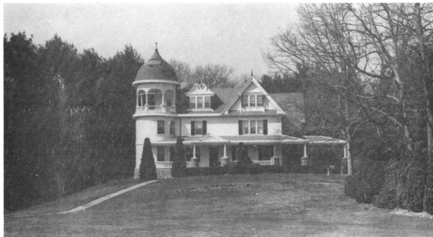
Ernest Tinkham House (1880-1882): 124 East Avenue, Harrisville Historic District (Map #7-M). Photo by Susan Dynes.
