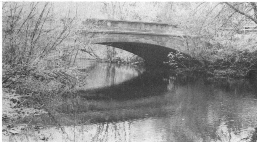
Oakland Bridge, Number 105 (1917-1918): Victory Highway, Oakland Historic District (#11-H).
