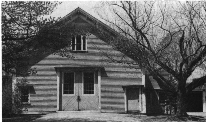
Barn (Late 19th-Century) at Superintendent's House: Victory Highway, Oakland Historic District (#11-D).
