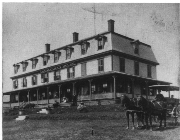
Connecticut House (c. 1880), Connecticut Avenue. Courtesy of Rhode Island Historical Society, view c. 1890.
