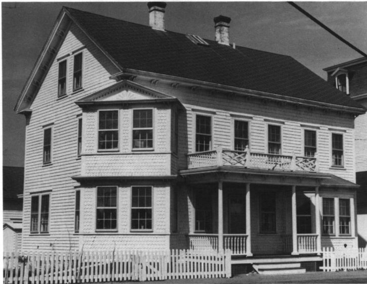
Bernal H. Dodge House Blue Dory Inn (c. 1870), Dodge Street. Rehabilitated using federal tax incentives.
