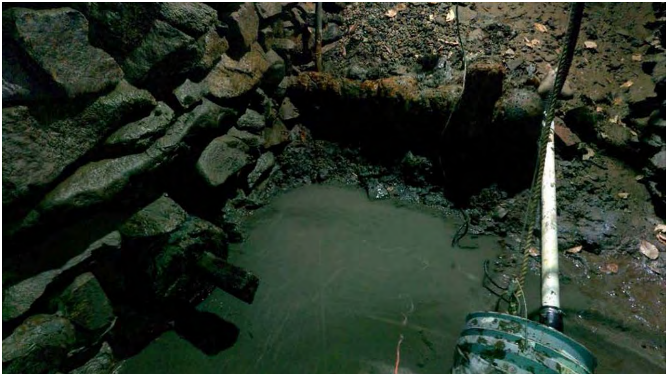
Figure 22. Spring box interior, view north, looking down (Newport Environmental 2018: Image 12b).
