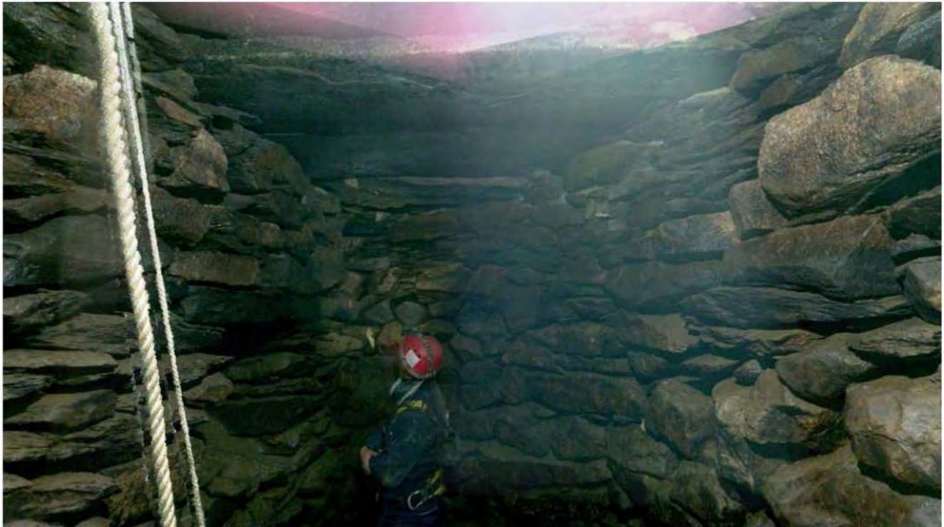
Figure 19. Spring box interior, view south, looking up (Newport Environmental 2018: Image 11a).
