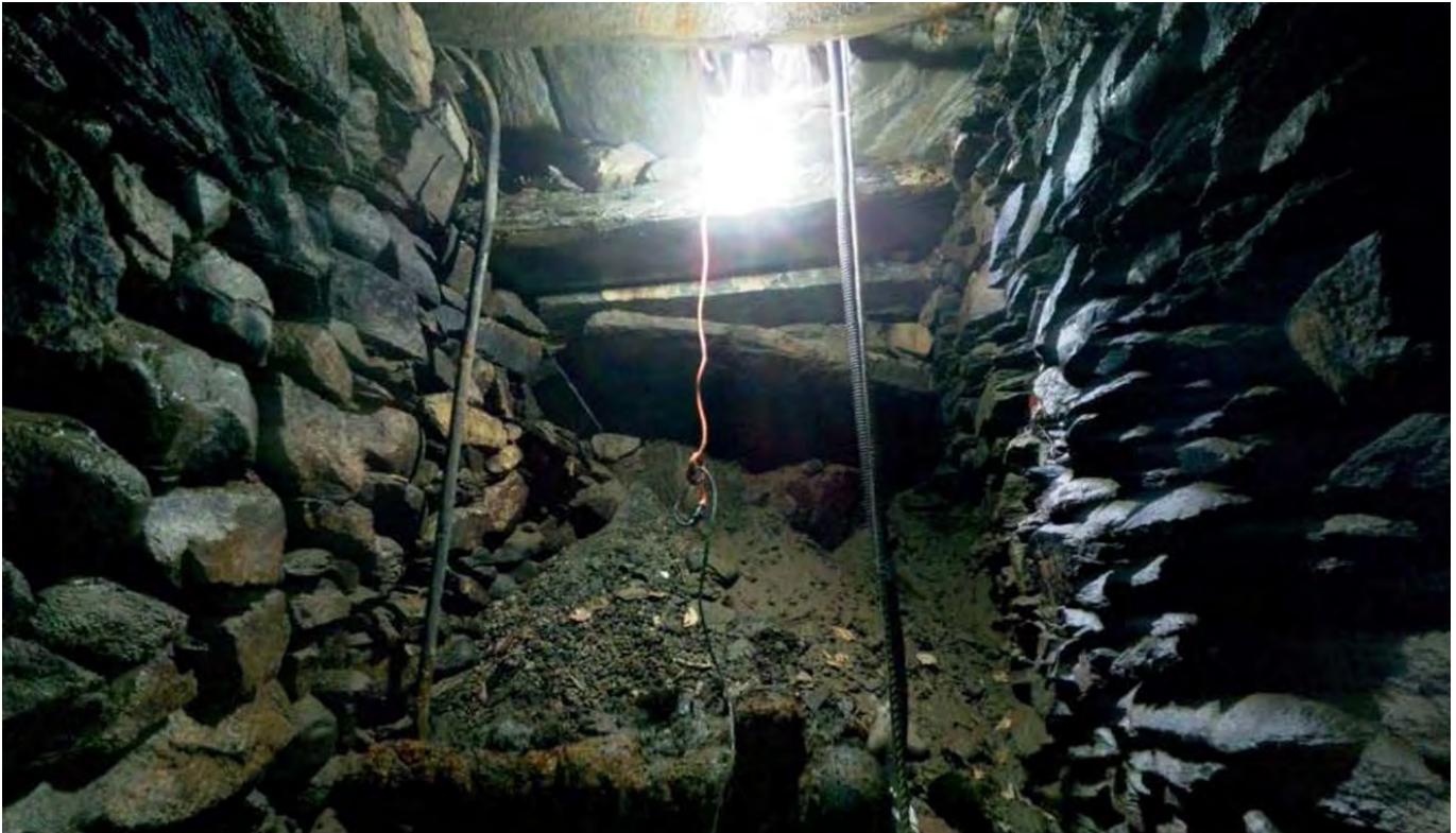
Figure 21. Spring box interior, view north, looking up (Newport Environmental 2018: Image 12a).
