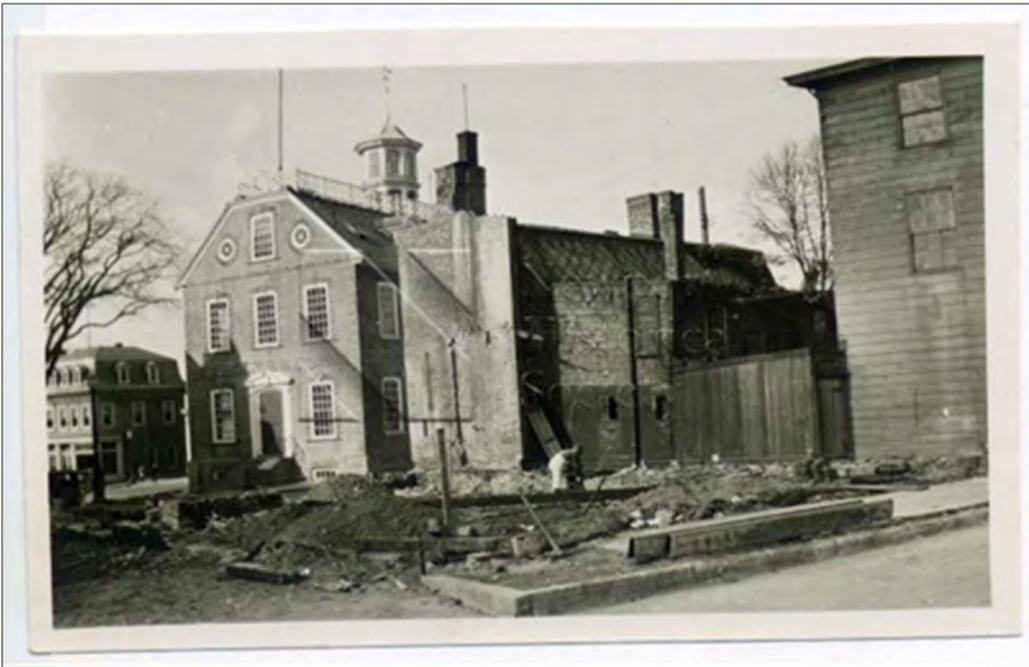
Figure 13. Undated photo of demolition work at the spring lot.
