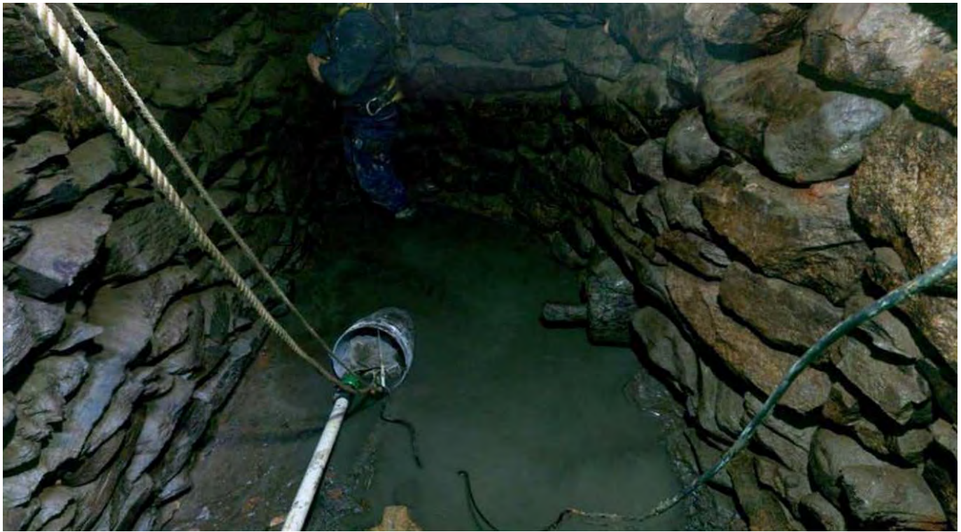
Figure 20. Spring box interior, view south, looking down (Newport Environmental 2018: Image 11b).
