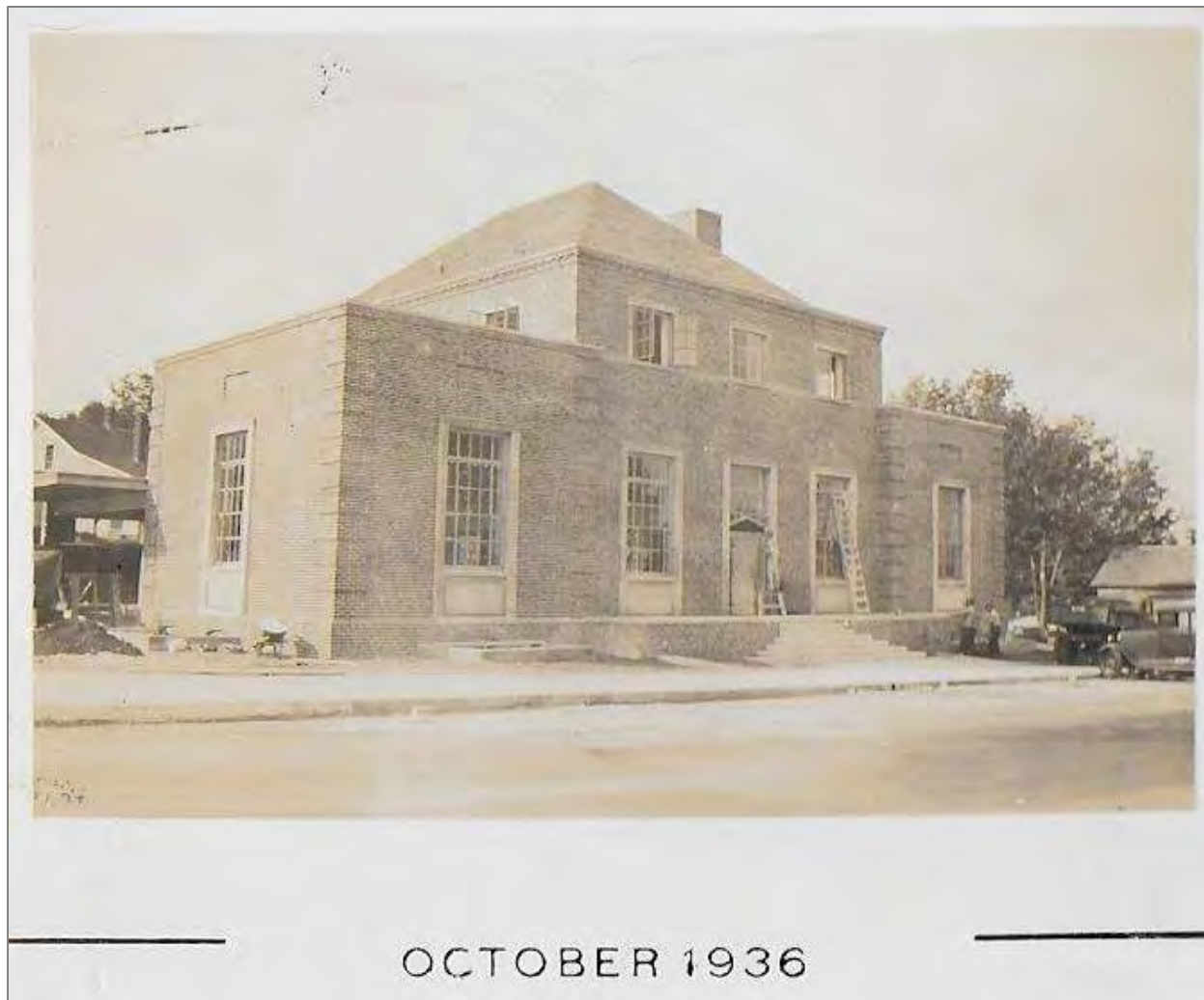
Figure 4 Former Wakefield Post Office, 238 Robinson Street, South Kingstown. View looking southwest, October 1936.
