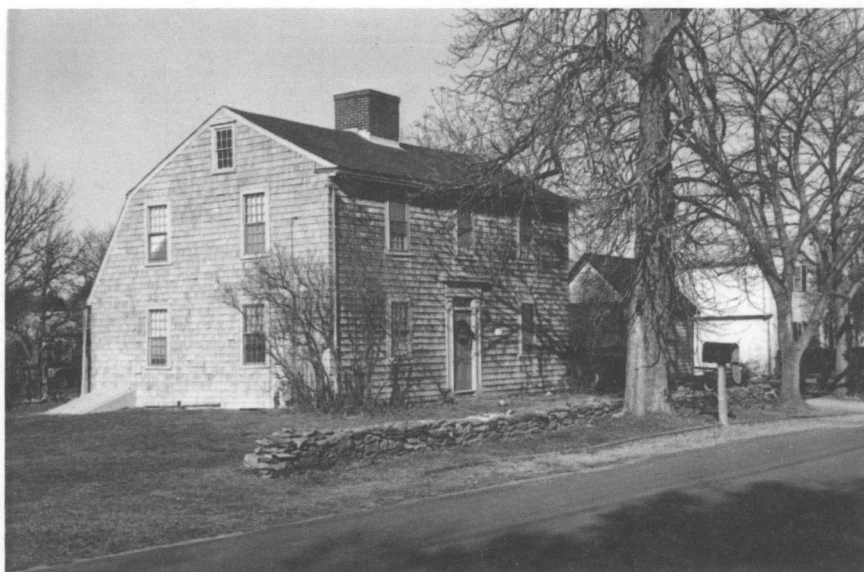
Nathaniel Heath House (1782), 38 Old River Road. Photograph by Bradford R. Smith, 1980. One of two unusual houses in town with gambrel-saltbox roofs.
