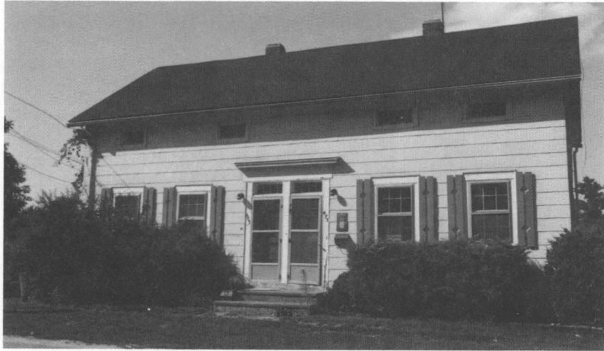
Mason Barney House (ca. 1840), 473-75 Sowams Road. This is a rare Barrington example of a common nineteenth-century double house type, with paired central entrances leading to separate units at each end of the house.
