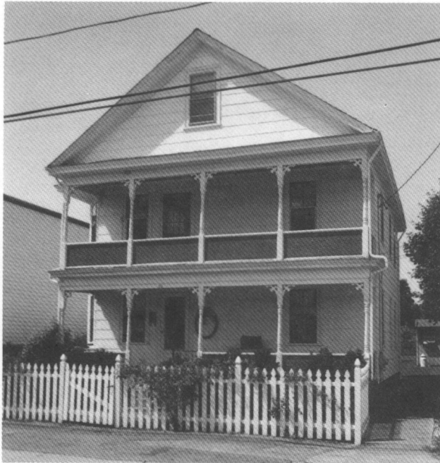
Alfredo Farina House (ca. 1910), 53 Maple Avenue. A typical double-decker residence with separate dwelling units on each story, fronted by an airy 2-story porch recessed under the roof mass.
