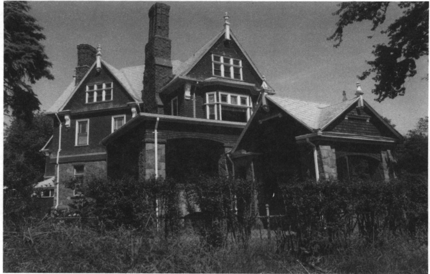
Leroy Fales House (ca. 1895), 32 Lorraine Avenue. Photograph, 1987. A very large, asymmetrical English Medieval Revival residence with multiple gables decked with finials and chimneys with pilastered tops.
