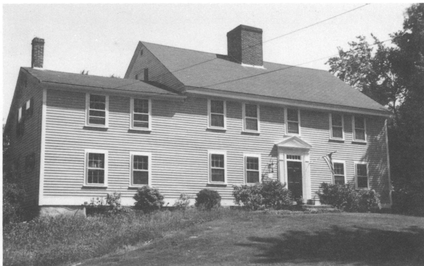
General Thomas Allin House (1783), 20 Lincoln Avenue. Photograph, 1993. A typical 2-1/2-story Georgian Colonial dwelling with a 5-bay facade, central entrance, and center chimney, with a later 2-bay addition on the west. The door pediment was reconstructed in 1952 to replace the original one which had been removed.
