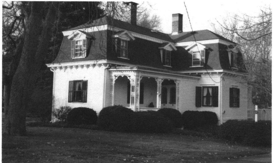
Allen C. Mathewson House (ca. 1862), 48 Jenny's Lane. The bell-curve mansard roof with bracketed cornice and chevron pattern band between the roof slopes contributes greatly to this house's distinctive architectural character.
