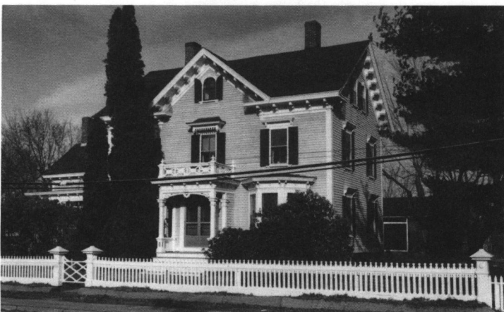
Albert G. Peck House (1865), 955 County Road. A fine Italianate dwelling with deep window cornices, a flaring hood over the center window, an arched window in the front gable, and brackets trimming the portico, bay window, and eaves.
