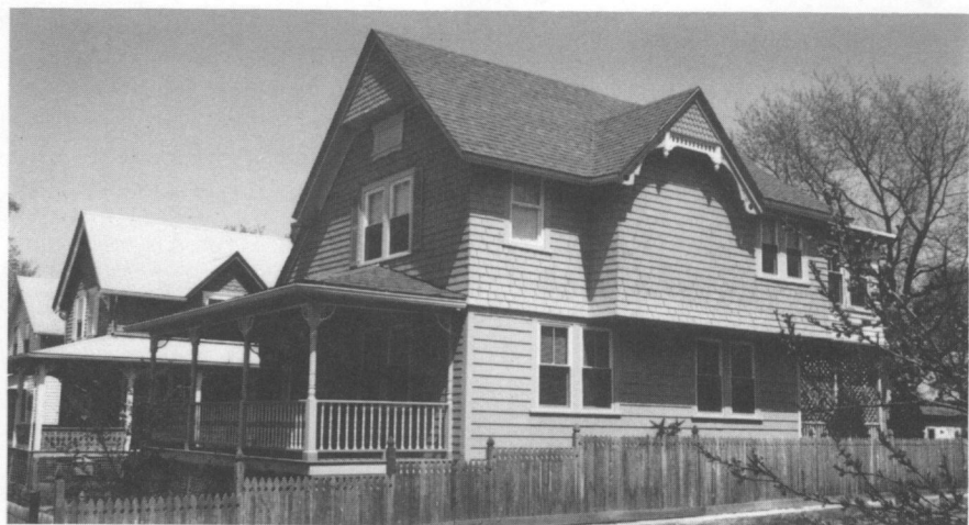
Thomas H. Bell Cottages (1901-09), 16 and 20 Edwin Street, Bay Spring. Two small summer houses, set on typical 50-foot wide lots. Detailing includes decorative shingling, vergeboards, brackets, and full-width porches.
