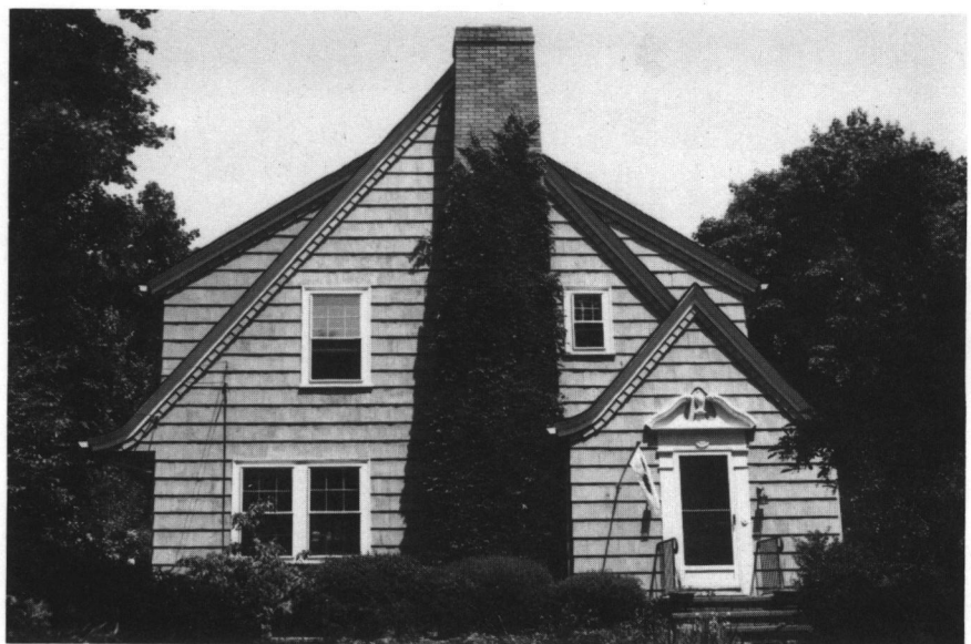
Anderson-Law House (1927), 26 Lincoln Avenue. An English Cottage style dwelling with end- gable roof, prominent front chimney, and off-center projecting entrance pavilion. The American Colonial pedimented doorway is typical of the mixed stylistic detailing found on such houses.
