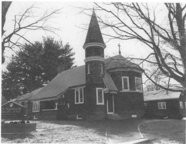
St. Matthew's Episcopal Church (1891), 5 Chapel Road. William R. Walker and Son, architects. A small shingled Queen Anne/Gothic Revival building with a polygonal bay and 3-stage cylindrical tower on the facade.
