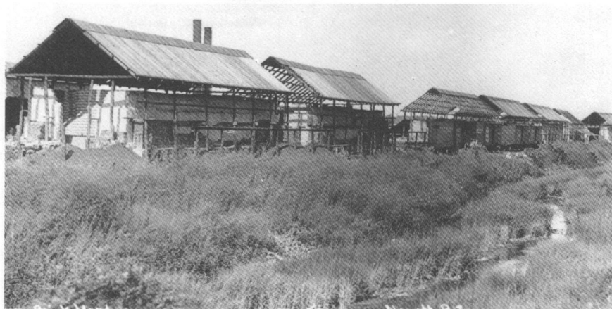
Brick Drying Sheds. Postcard view, ca. 1905. Courtesy of Barrington Preservation Society, Nicholas Gizzarelli collection. These open sheds once lined Brickyard Pond, which was formed by flooding excavated clay pits.
