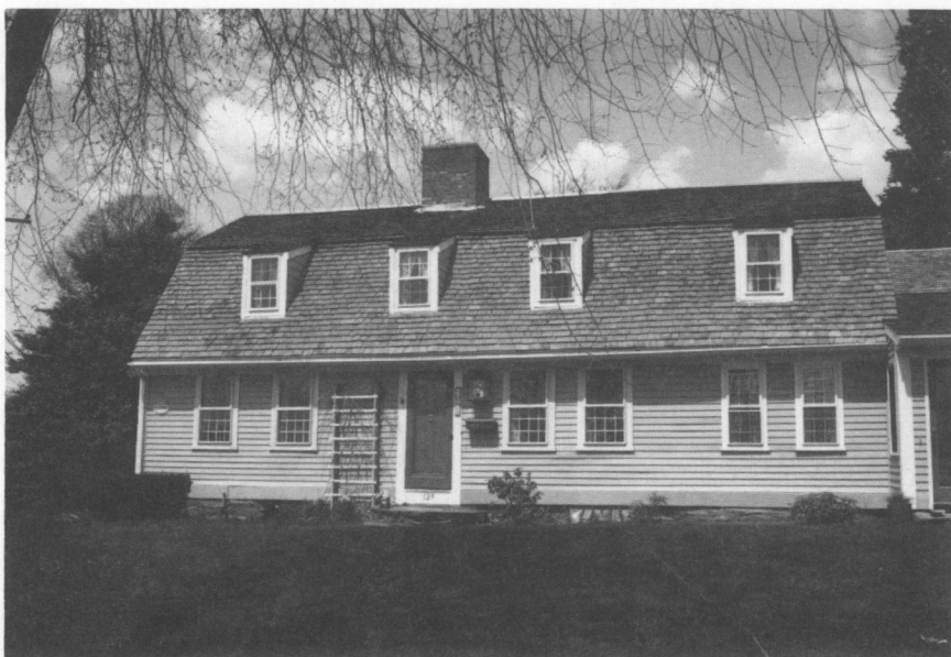
James Martin House (1786 et seq.), 125 New Meadow Road. A Colonial house of the 1-1/2-story, gambrel-roof type, with two additional bays added to the east.
