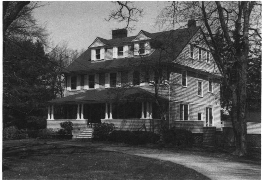
Arthur F. Kidder House (ca. 1900), 16 Jenny's Lane. An excellent example of a Modern Colonial style residence modeled after 17th- and 18th-century New England domestic architecture.
