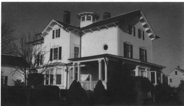
Jesse Davis House (ca. 1850), 12-18 Tyler Point Road. A good example of an Italianate villa, with cross-plan massing, bracketed cornice, and cross-gable roof topped with an octagonal cupola.
