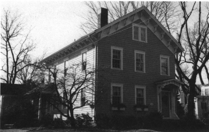
Lewis T. Fisher House (1863), 33 Jenny's Lane. This end-gable, side-hall-plan house has an Italianate hood over the main entrance and bracketed eaves.
