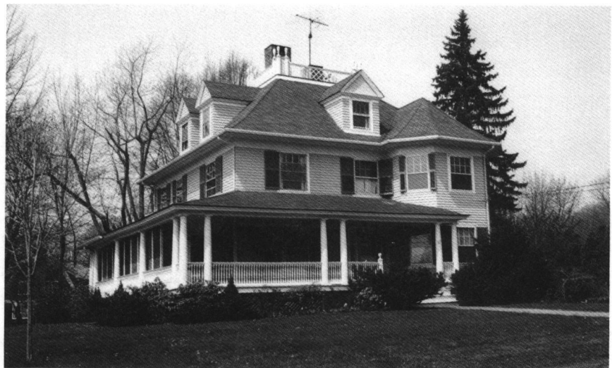
George Howard Smith House (ca. 1895), 217 Washington Road. A high-style Colonial Revival residence with characteristic Tuscan column veranda, shutter-trimmed windows, pedimented gable dormers, and roof balustrade. The polygonal corner bay, a feature not seen on real Colonial houses, is a typical embellishment found on Colonial Revival dwellings.
