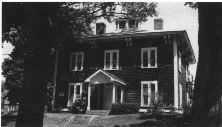
The Rev. Francis Horton House (ca. 1870), Federal Road. An illustrative example of the Italianate palazzo house type, with cubical form, symmetrical facade, paired narrow windows, bracketed cornice, and hip roof capped with a central cupola. The present front entrance portico is a later addition.
