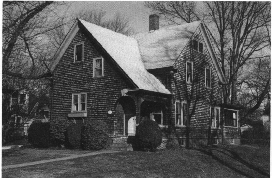
Henry and Lucy Anthony House (1892), 50 Walnut Road. The relatively simple geometry, uniform shingle wall surface, and lack of extensive ornamentation seen here are hallmarks of the Shingle Style.
