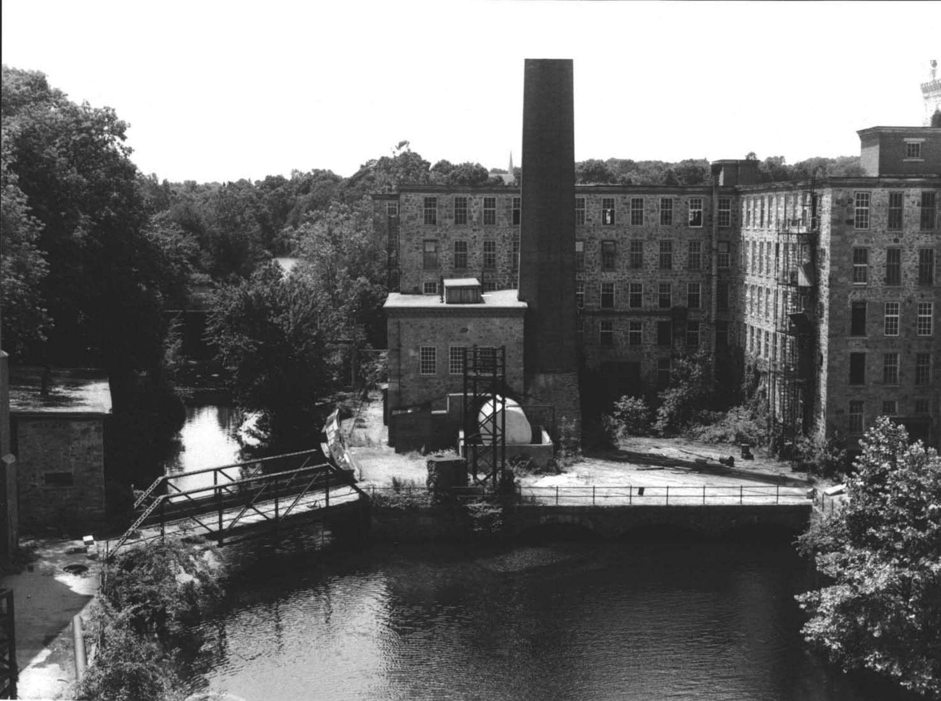
ROYAL MILL COMPLEX KENT COUNTY, RI No. 4
