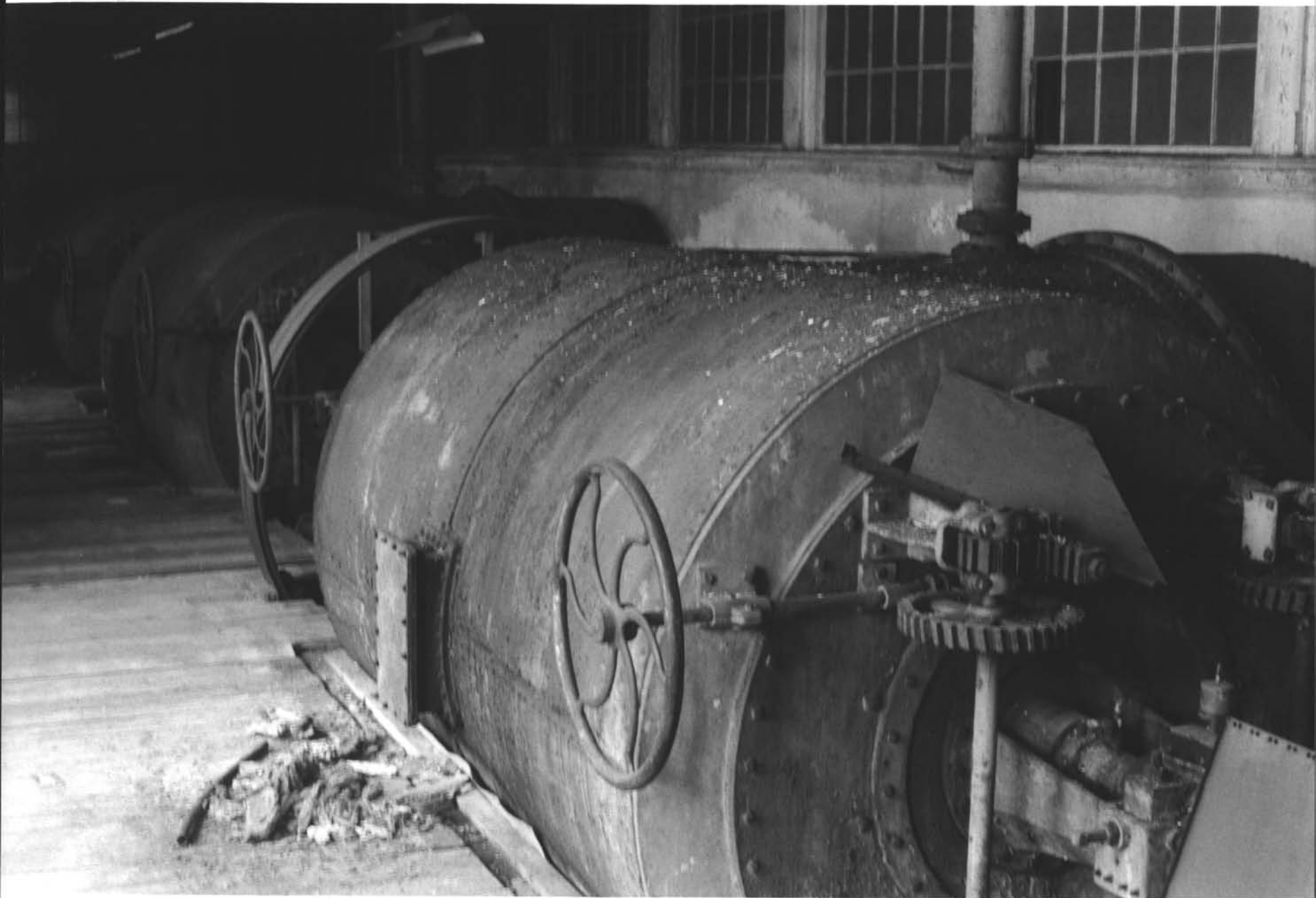
ROYAL MILL COMPLEX KENT COUNTY, RI No. 5
