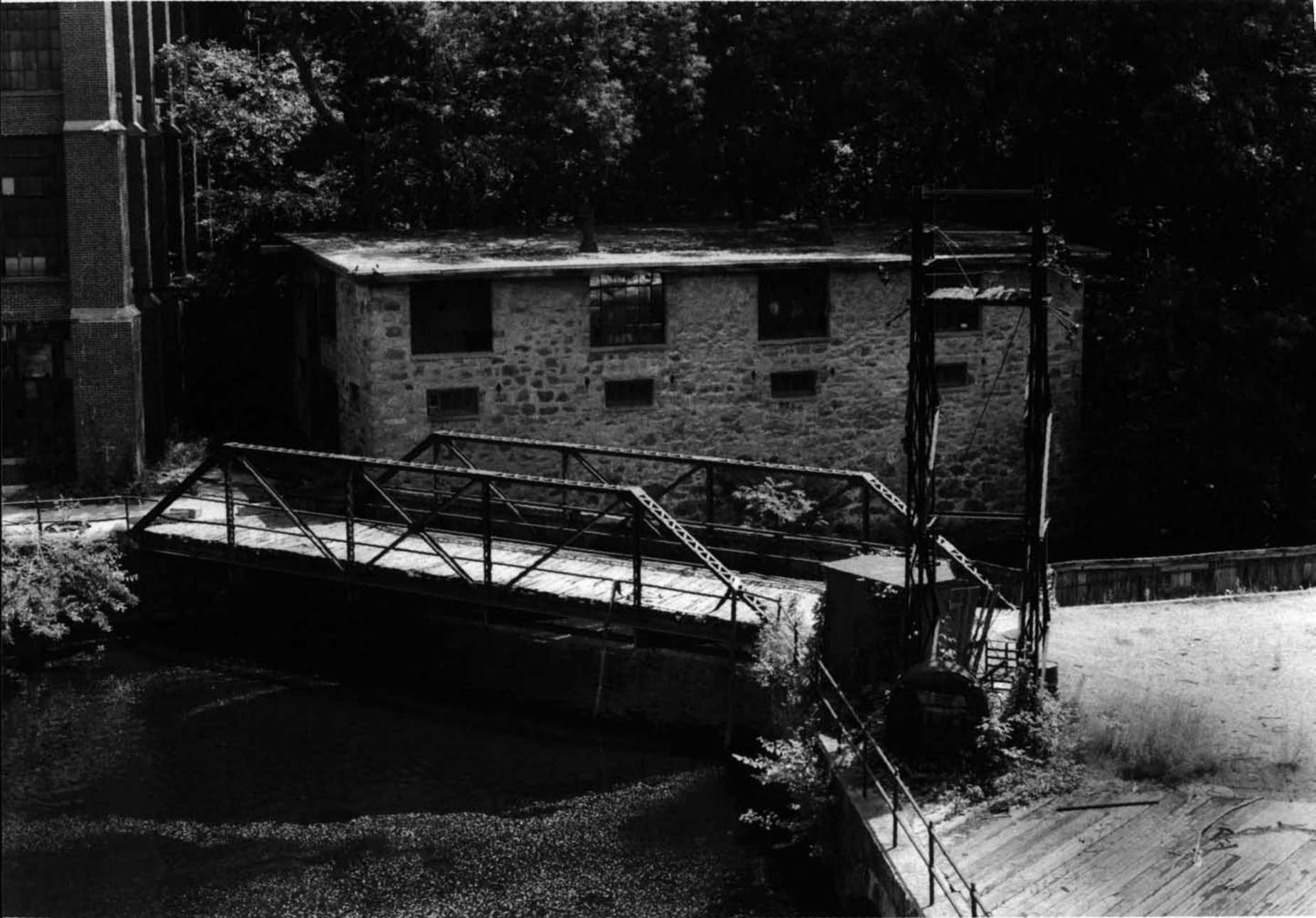
ROYAL MILL COMPLEX KENT COUNTY, RI No. 9
