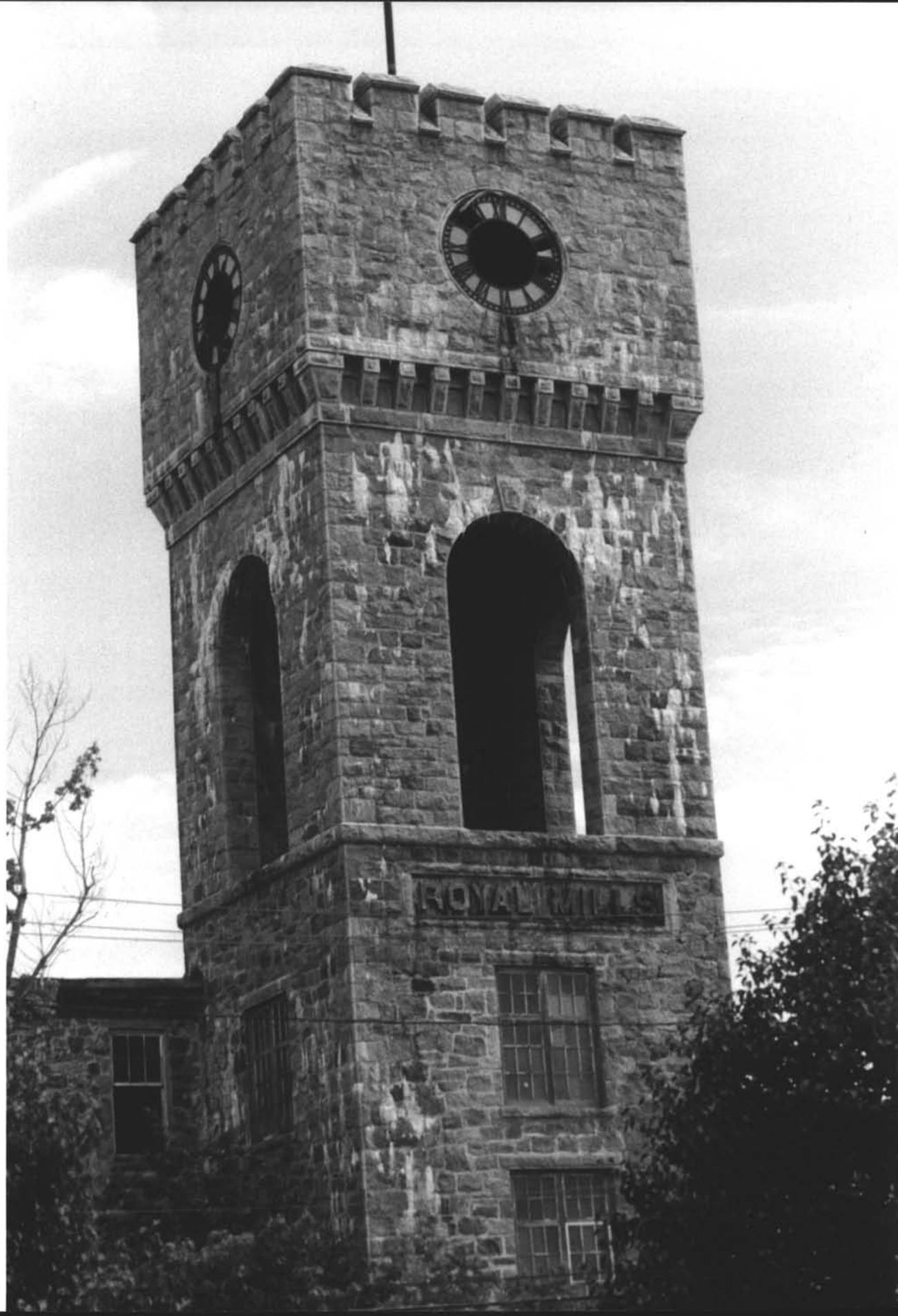
ROYAL MILL COMPLEX KENT COUNTY, RI No. 2
