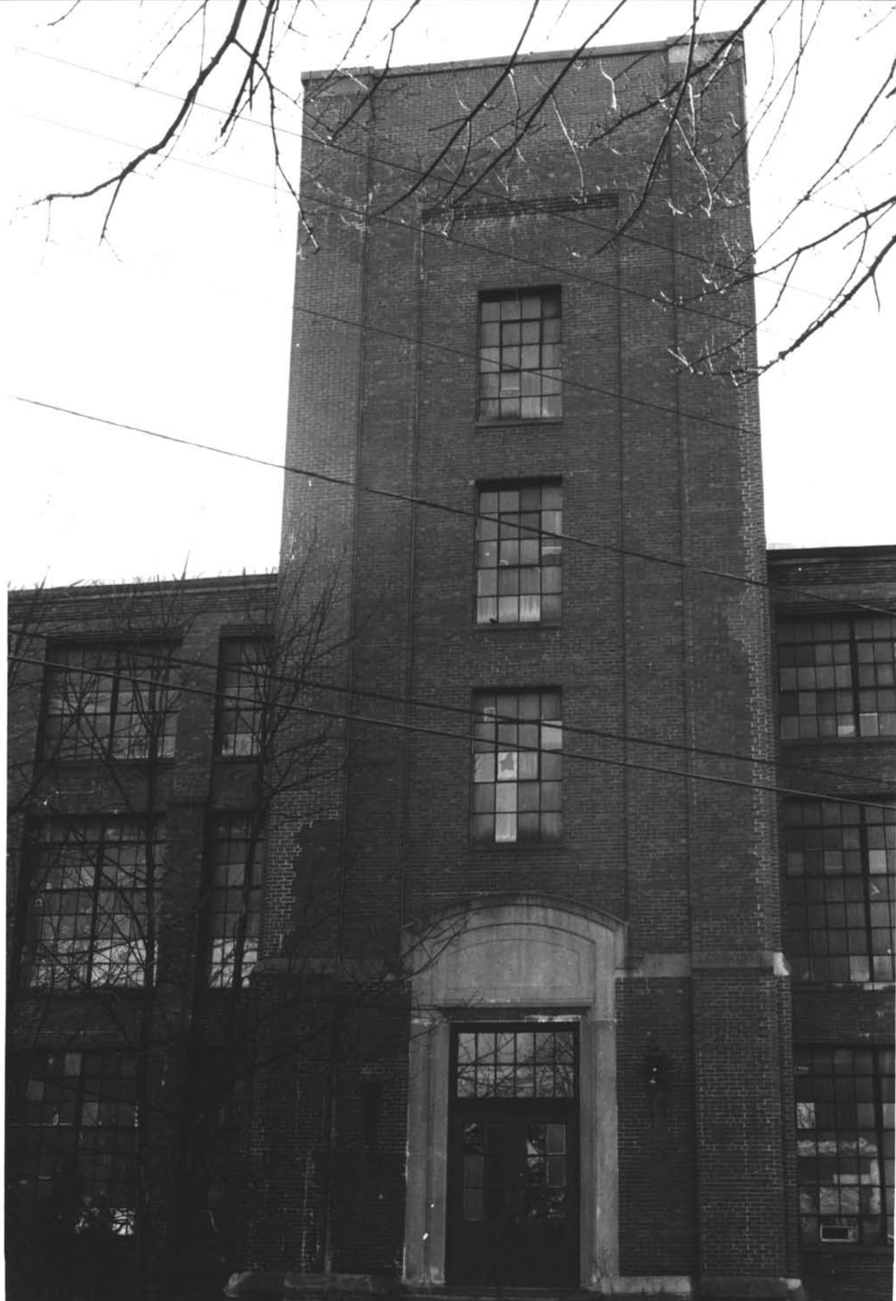
ROYAL MILL COMPLEX KENT COUNTY, RI No. 7
