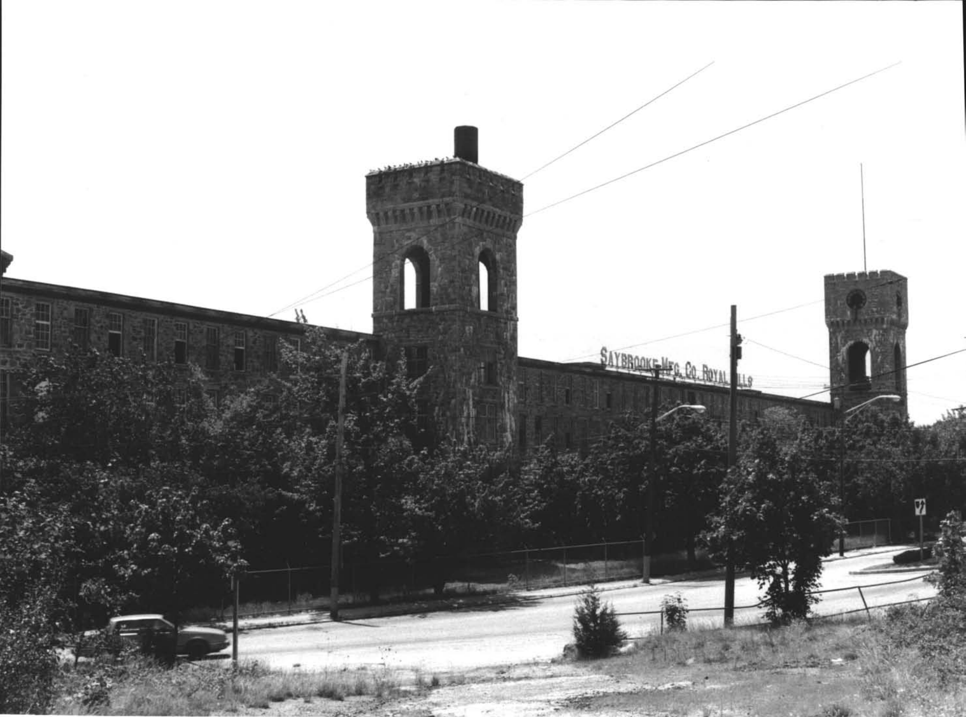
ROYAL MILL COMPLEX KENT COUNTY, RI No. 1
