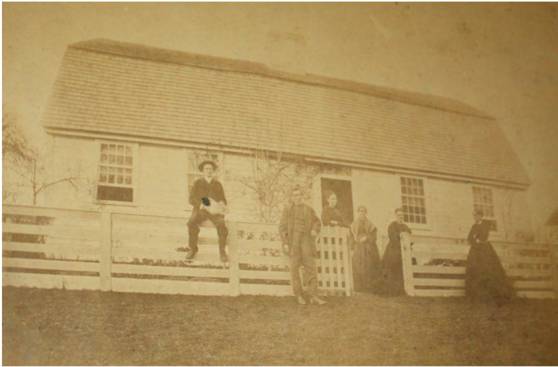
FIGURE 4 – historic photo of the Samuel Clarke Farm house, ca. 1865, looking northeast.
