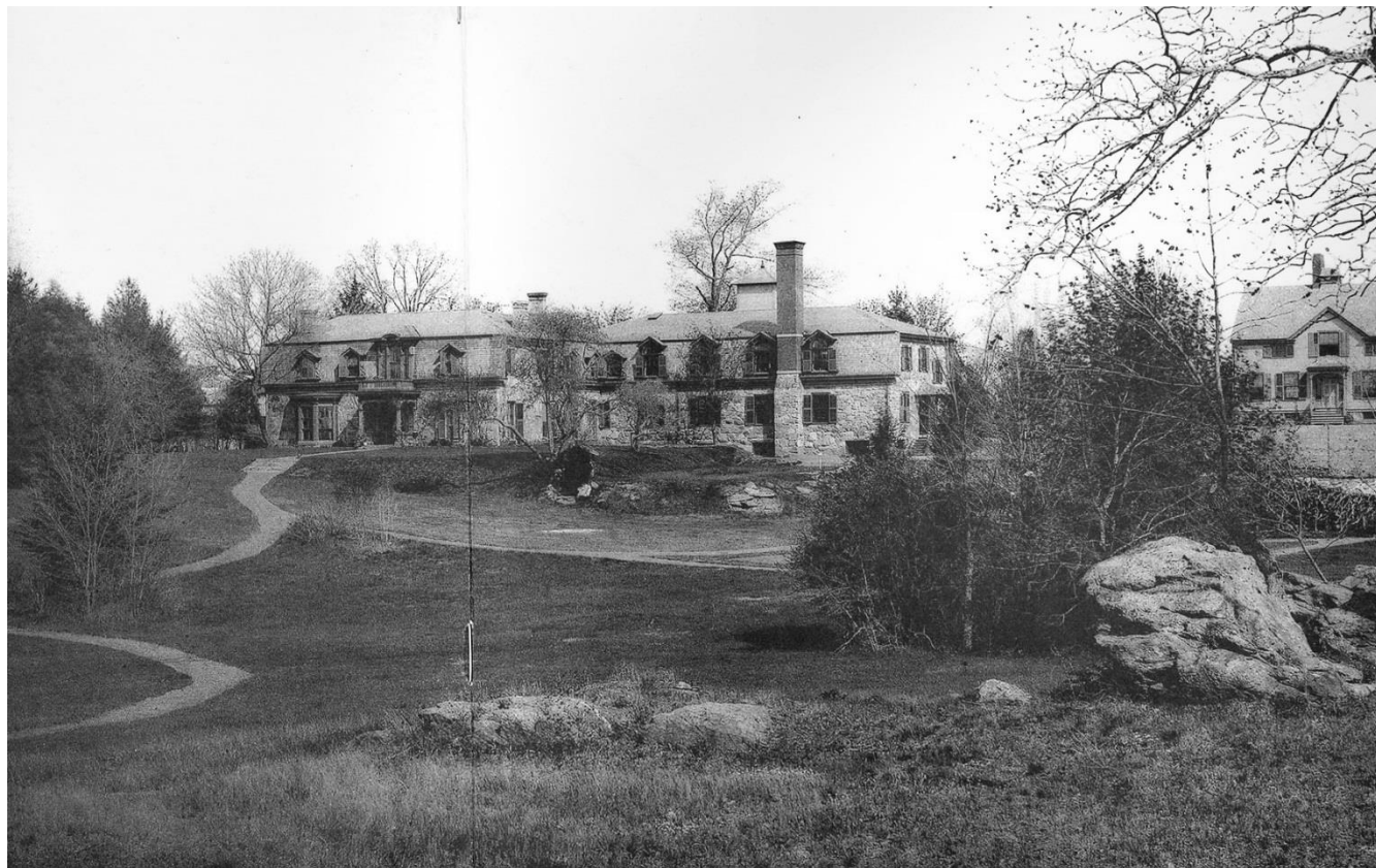
Figure 5 The earliest known photograph (c. 1890) of the State Home and School for Dependent and Neglected Children property showing the George W. Chapin House (left) after its conversion to a superintendent's residence and the completion of a wing addition to house a dining room and multi-purpose space for children. Cottage C (1885), the first wood-frame cottage purpose-built for the State Home and School, is seen to the right. This image also displays pathways and road systems which partially survive today. The boulder in the foreground is extant and provides a placemaker for the property.
