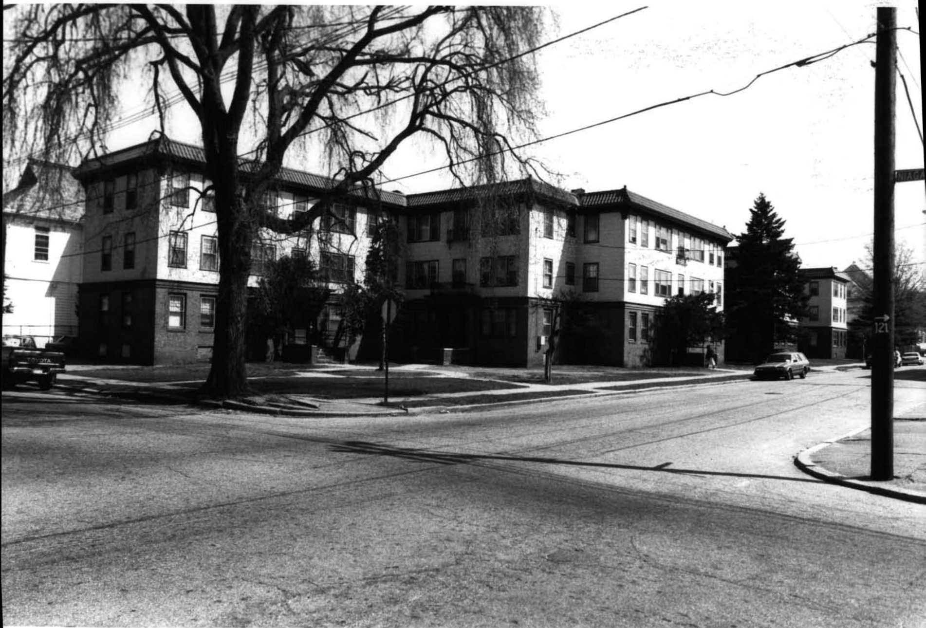
Ontario Apartments Providence City, Prov., R. I. Photo # 6 of 9
