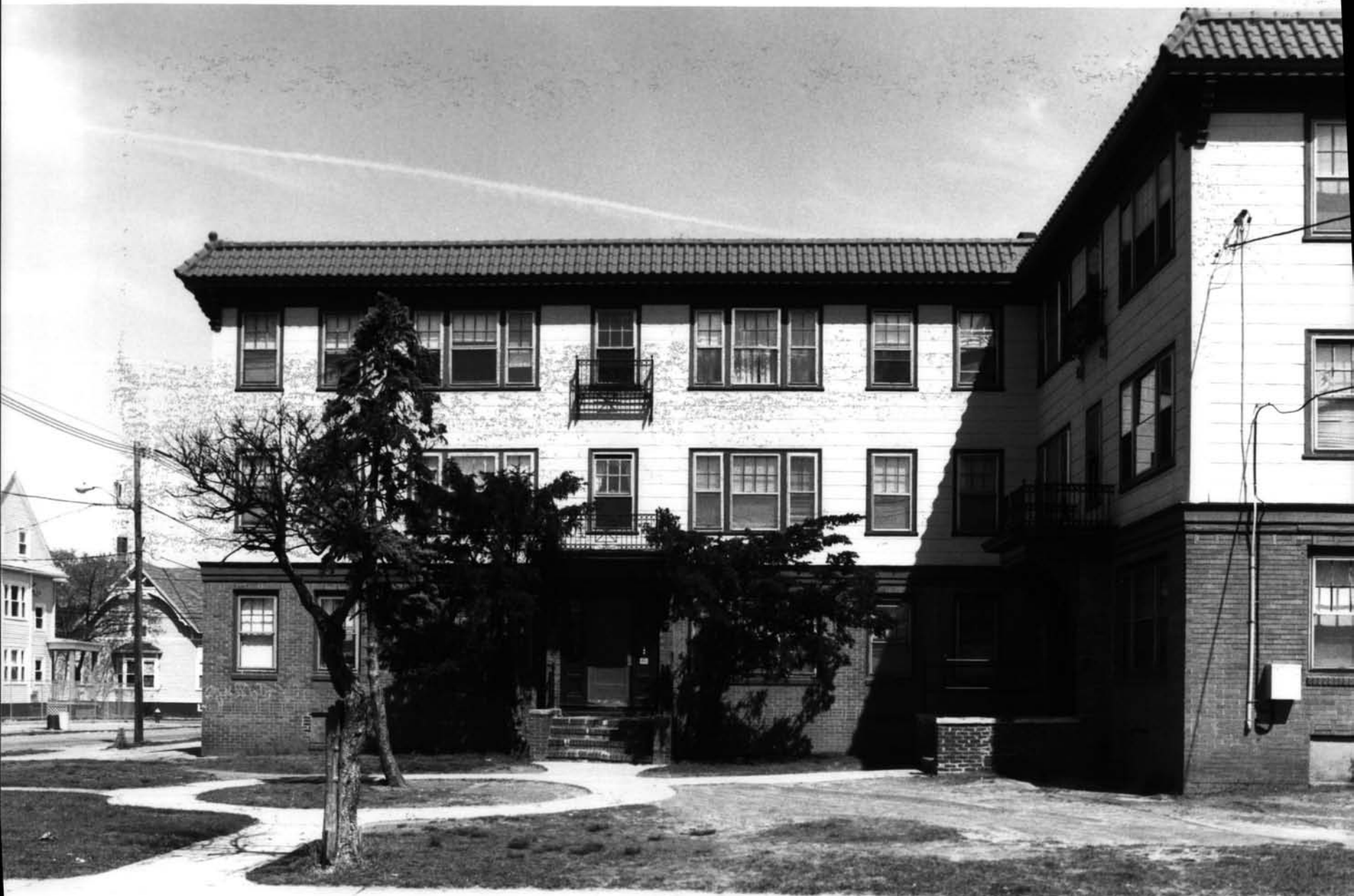
Ontario Apartments Providence City, Prov., R.I. Photo # 7 of 9
