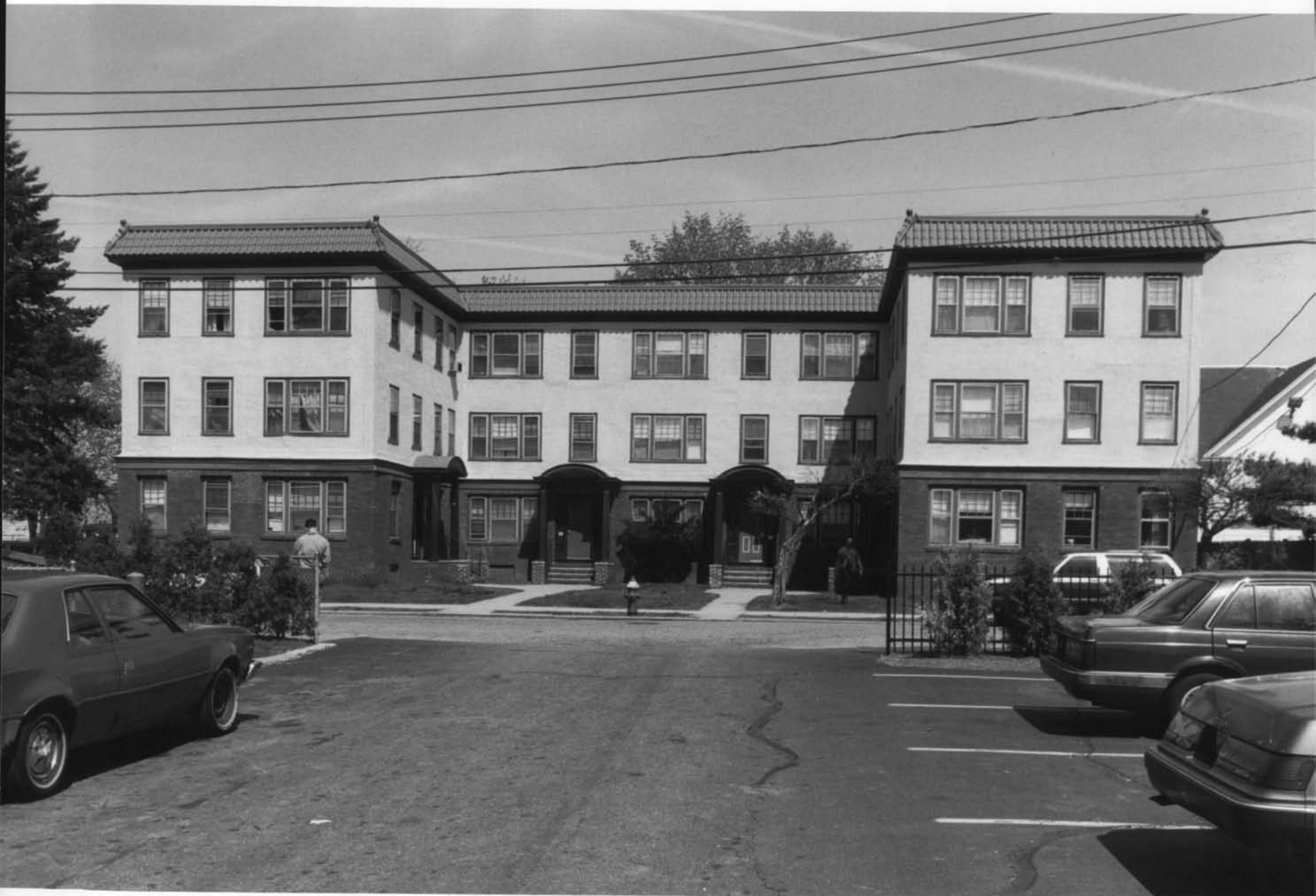
Ontario Apartments Providence City, Prov., R.I. Photo # 1 of 9
