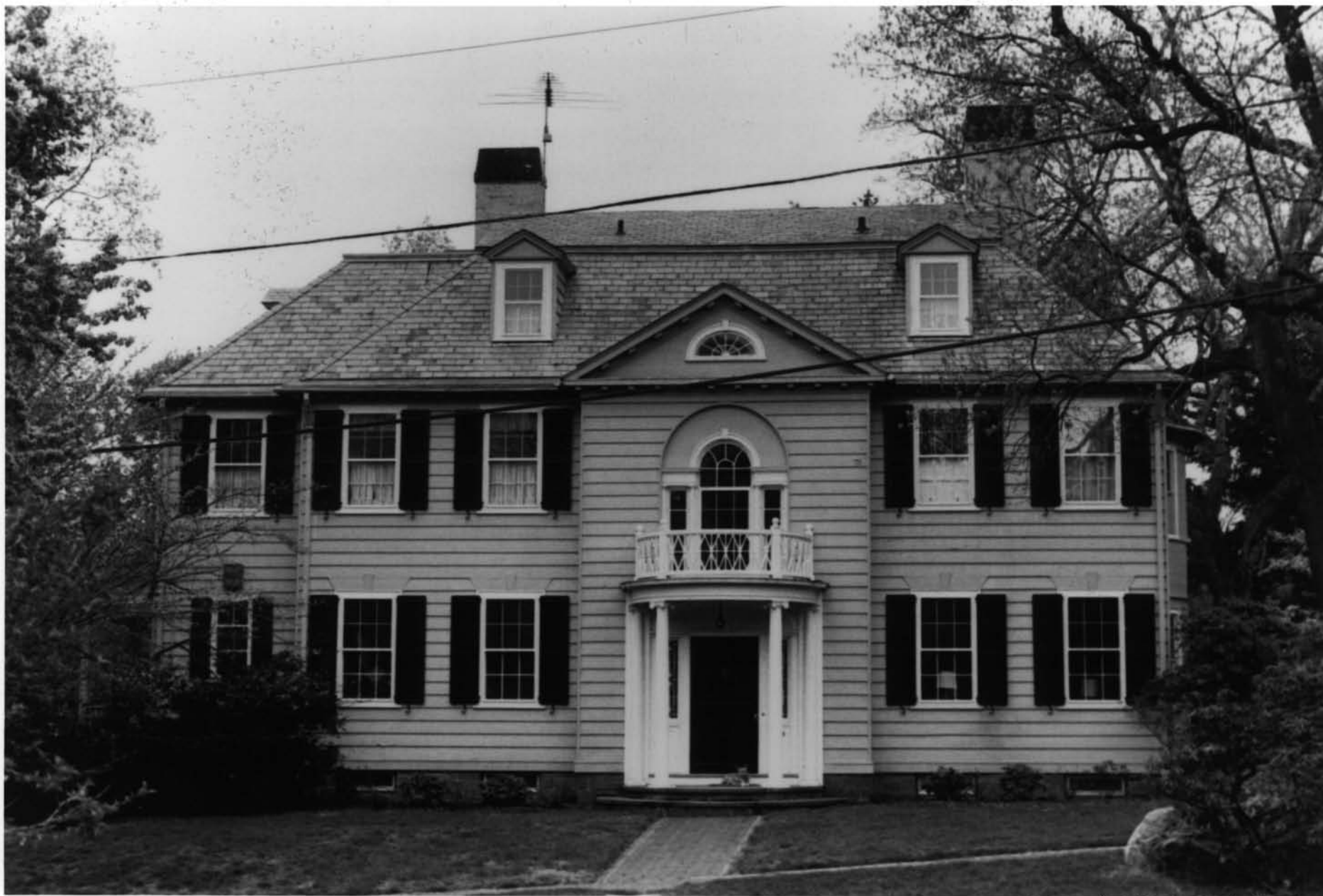
Freeman Plat Historic District Providence County, Rhode Island Photo # 4 of 7
