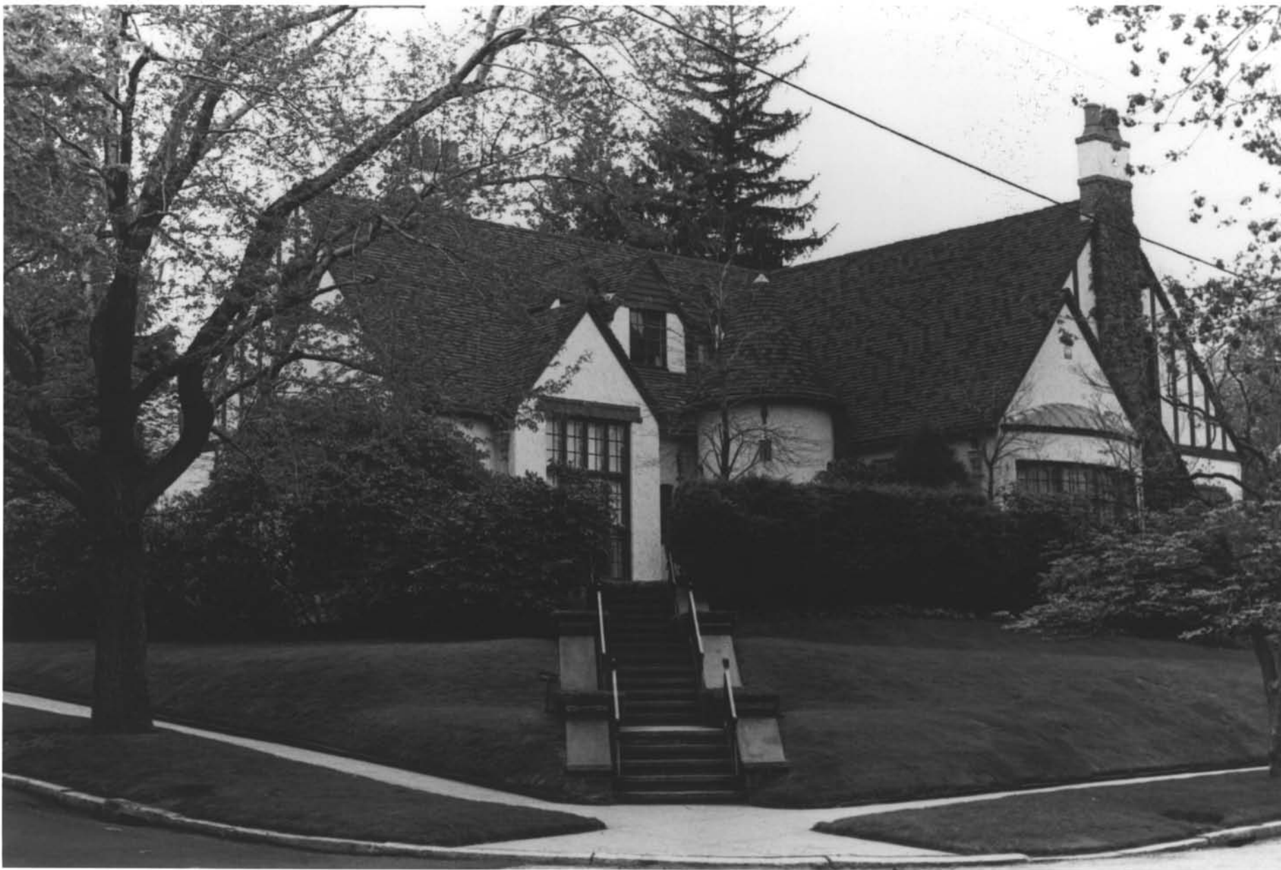
Freeman Plat Historic District Providence County, Rhode Island Photo # 6 of 7
