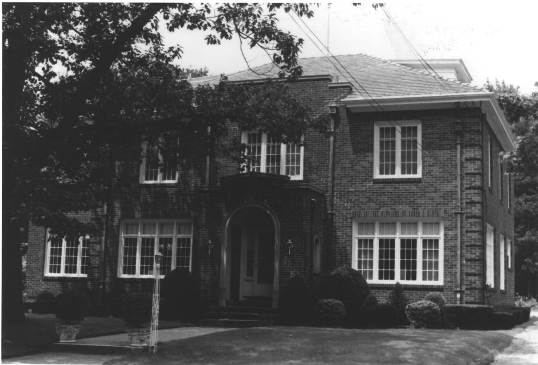
Freeman Plat Historic District Providence County, Rhode Island Photo #7 of 8
