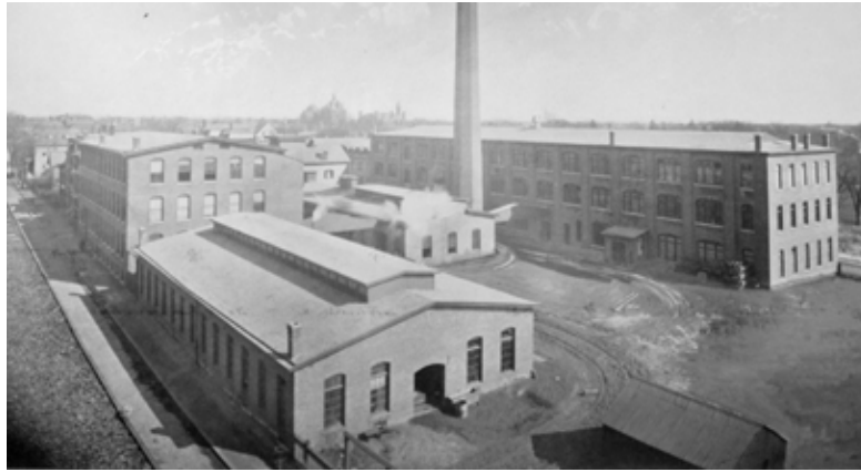
Figure 3 Plant of the Mechanical Fabric Company Halftone published in Board of Trade Journal (1894) showing Building 3 as original 3-story building, Building 4 as a 1-story building, and the Boiler House (Building 2) with original clerestory monitor.
