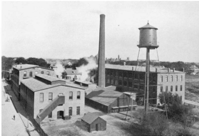
Figure 4 Plant of the Mechanical Fabric Company Halftone published in Board of Trade Journal (1897) showing expansion of Building 4 to two stories and the first iteration of Building 5 as a steel-clad, single-story storehouse Note gable-on-hip roof of Building 3 at right.
