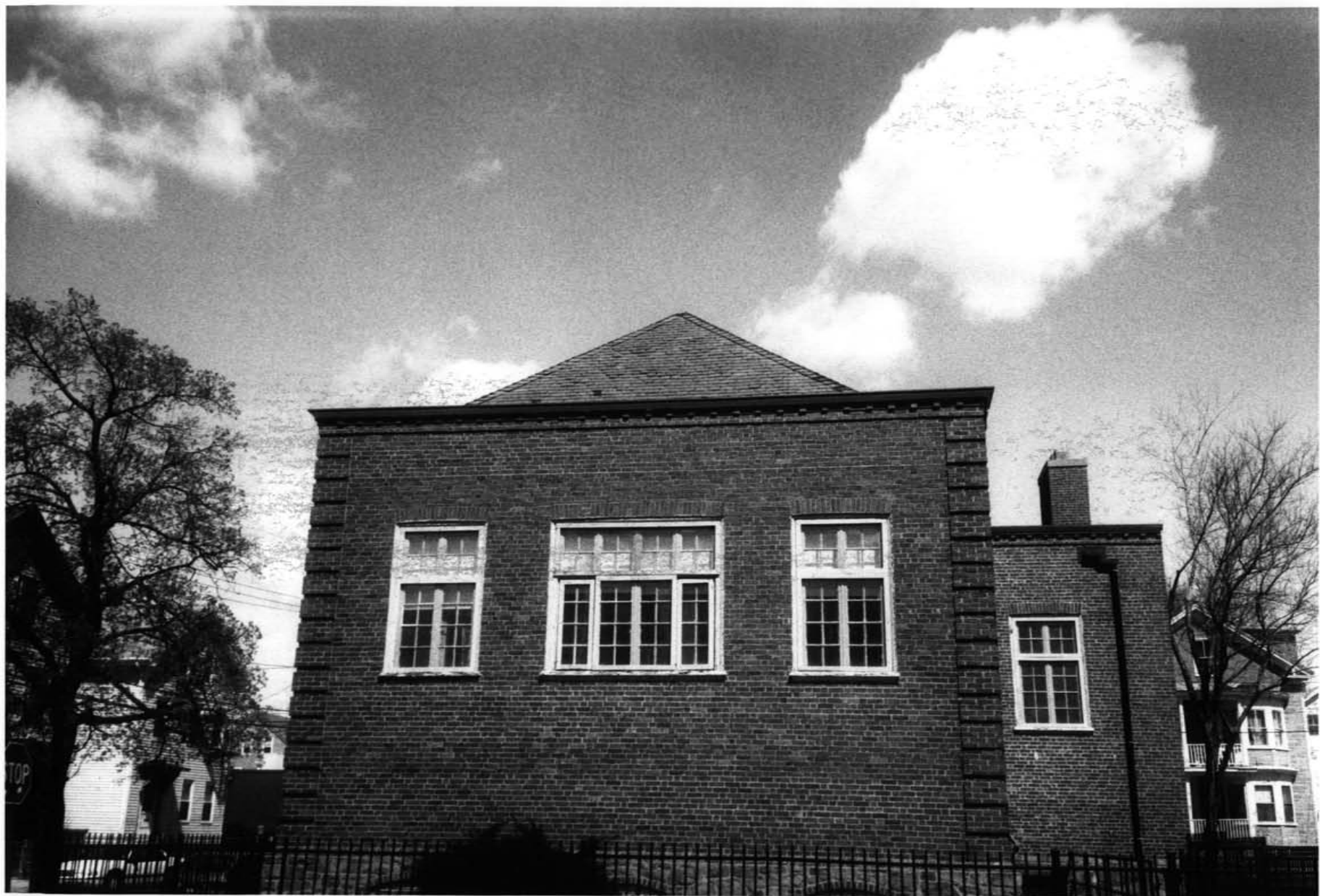
Smith Hill Branch Library Providence City, Prov., R.I. Photo # 2 of 4
