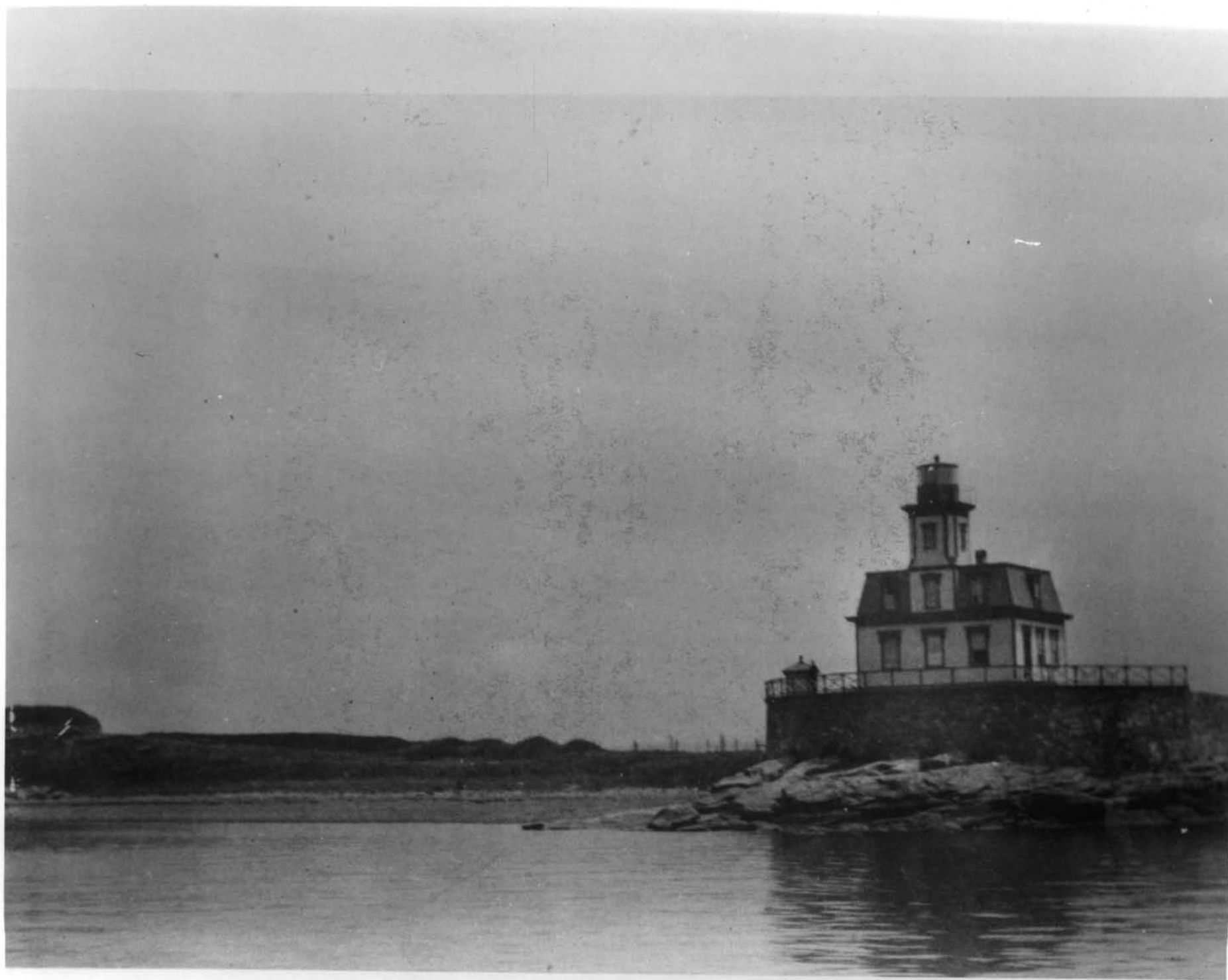
Fort Hamilton H.D., Newport County, R.I. Photo # 8 of 18
