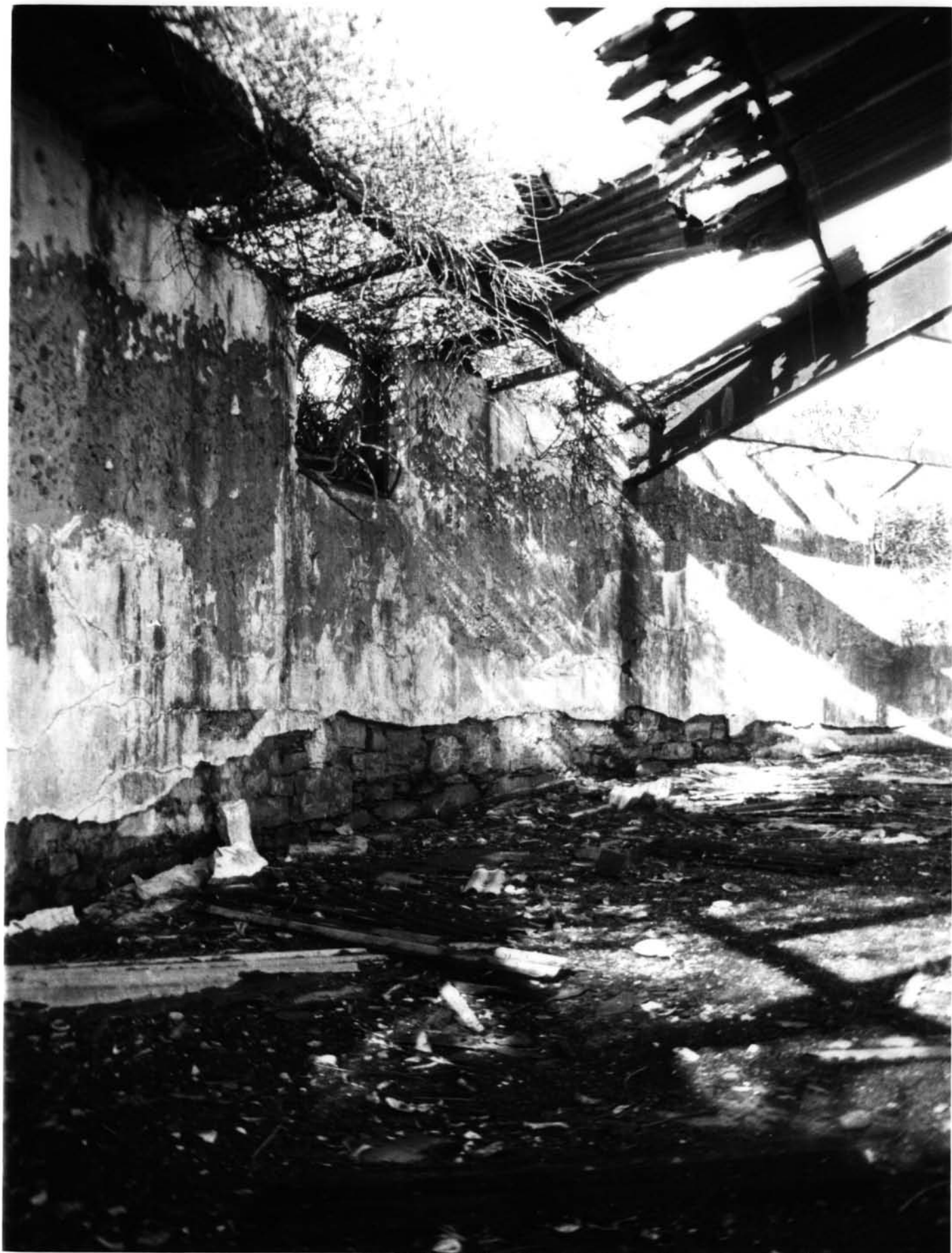
Fort Hamilton H. P., Newport County, R. I. Photo # 12 of 18
