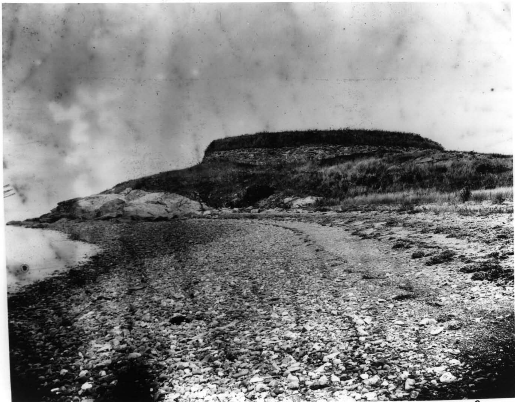
Fort Hamilton H.D., Newport County, R.I. Photo # 9 of 18
