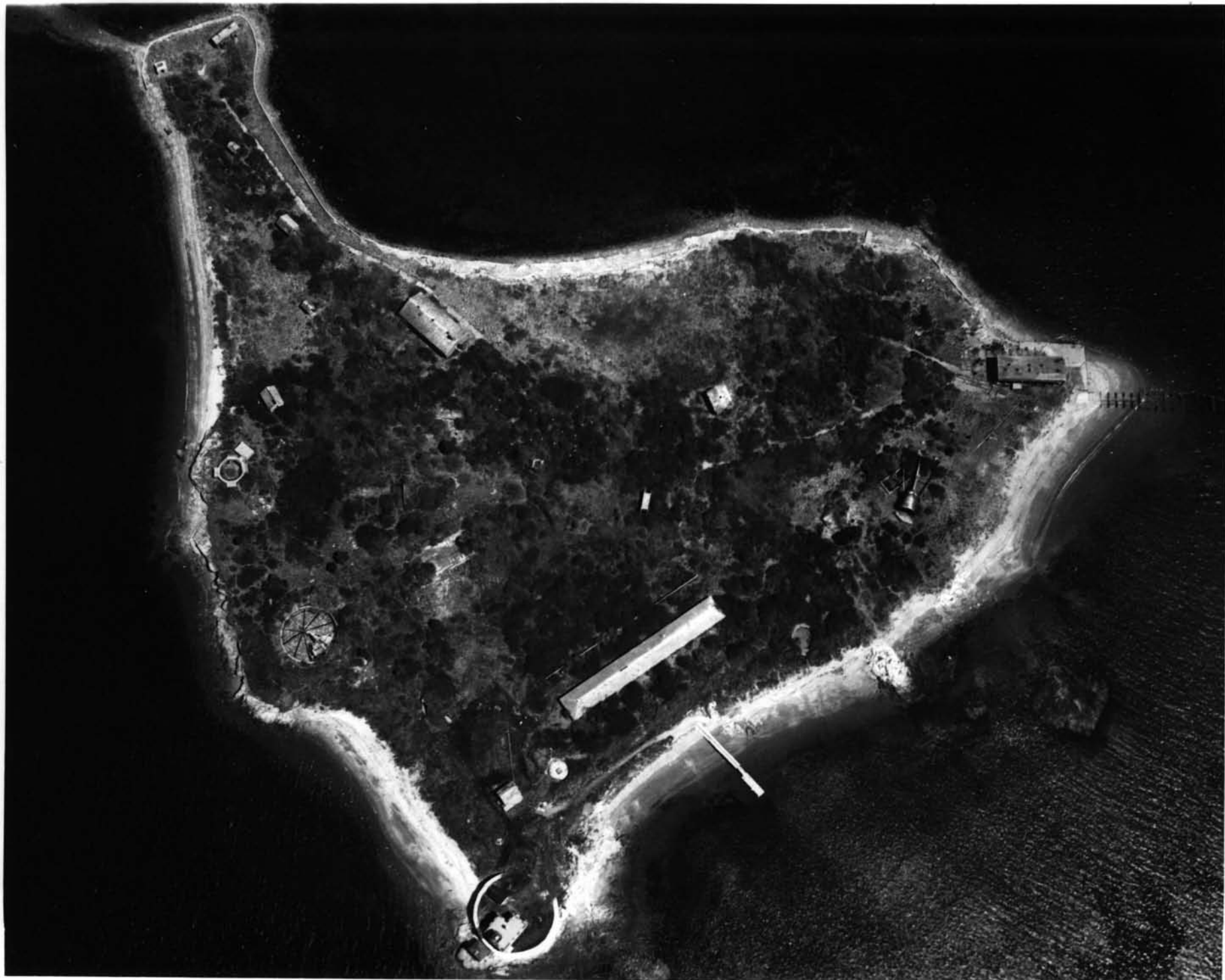
Fort Hamilton H.D., Newport County, R.I. Photo #5 of 18
