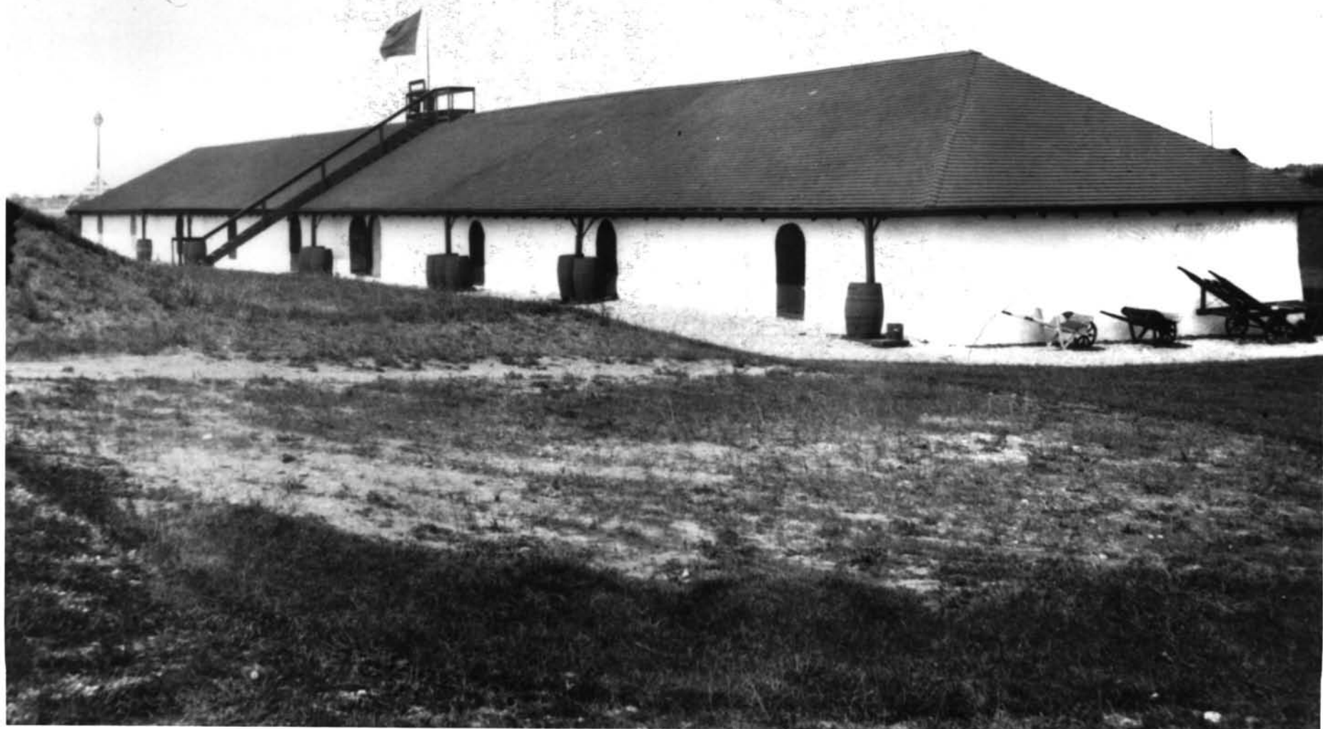
Fort Hamilton H. D., Newport County, R. I. Photo # 15 of 18
