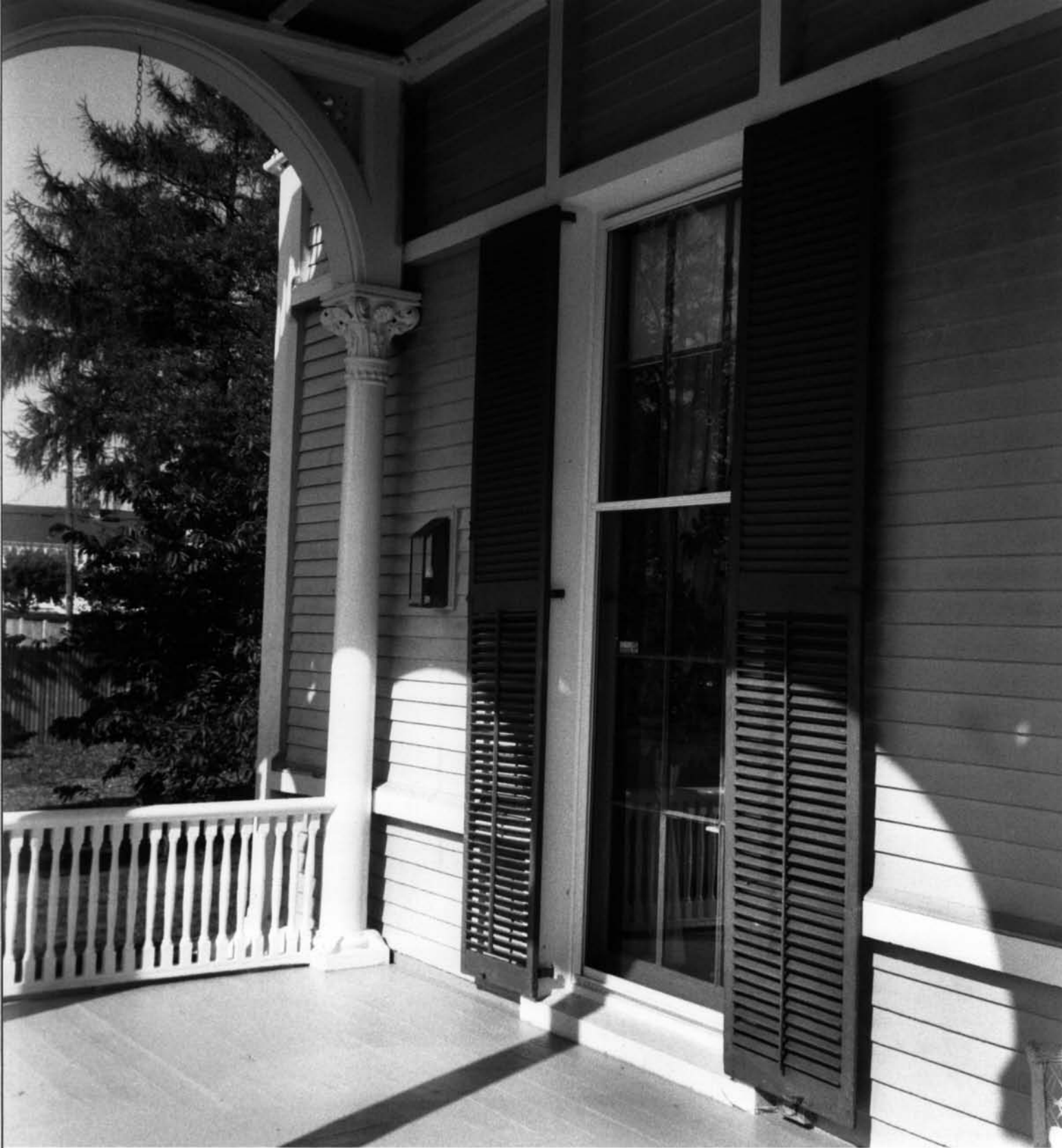
Hamilton Hoppin House Newport County, Middletown, N.H. Photo #3 of 10
