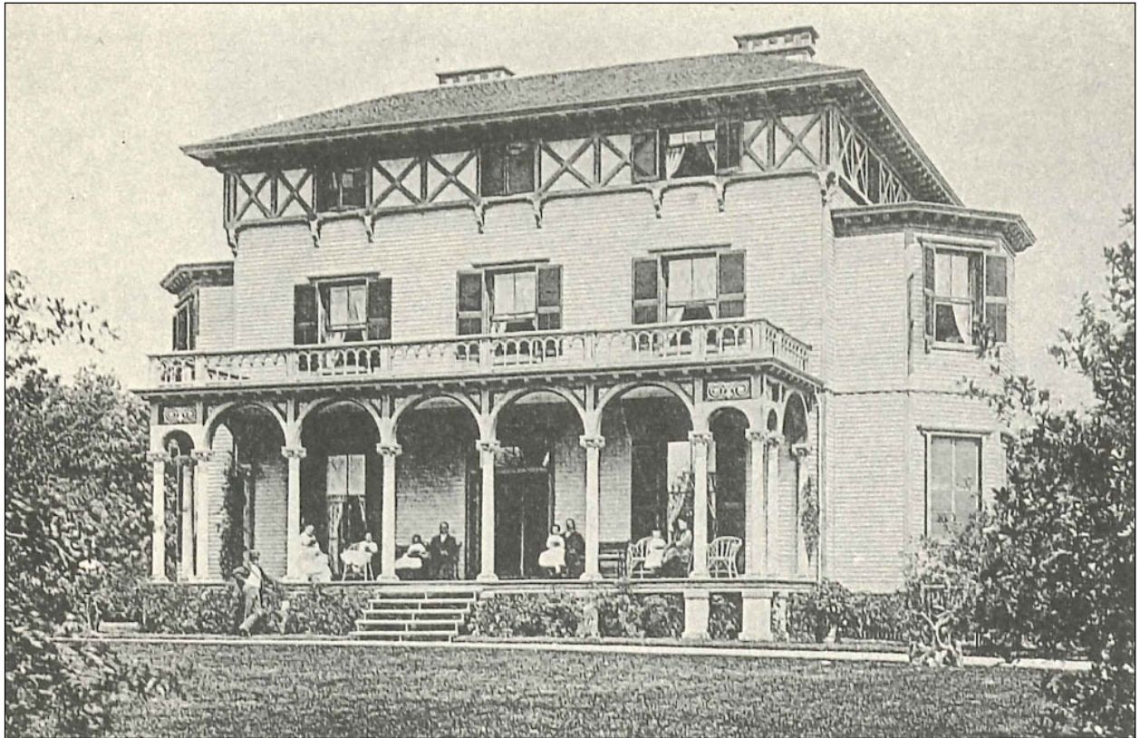
Figure 2. Photograph of Van Rensselaer House taken between 1880 and 1900, showing the original configuration of façade openings, porch design, and the two-story bays on the east and west elevations (source: Clarence Stanhope in Downing and Scully 1967).
