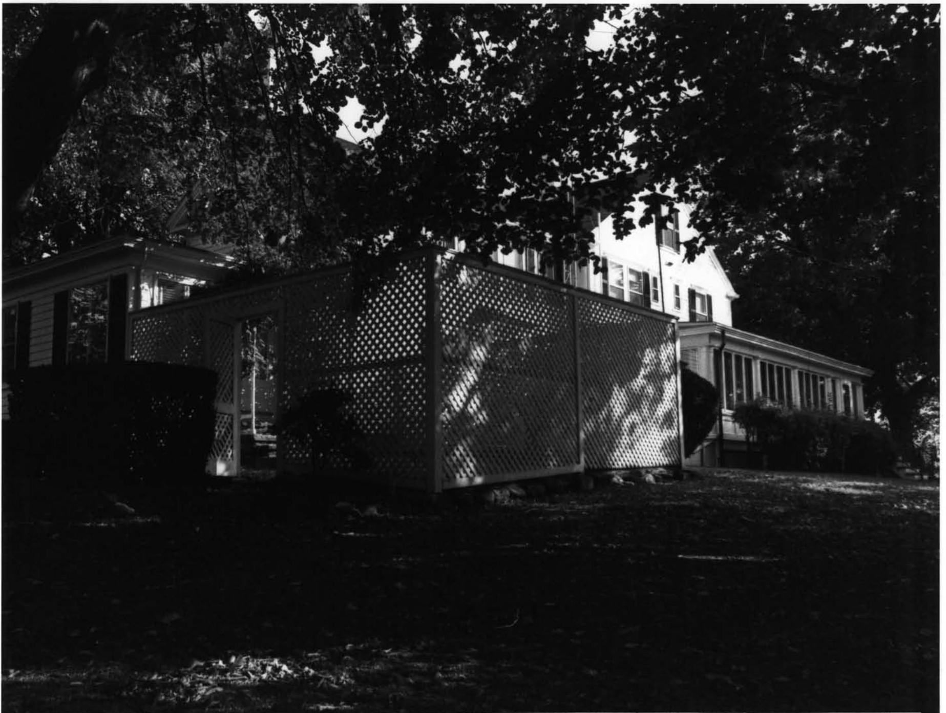
Taylor-Chase-Smythe House: View from northwest, showing 20th century laundry addition and drying yard in foreground.
