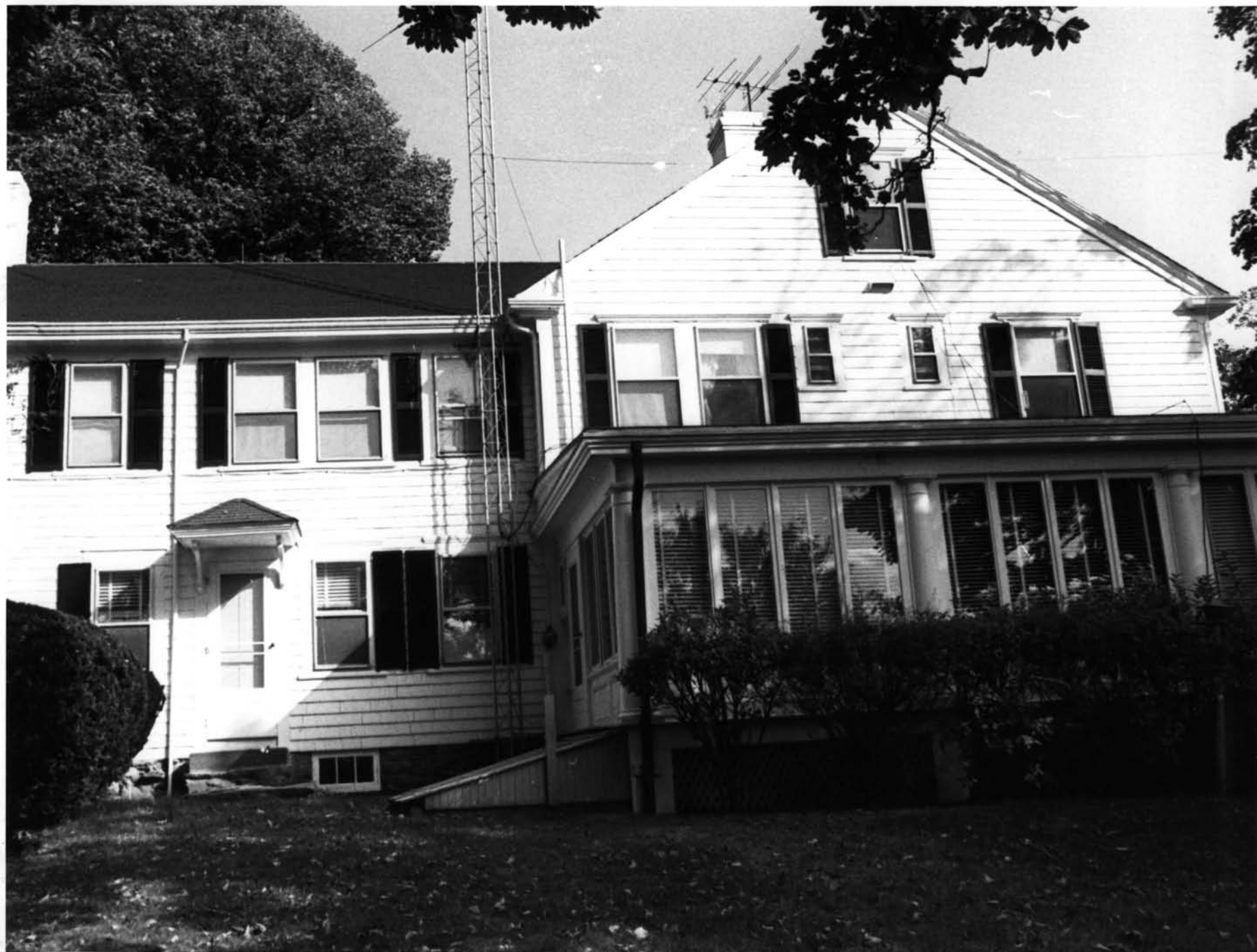
Taylor-Chase-Smythe House: West facade, showing gable-end of 18th century house with 20th century porch and 19th century ell.
