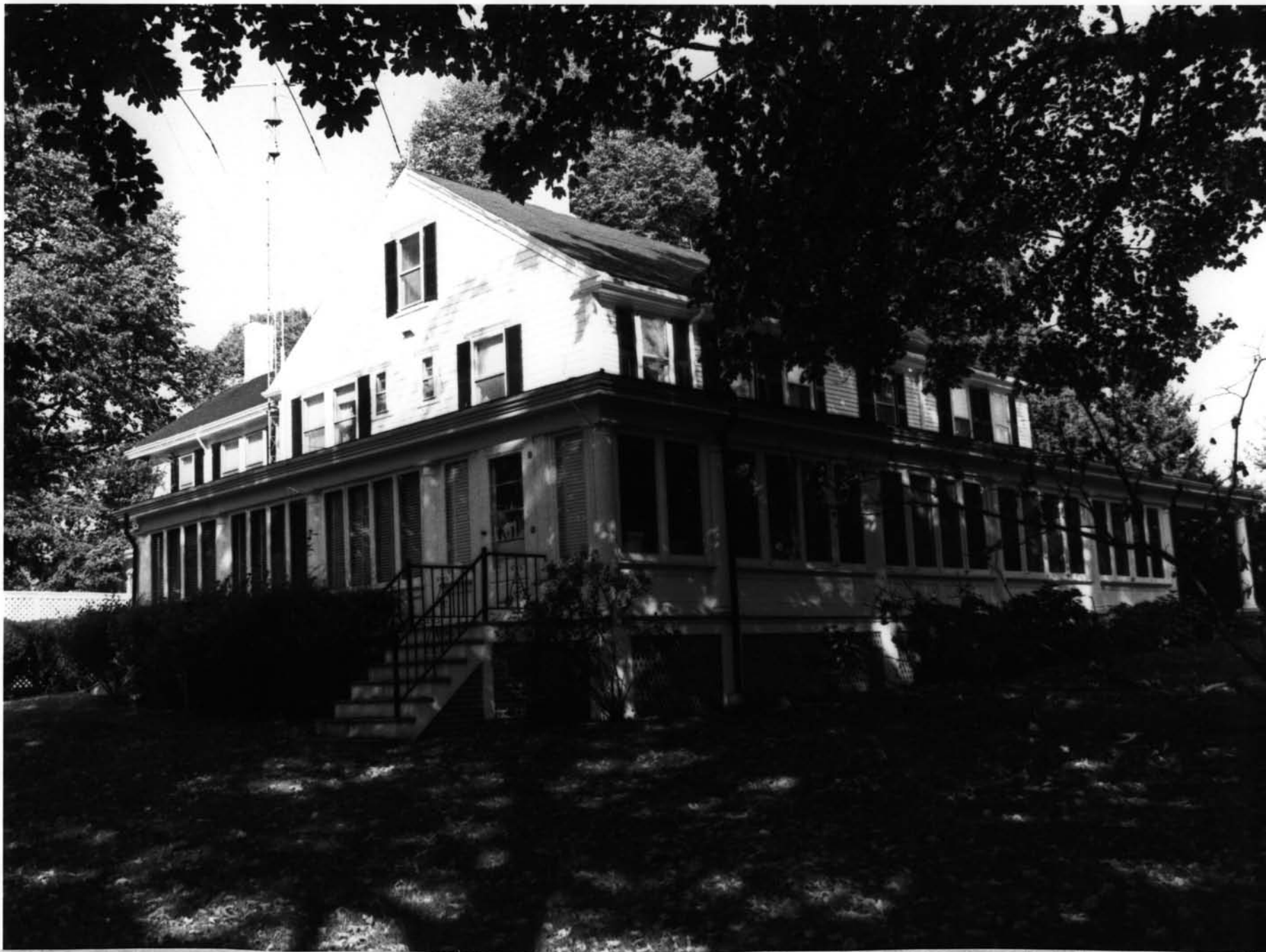
Taylor-Chase-Smythe House: South and west facades, showing original mass of 18th century house surrounded by glassed-in porch added in 20th century. Porte-cochere visible at far right.
