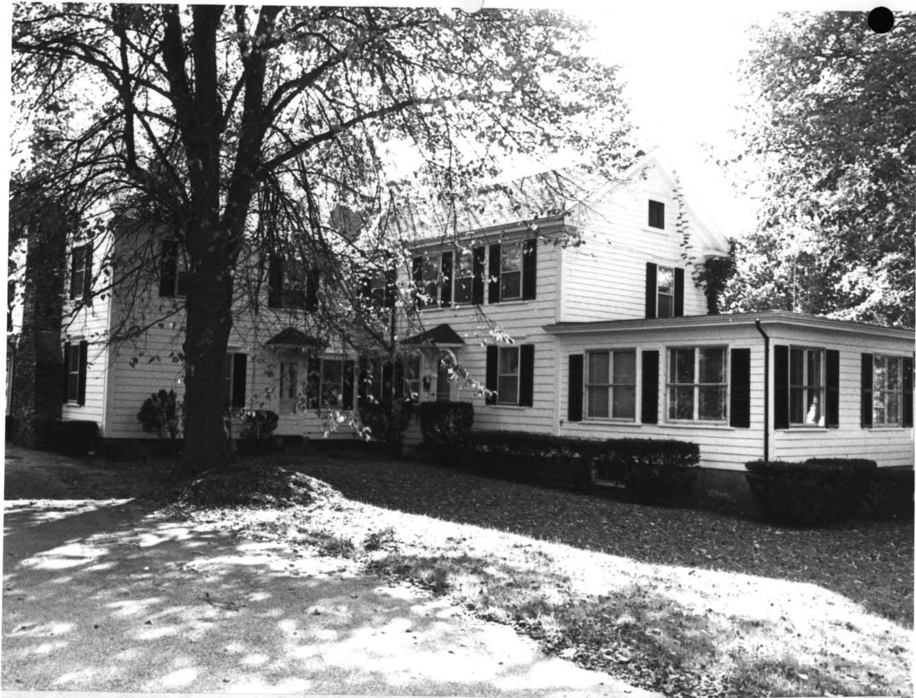
Taylor-Chase-Smythe House: North facade, showing, from left: original 18th century house, 19th century gabled ell, 20th century laundry addition.
