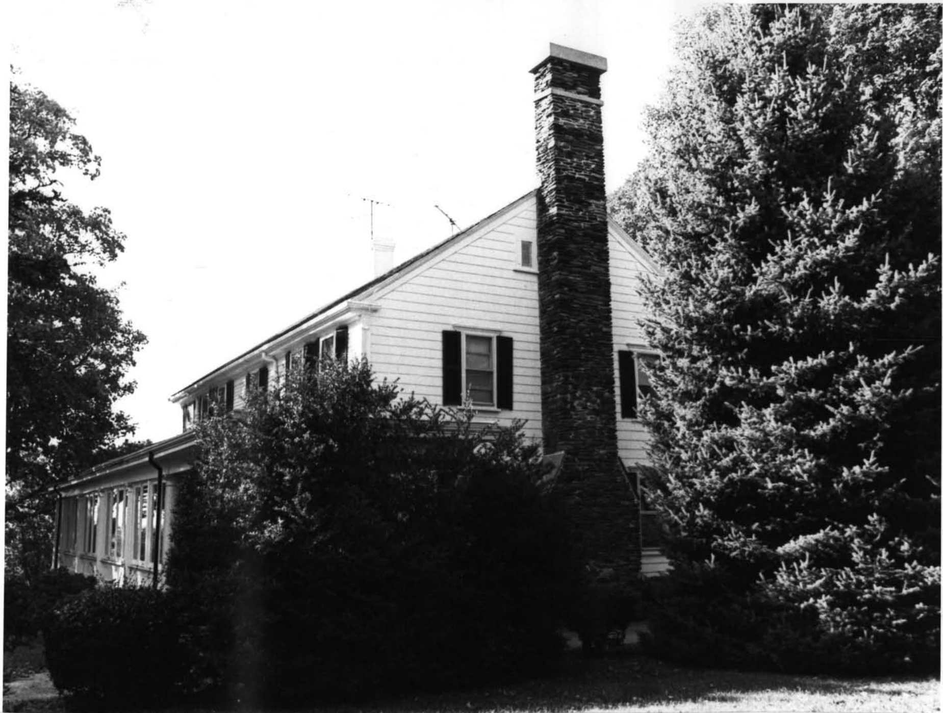
Taylor-Chase-Smythe House: East facade showing end chimney added in 1930s. Porte-cochere is behind shrubbery.
