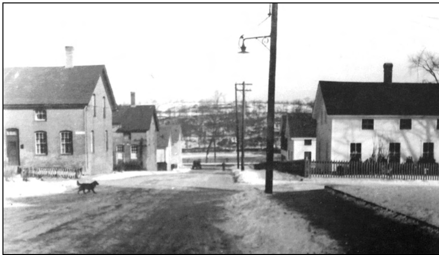
Figure 10 View down Spring Street to River near intersection of Spring and Park Way (1939) Roger Gladu collection
