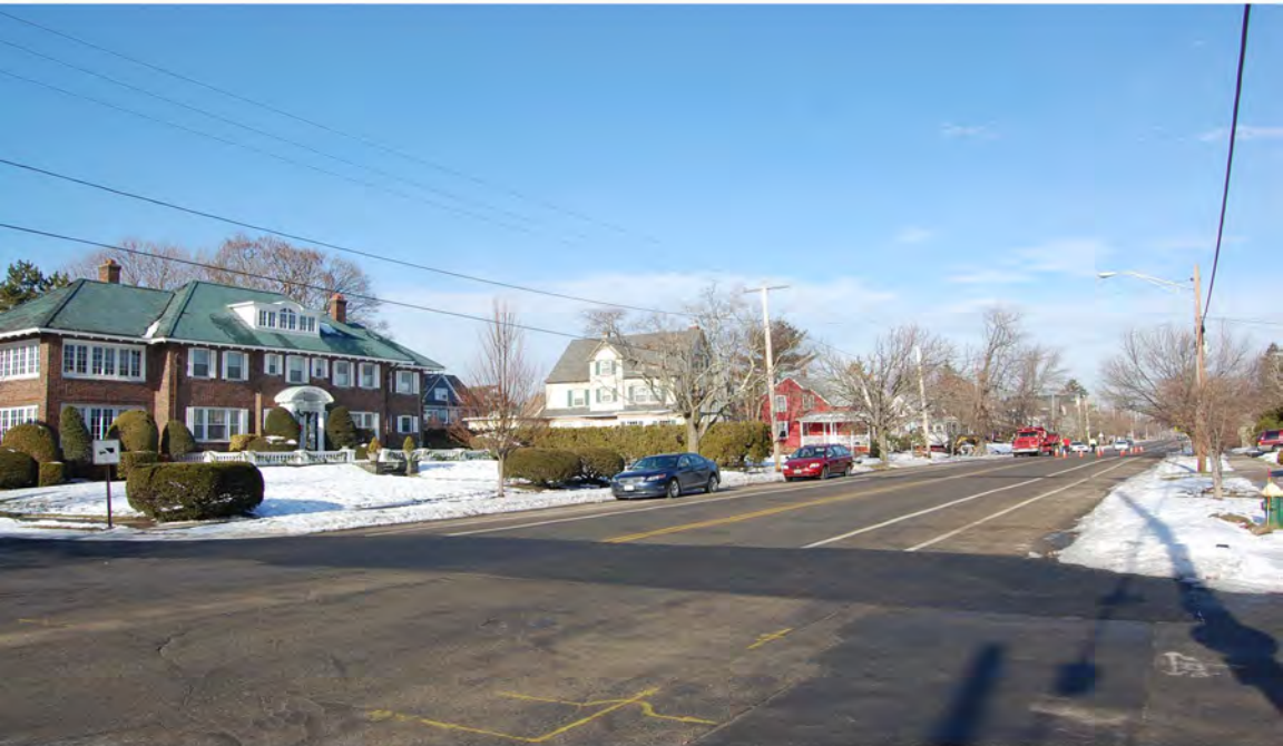
Edgewood Historic District - Anstis Greene Estate Plats Providence Co., RI Photo 4 of 13
