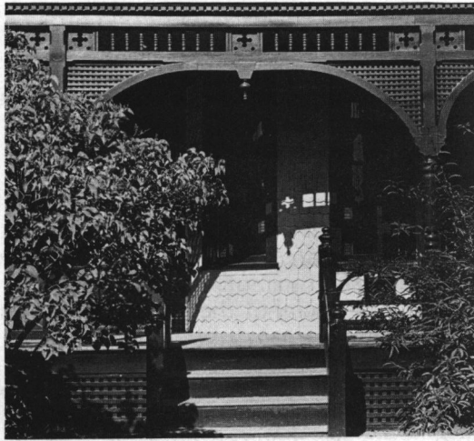
Fig. 53: Detail, Alphonse Gaulin House porch (c. 1885), 311 Elm Street.
