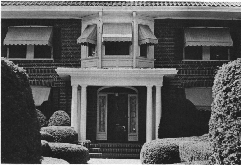
Fig. 74: The Joel Bense House entrance (c. 1917), 103 Glen Road .
