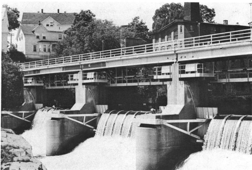
Fig. 85: Woonsocket Falls flood control barrier.
