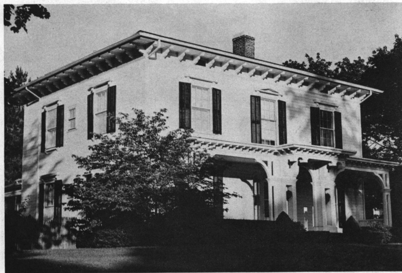
Fig. 24: The Lyman Cook House (1847), 246 Harris Avenue.
