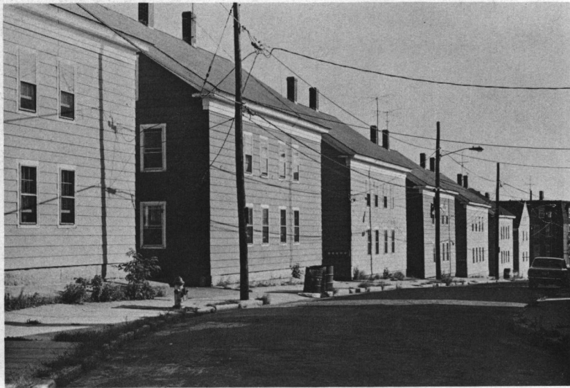
Fig. 22: Globe Mill housing (c. 1865), Lincoln Street.
