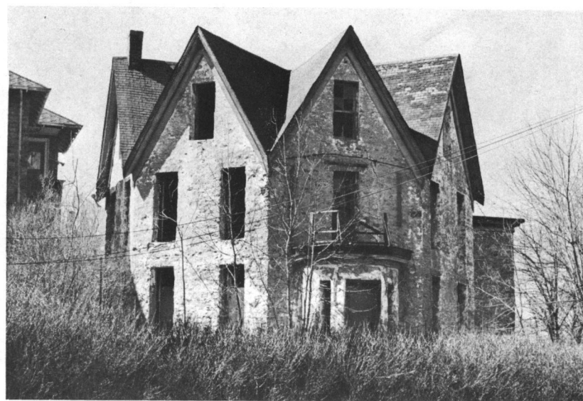
Fig. 27: The Sabin Pond House (c. 1849), 315 Grove Street.
