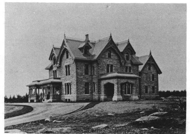
Fig. 50: Alfred A. Reed Estate (between 1870 and 1875); 4157 Post Road; photograph, 1870s.
