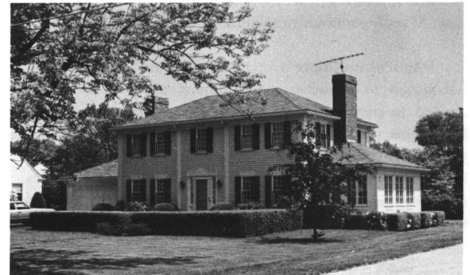
Fig. 80: John Olson House (1940); 296 Spring Green Road.
