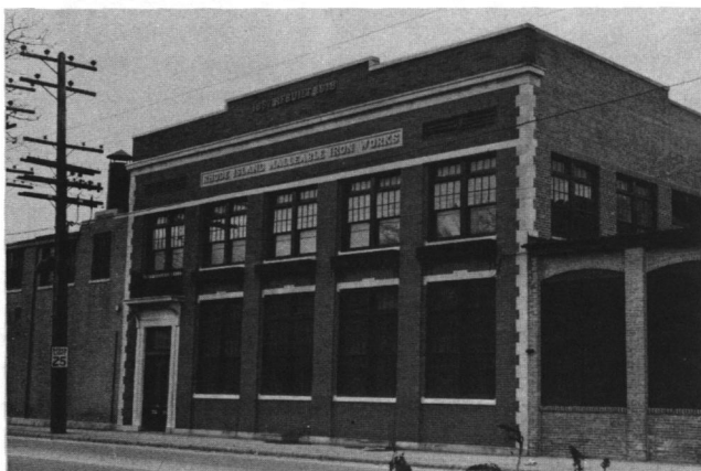
Fig. 66: Rhode Island Malleable Iron Works, now United Wire and Supply (1918); 697 Jefferson Boulevard.
