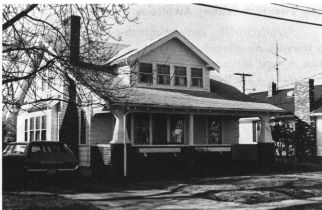
Fig. 74: Noel B. Chartier House (1930); 381 Norwood Avenue.
