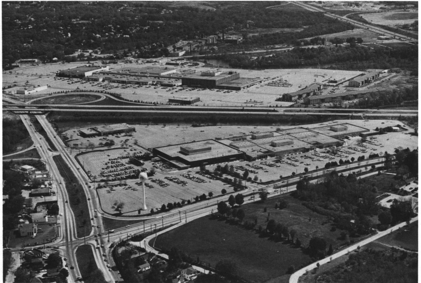
Fig. 86: Aerial view showing Midland Mall (1965-1967) in the foreground and Warwick Mall (1968-1970) in the background; photograph, 1976.
