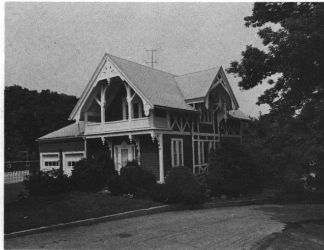
Fig. 47: Amasa Sprague Estate Carriage House (ca. 1870); 118 Valentine Circle.
