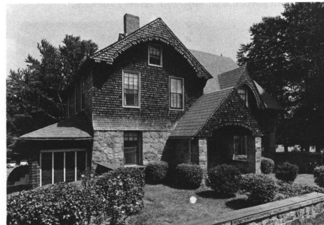
Fig. 62: Aldrich Estate Gardener's Cottage (1899); 946 Warwick Neck Avenue.
