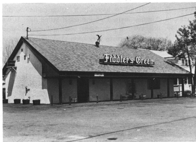
Fig. 12: Quaker Meetinghouse, now Fiddler's Green Restaurant (ca. 1716 with later alterations); 1705 West Shore Road.
