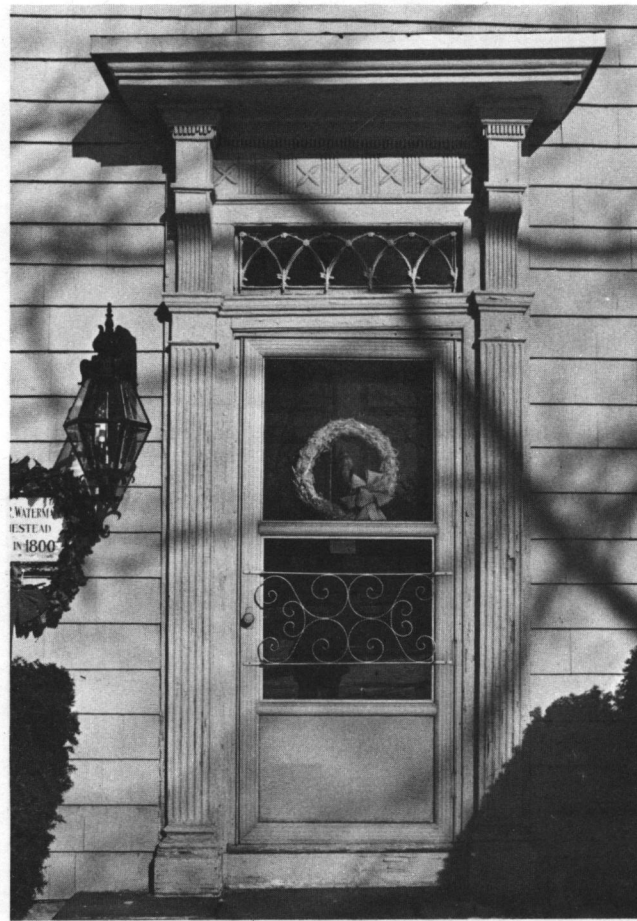
Fig. 22: Flat-top doorway with transom and consoles from the John R. Waterman House (ca. 1800); 100 Old Homestead Road.
