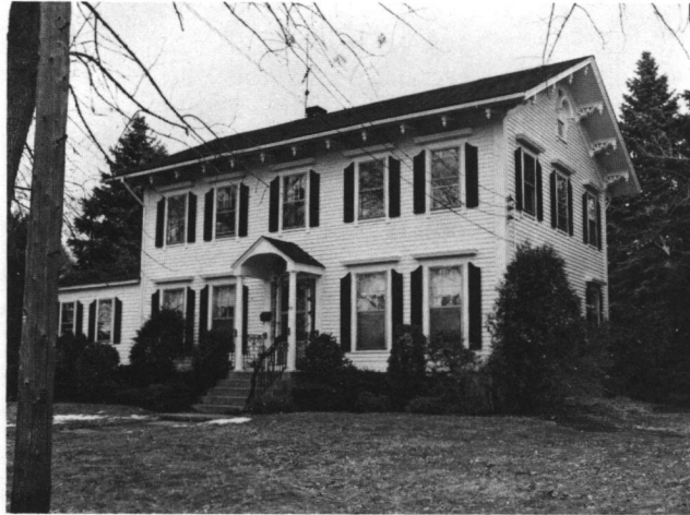
Fig. 57: Reverend Jonathan Brayton House (ca. 1860); 42 Bridal Avenue. A fine example of a traditional 5-bay house updated with Italianate brackets and window hoods. The front portico is an early 20th-century addition.
