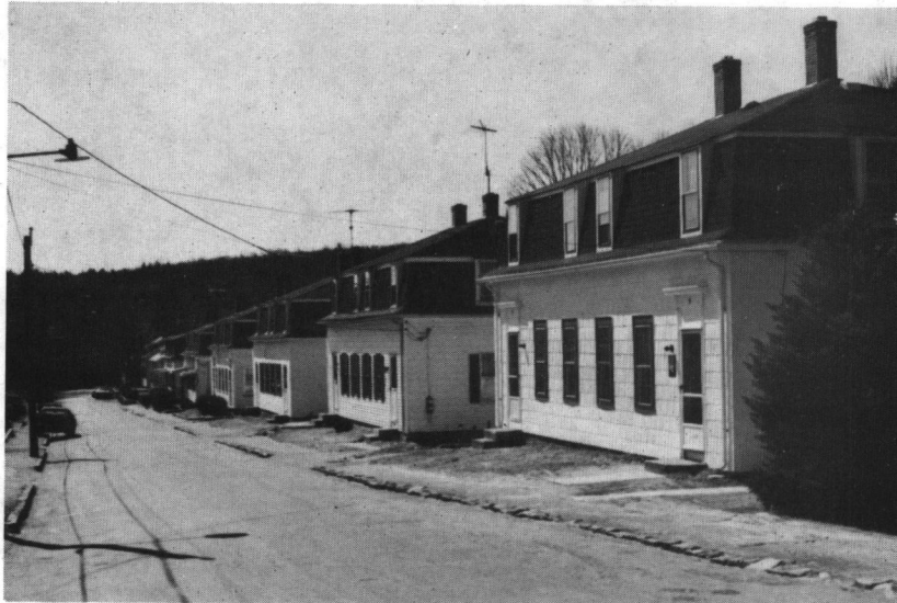
Mill House (1872): Mill Street, Hope Historic District. (Map #2K)
