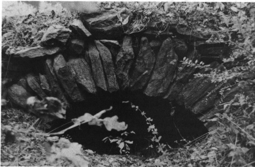
Stone Arch under Peeptoad Road at Site of Harrisdale Mill. (Map #103)
