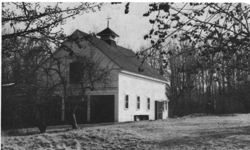
Barn at Aldrich House: Rocky Hill Road. (Map #131)
