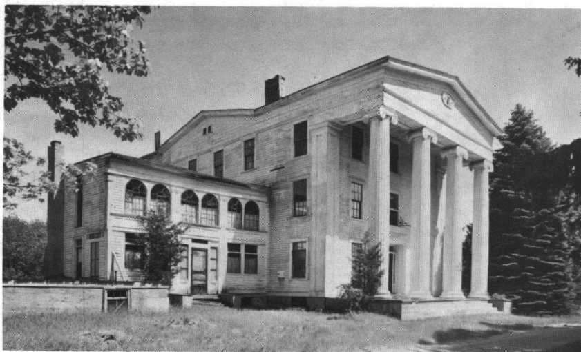
Former Smithville Seminary (1839): Institute Lane, North Scituate Village Historic District. (#3F)
