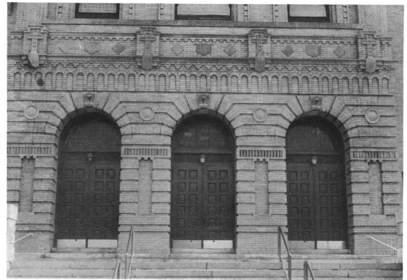
Fig. 48: Entrance, St. Charles Borromeo (1915)
