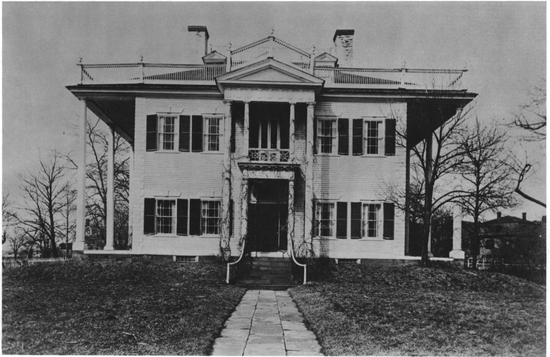
Fig. 5: Messer Mansion (c. 1800, demolished 1894), Cranston Street
