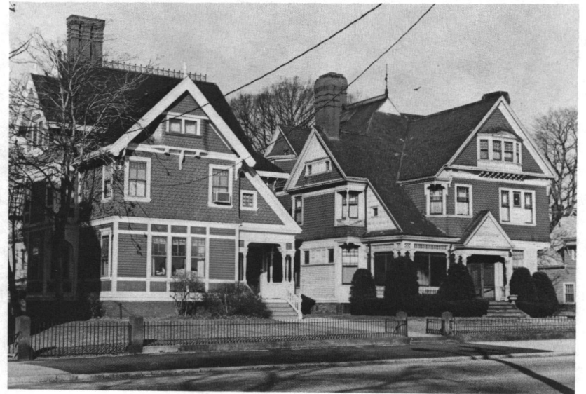
Fig. 36: E. I. Nickerson Houses (c. 1890), 77 and 81 Parade Street
