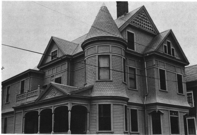
Fig. 35: Residence (c. 1891), 56 Bainbridge Avenue
