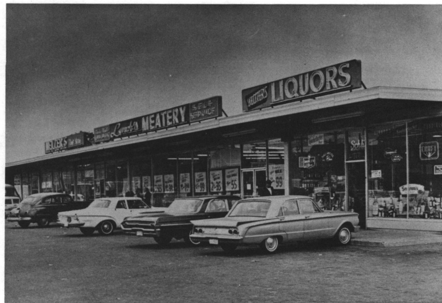
Figure 66: Willard Shopping Center (1956); Prairie Avenue; photograph, c. 1963.
