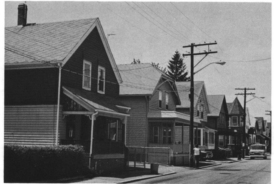
Figure 38: Powder House Plat Houses (c. 1888); Gladstone Street.
