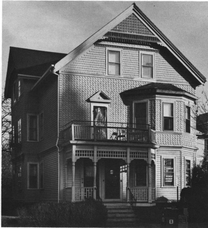
Figure 37: James H. Hagan House (1891); 728-730 Broad Street.
