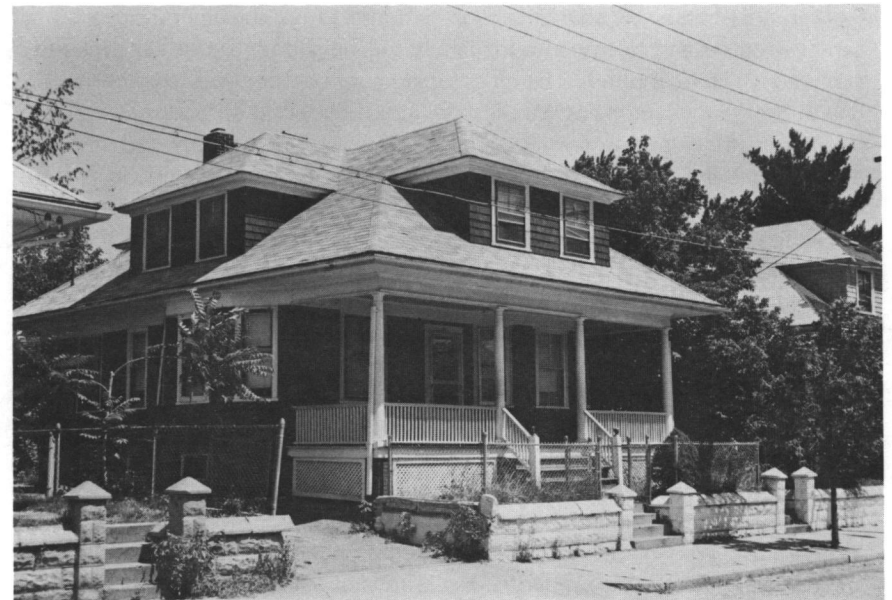
Figure 59: Thomas Carlisle House (c. 1912); 151 Briggs Street.
