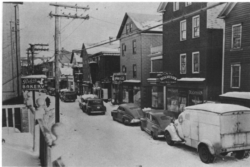
Figure 65: View of the Willard Avenue Retail Section (all buildings demolished in 1954); photograph, 1948.
