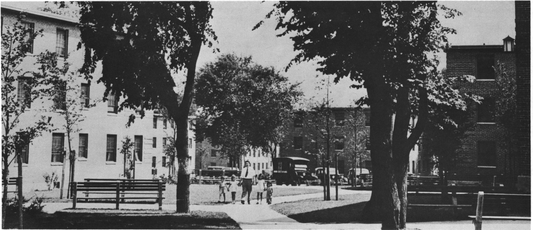
Figure 60: Roger Williams Housing Project (1943); Thurbers Avenue between Prairie Avenue and Rugby Street; photograph, c. 1950.
