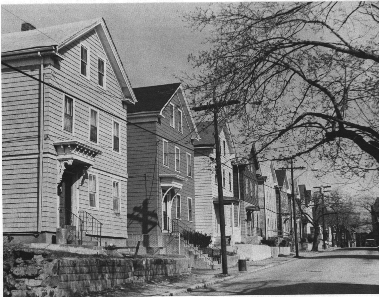
Fig. 39: Burnside Row (1866-1867); Zone Street.
