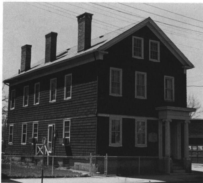
Fig. 31: Jonathan Tucker House (ca 1851); 206 Smith Street. Alterations in the late 19th century included shingling that covers the corner boards.
