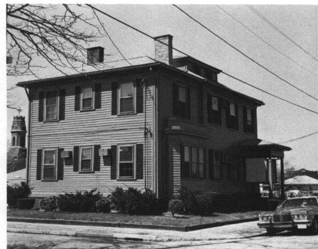
Fig. 30: House (ca 1830 et seq.); 60 Davis Street. Front elevation, showing addition at left.
