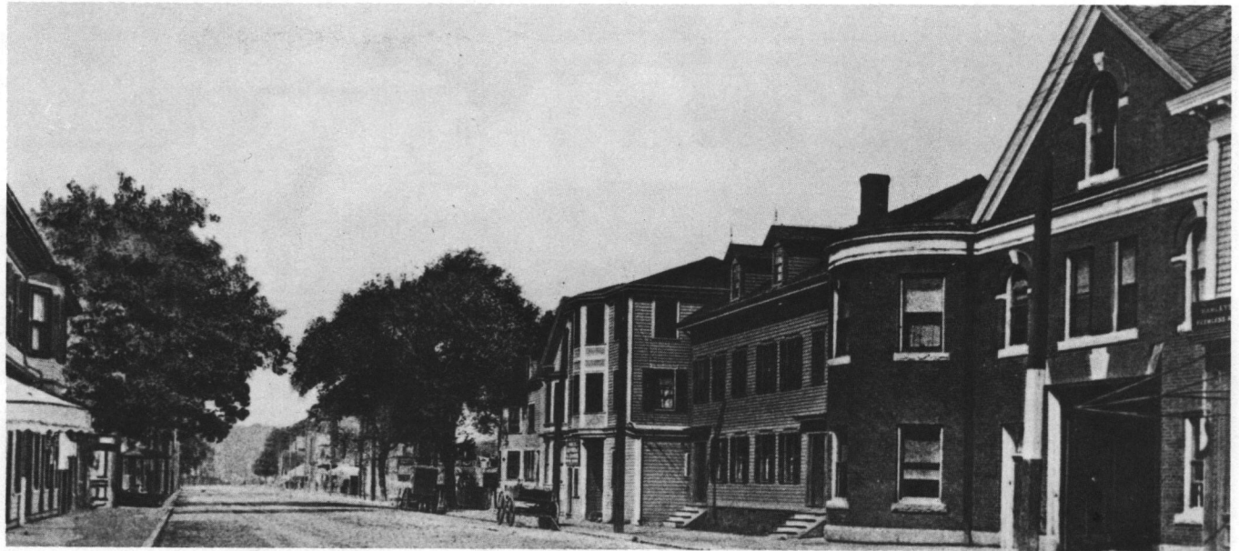
Fig. 48: View west on Douglas Avenue from the intersection of Chalkstone Avenue. The Douglas Avenue Fire Station is at the far right.
