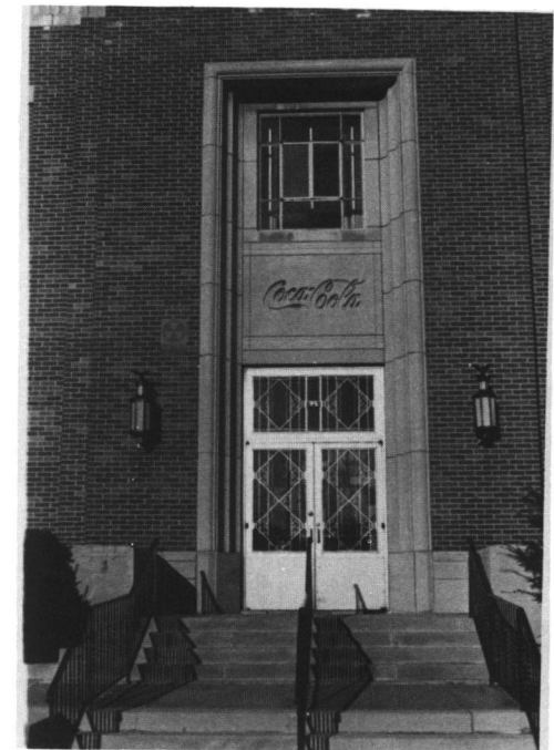
Fig. 61: Pleasant Valley Parkway; detail of Coca-Cola bottling plant.
