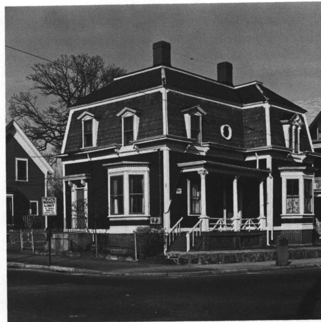
Fig. 26: Charles Dowler House (1872); 581 Smith Street. This mansard-roof dwelling is a typical 1870s form. Few houses of this type and quality remain in the city today in such a well-preserved state.
