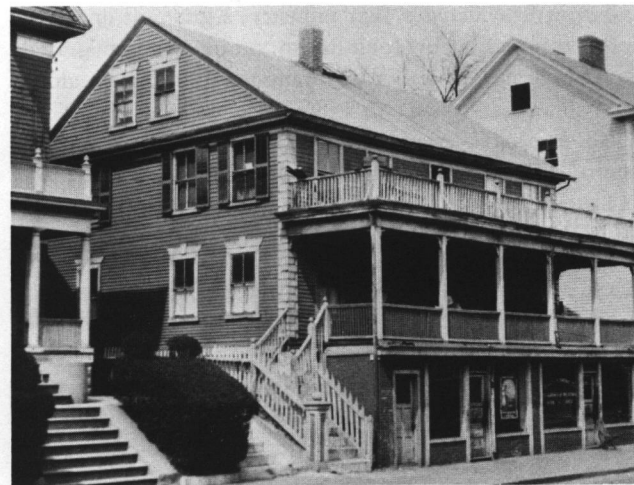
Fig. 9: Zachariah Allen House (ca 1770); 151 Orms Street; photograph, ca 1930; demolished. The porch and street-level storefronts are later 19th-century additions.
