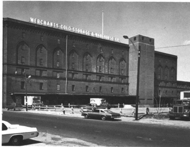
Fig. 14: Merchants Cold Storage Warehouse (1893 et seq.); 160 Kinsley Avenue.
