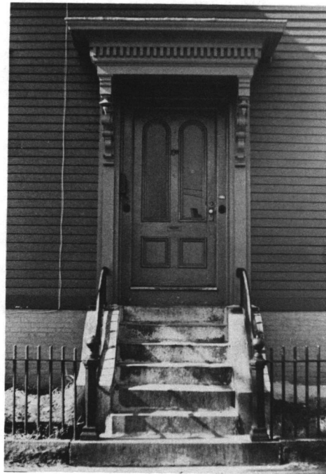
Fig. 60: Alma Street, detail of doorway.
