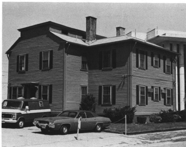
Fig. 29: House (ca 1830 et seq.); 60 Davis Street. The portion at left is part of the original monitor-on-hip-roof section.
